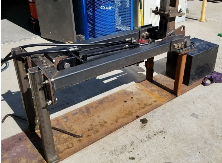
Figure 72. Truss attachment assembly in progress
