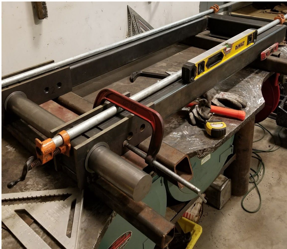
Figure 65. Shaft assembly leveled and tacked onto base frame assembly
