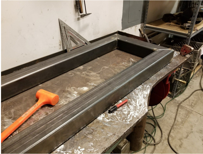
Figure 64. Frame assembly leveled and tack welded
