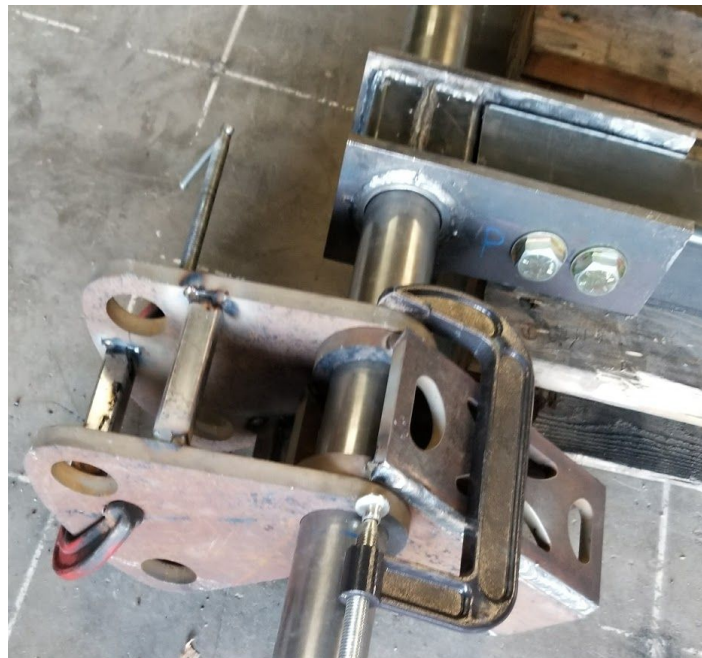
Figure 70. Truss attachment assembly in progress
