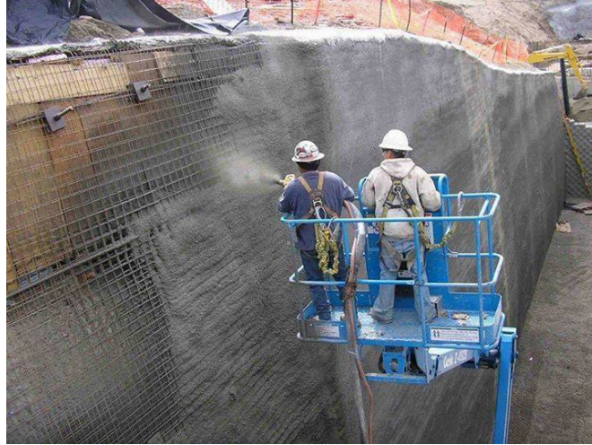
Figure 5 – Shotcrete Application on Commercial Foundation
