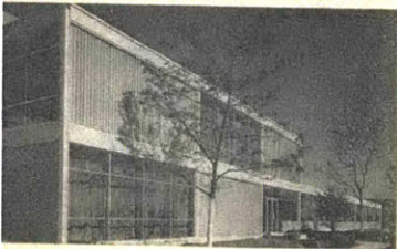
FACTORY of United Biscuit Co. at Melrose Park, Ill., has wide windows contrasting with ribbed metal panels framed in steel. It extends a quarter-mile back from this end.
