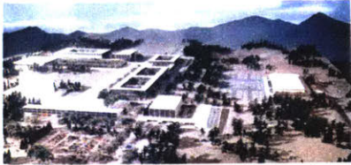
The Air Force Academy commission went to S.O.M. in 1954 when the Air Force selected it from a field of 147 competing firms to take full responsibility for master planning, design, and construction supervision. In addition to the academic area shown, accommodating 2,640 cadets, the 17,900-acre site near Colorado Springs will include a community to house 3,000 support personnel. S.O.M. has set up a 250-man field office in the area to supervise the forty general contractors who are doing the actual building.
