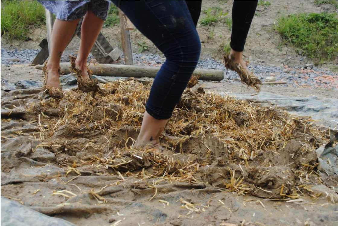
Photo 7.5 Bare feet 'puddling' cob in preparation for a building project at Embercombe (author photo).
