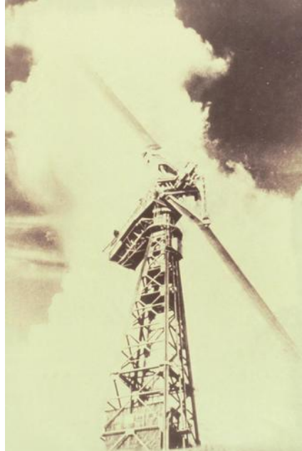
Figure 7 The Smith-Putnam MW wind turbine built in Vermont, U.S.A. in 1941[Source: NREL].
