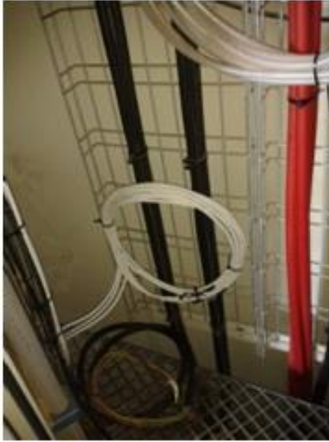
Figure 102 Stator current sensor installation. The photograph is courtesy of INDRA.
