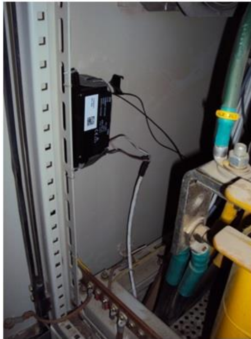
Figure 100 Photograph showing the BCC Bus sensor. The photograph is courtesy of INDRA.
