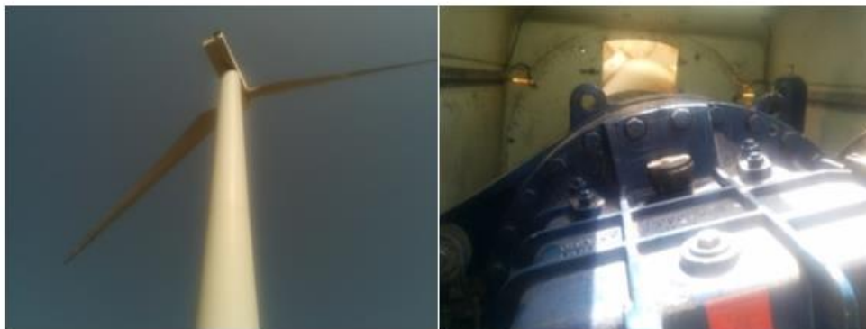
Figure 122 The 850 kW wind turbine and gearbox monitored using AE.
