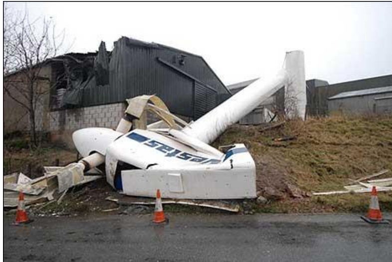
Figure 11 Collapsed wind turbine in Scotland in 2008 [Image Source: The Guardian].
