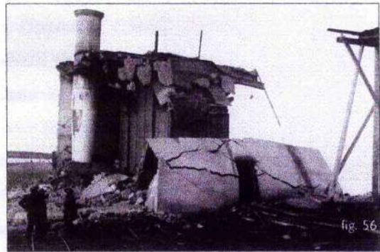
The power station at Kongsfjord, which supplied power to the Spitzbergen mines, demolished during GAUNTLET.
