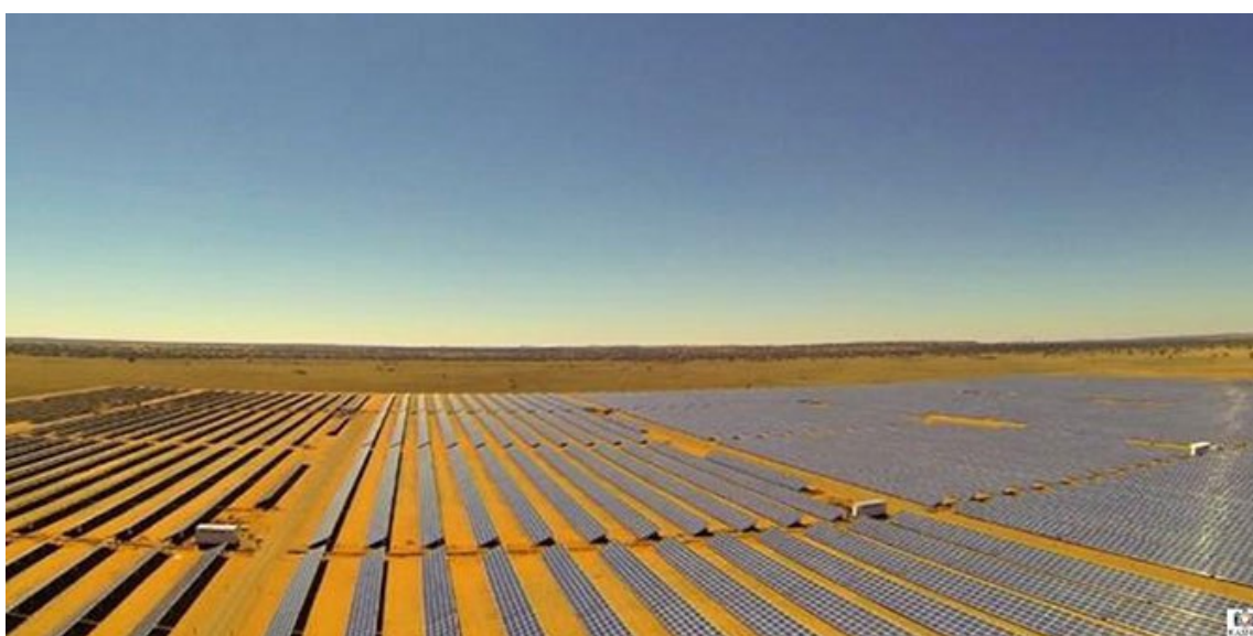
The Drogfontein solar plant near Kimberley opened in 2014 Photo Credit: Kasif Parthan via Flickr ( http://bit.ly/2iHSqvo ) CC BY-SA 2.0
