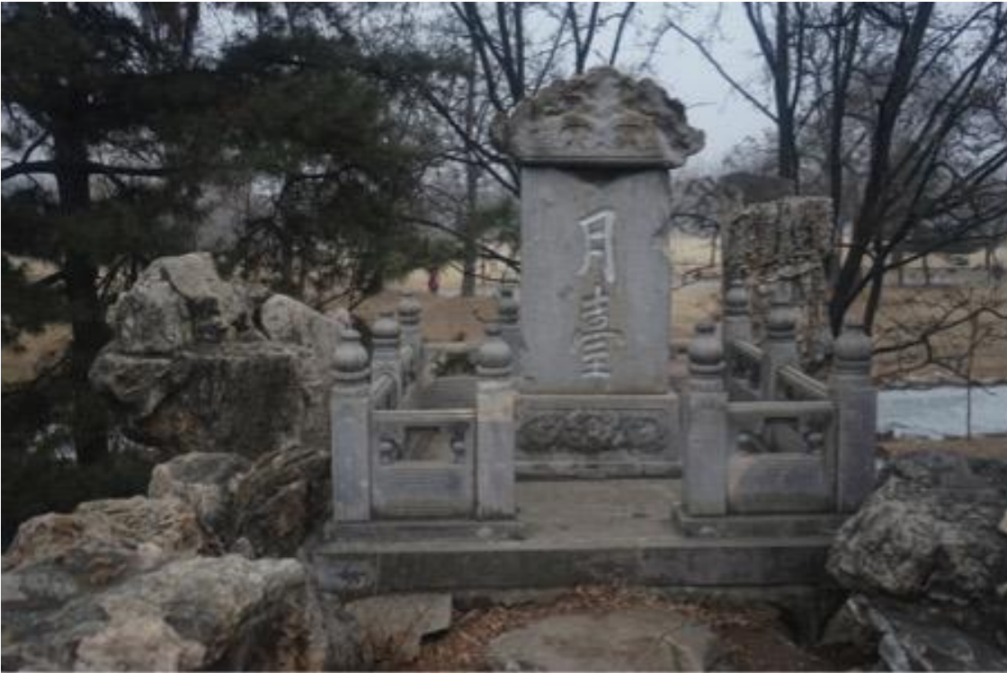
Figure 5-3: The Moon Platform on the rockwork in Wenjin Chamber, Chengde Imperial Mountain Resort. It is a small stone platform placed on rockwork, which is quite different from the huge ancient platform that had been constructed from rammed earth. (Source: author, 2014.)
