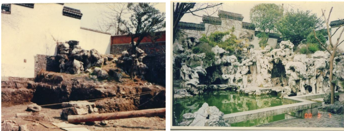
Figure 6-13. The rockwork at the north east corner, before (left, taken in 1989) and after (right, taken in 2000) the restoration. (Source: Administration Office of He Garden ( He yuan guanlichu 何园管理处), 'Heyuan jianzhu Lülibiao (pianshi shanfang jiashan xiujian Lülibiao) 何园建筑履历表 (片石山房假山修建履历表) [Resume of Buildings in He Garden (Resume of the Conservation of the Rockwork in the Mountain House of Sliced Stones)]', held by the Administration Office of He Garden ( He yuan guanlichu 何园管理处).)
