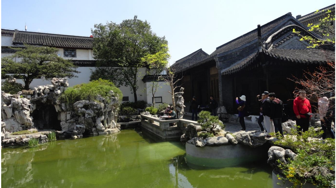
Figure 6-17. Current east and south side of the garden, where the repaired and renovated revetment can be found. (Source: author, 2013.)
