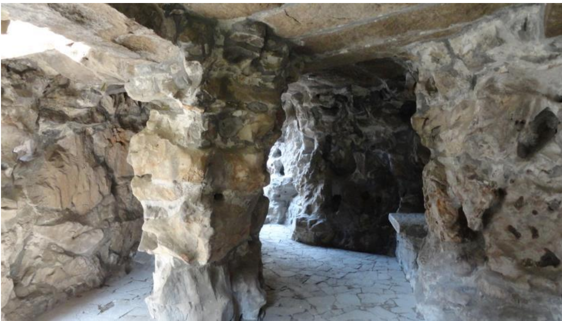
Figure 2-20. The rockwork in the Pan Gu Garden ( Xiao pangu 小盘谷), Yangzhou. The ceiling was made of linear stones. (Source: author, 2013.)
