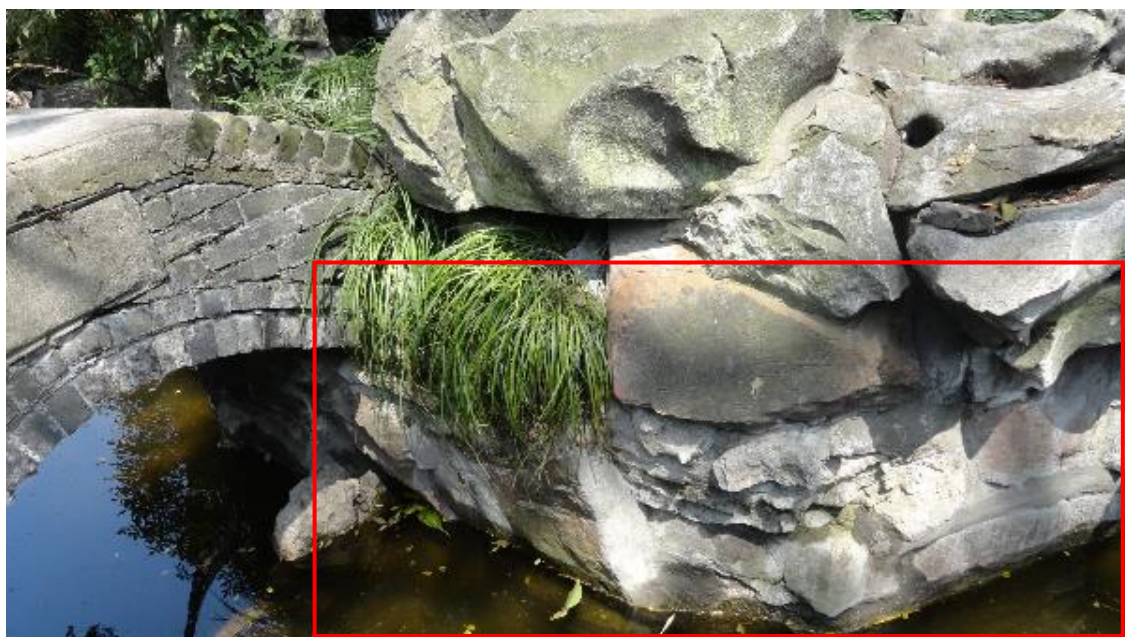
Figure 4-14. Yellow Rocks were used under the stream and the embankment but covered by Taihu Rocks. Rocks in the red frame are Yellow Rocks. (Source: author, 2013.)
