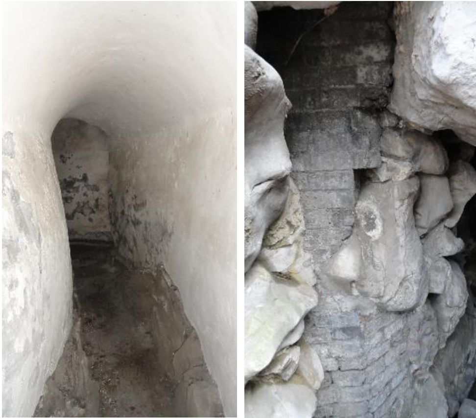
Figure 4-10. (Left) Linear cave made of brick walls; the bottom part is made of Yellow Rocks. (Source: author, 2013.)
