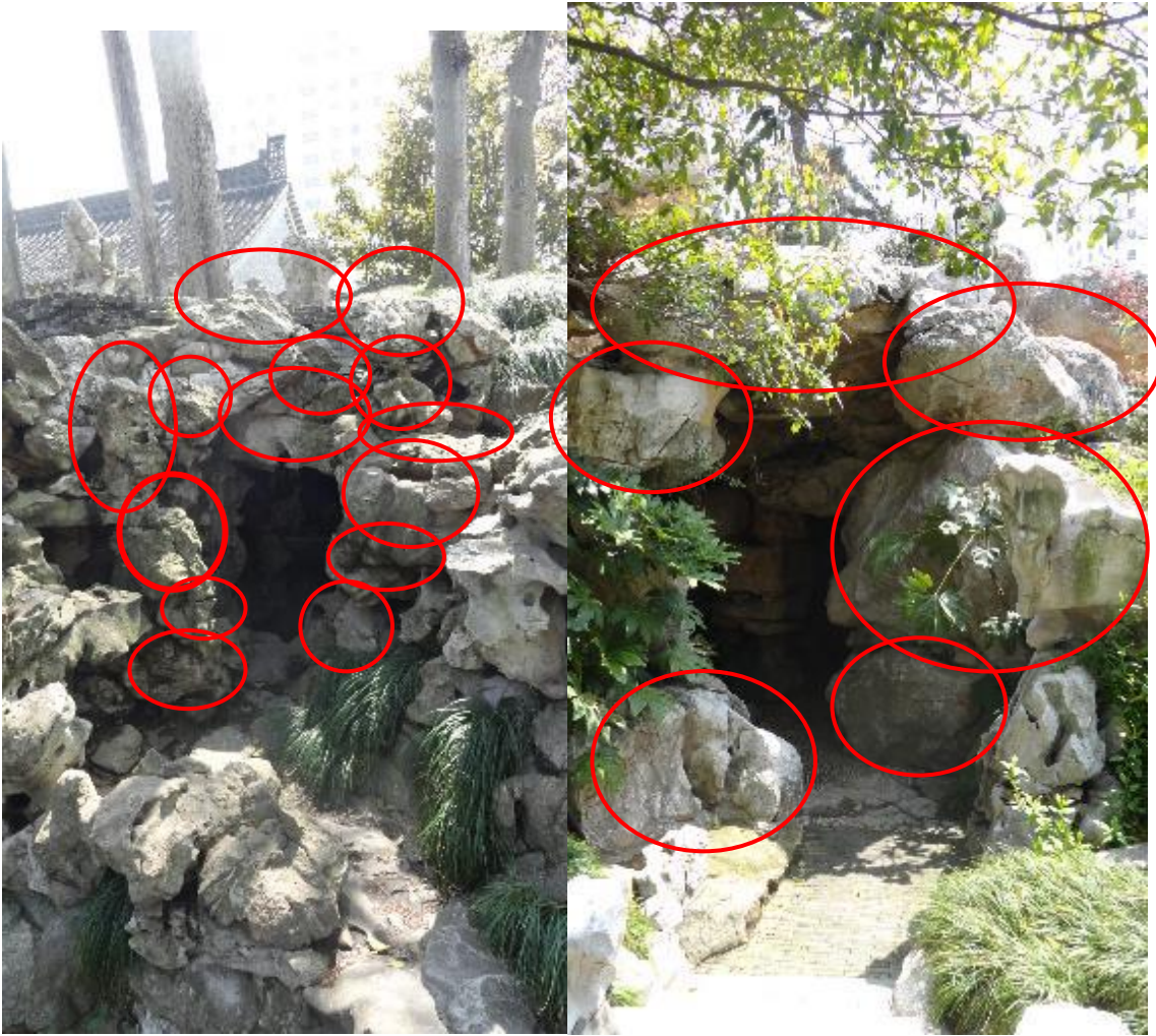
Figure 4-21. The comparison of the size of rocks used in the historical rockwork (left) and the newly constructed rockwork (right). The red circles show the size of rocks used at the entrance of caves. (Source: author, 2013.)
