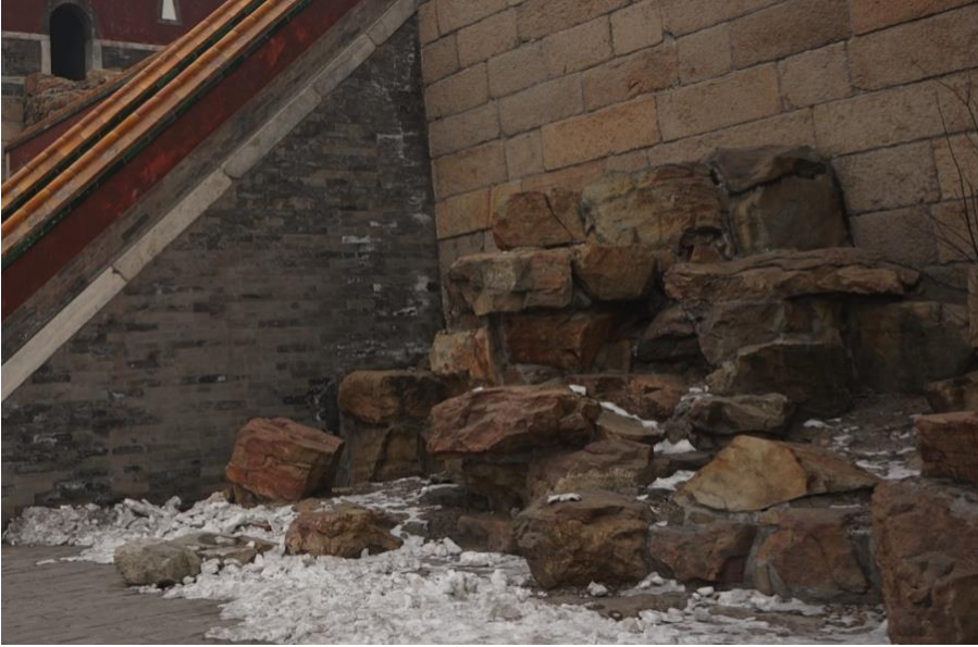
Figure 1-2. Rockwork constructed with Yellow Rocks in the Summer Palace, Beijing. (Source: author, 2014.)
