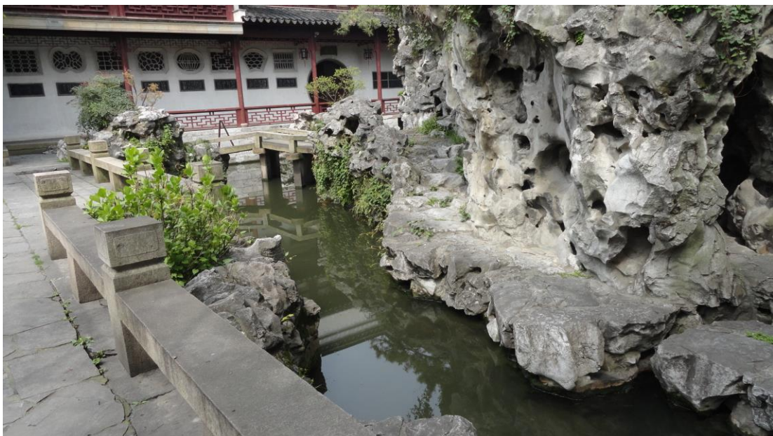
Figure 8-2. The historic rockwork in Mountain Villa with Embracing Beauty ( Huanxiu shanzhuang 环秀山庄) in Suzhou, which was constructed by Ge Yuliang and shows narrow joints between rocks, which are nearly invisible from a distance. (Source: author, 2013.)
