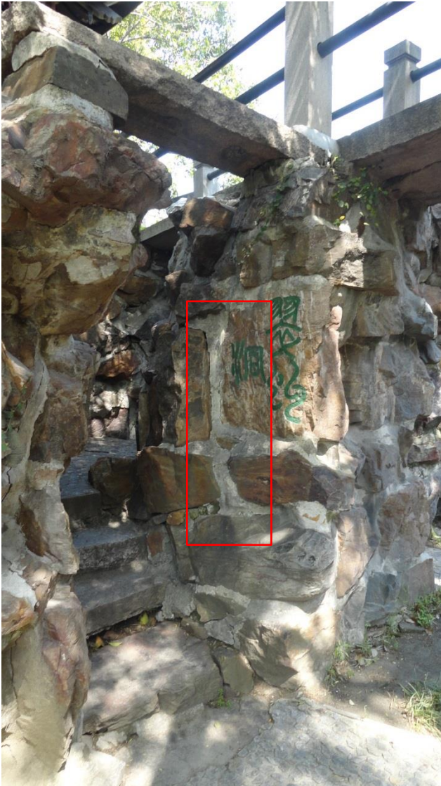
Figure 8-3. Repaired historic rockwork in the Garden of Fuzzy Boundary ( Xukuo yuan 虚廓园); the rectangular frame shows the wide joints left by the repointing process. (Source: author, 2013.)
