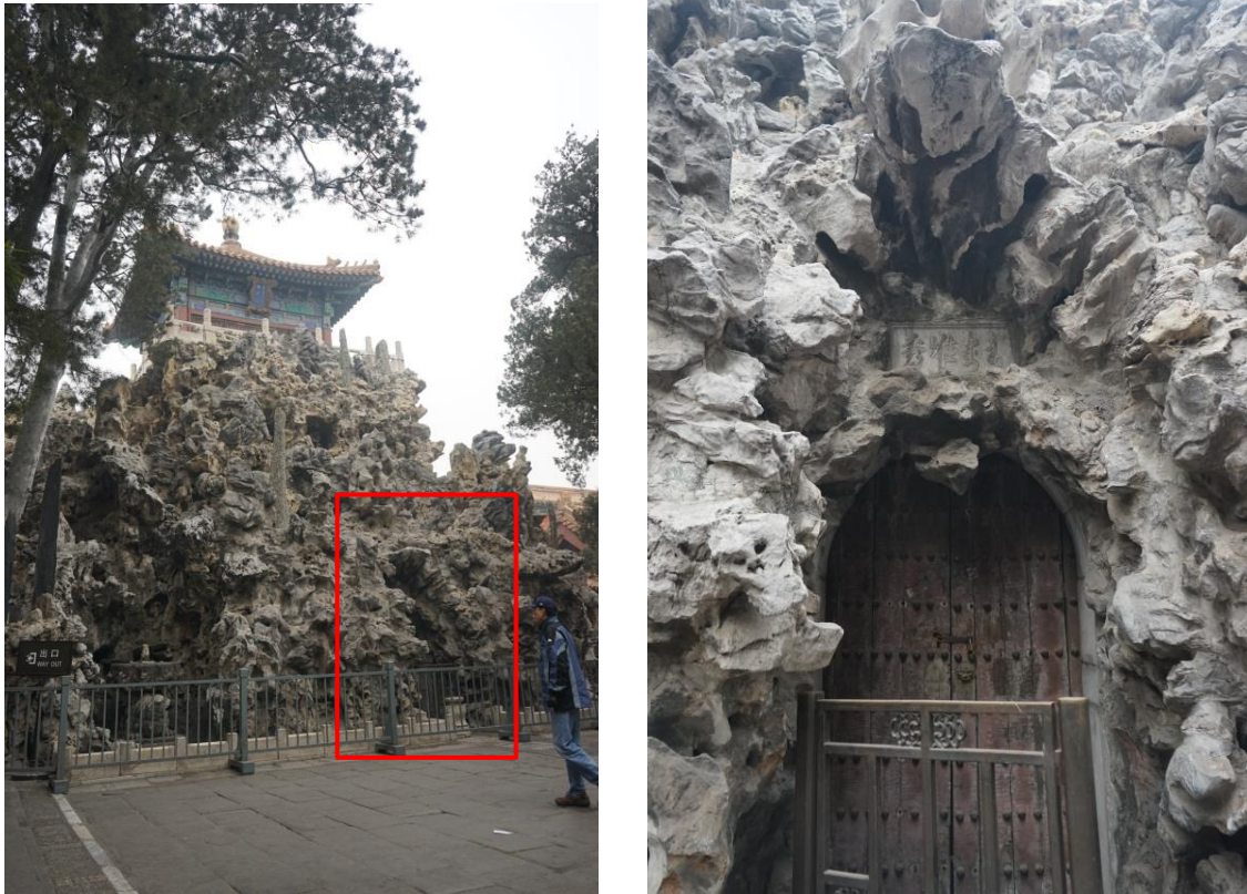
Figure 2-4. The rockwork named Piling Up the Delicacy ( Duixiu 堆秀) in the Imperial Garden of the Forbidden City, Beijing. It was made of a large number of bizarre Fangshan Rocks; many pointed Bamboo Shoot Rocks were also displayed on it as peaks. The image on the right shows the entrance of the cave, which is labelled in the red frame of the left image. (Source: author, 2014.)
