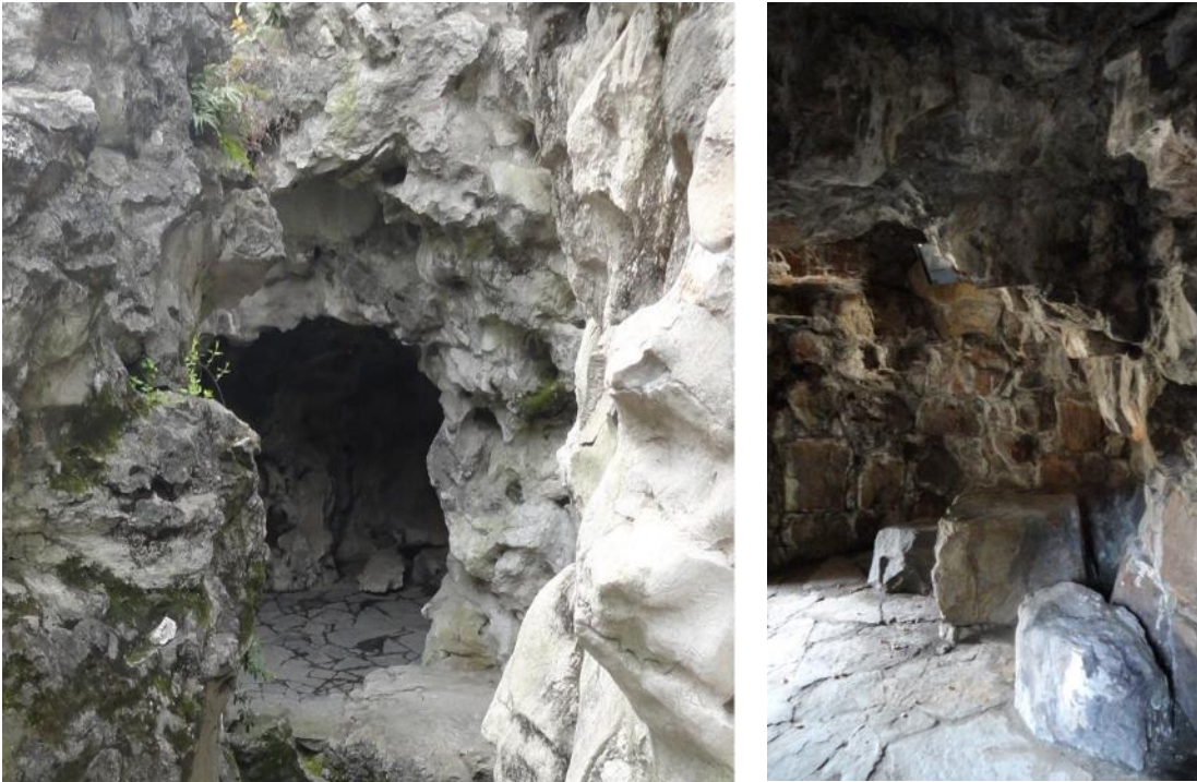
Figure 2-19. The 'Hook and Connect Method' that Ge Yuliang applied in the caves of Mountain Villa and the Swallow Valley. (Source: author, 2013.)
