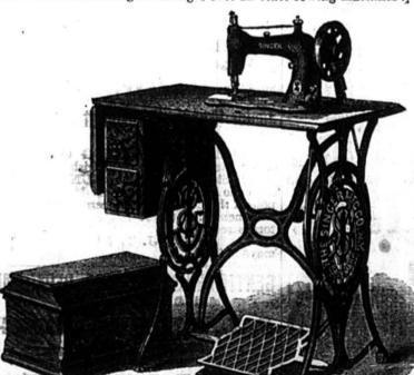
1st Uses the shortest needle of any lock-stitch machine. 2nd-Carries a finer needle with given size thread.
