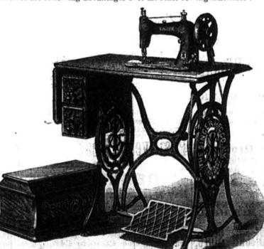
1st. Uses the shortest needle of any lock-stitch machine. 2nd-Carries a finer needle with given size thread.
