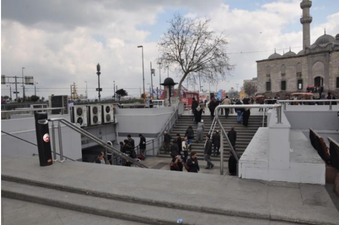
Figure 3.25 : Pedestrian underpass in Eminönü Square (Personal archive)
