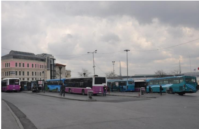
Figure 3.26 : Bus Stations in Eminönü Square (Personal archive)
