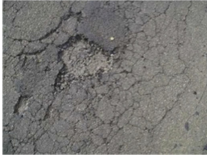
Fig. 1. Wear losses on pavements by aging effect.
