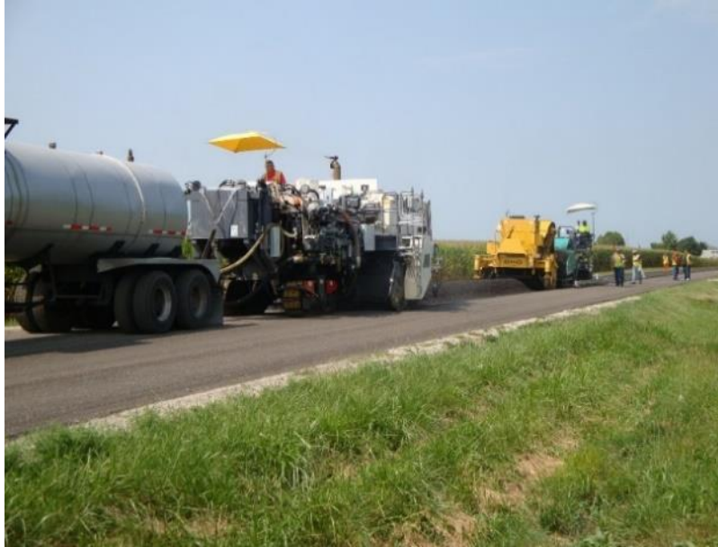
Figure 1.2 (left). Photo. Conventional mill and fill train (Wirtgen Group)
