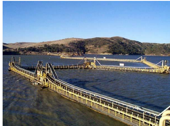
Figure 33. A large floating conveyor in a gravel mine in California.
