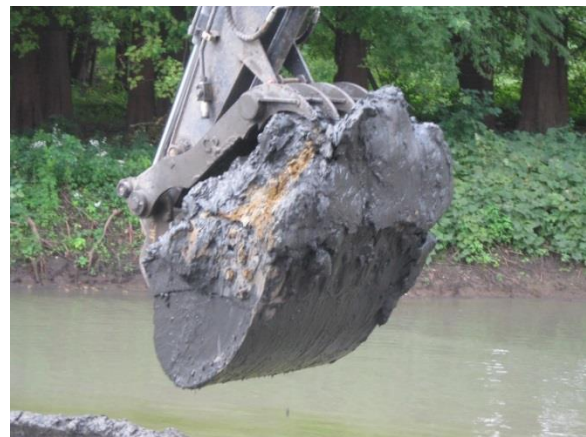
Figure 23. Heaped excavator bucket. Note color differences in this stiff material from below the soft sediment layer at Rice Lake.
