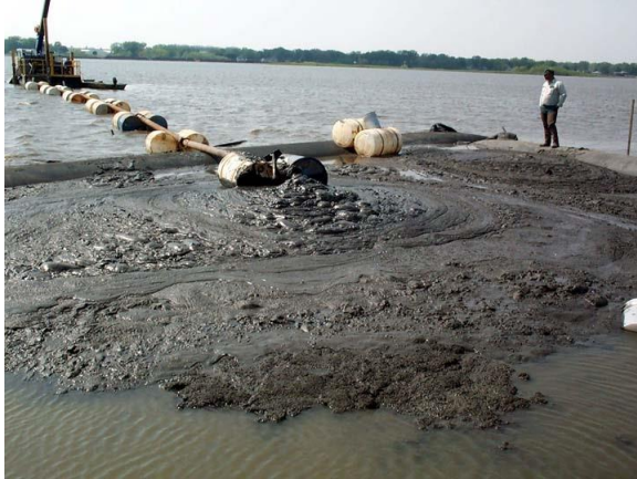
Figure 24. Cohesive dredged material forming a mound as it comes from Dry Dredge™ pipe.
