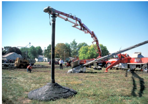
Figure 27. Sediment leaves the placing boom, which can be moved to spread the sediment.
