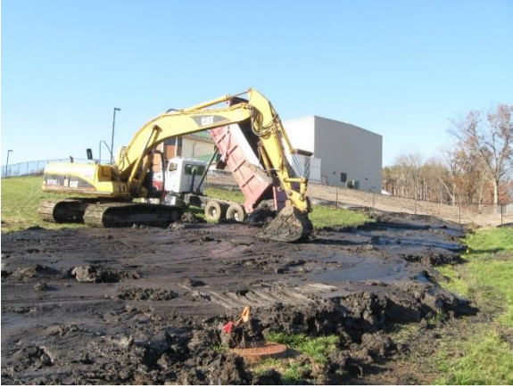
Figure 65. Sediment from Walton Lake is placed at the Litchfield water treatment plant and smoothed to the desired thickness.
