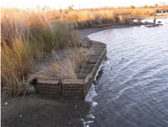
Figure 73. Hesco Units™ near Ft. Pike in La. survived Hurricane Katrina. They have the potential for marsh restoration and habitat enhancement.
