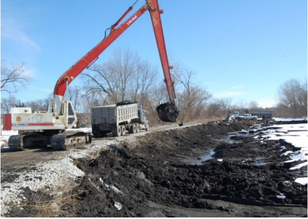
Figure 58. Hydraulically dredged sediment is loaded onto trucks from a dewatering basin by the Fox Waterway Agency.
