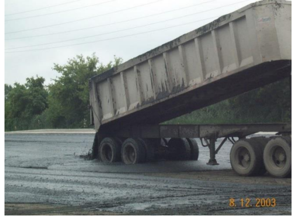
Figure 76. Wet biosolids are seen pouring from a truck onto a drying bed in Chicago.
