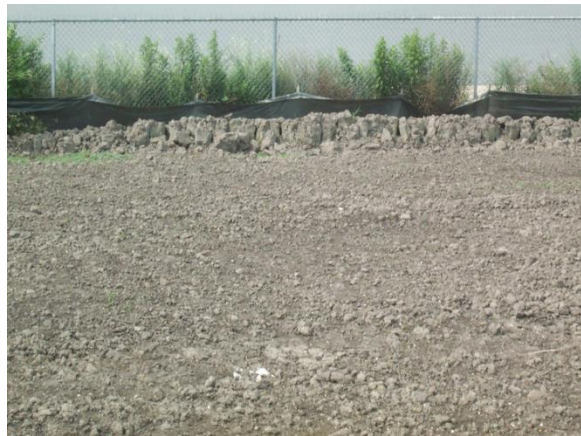
Figure 41. In June the material had dried and formed polygons as seen in the rear. A disk was used to break them up and level the field.
