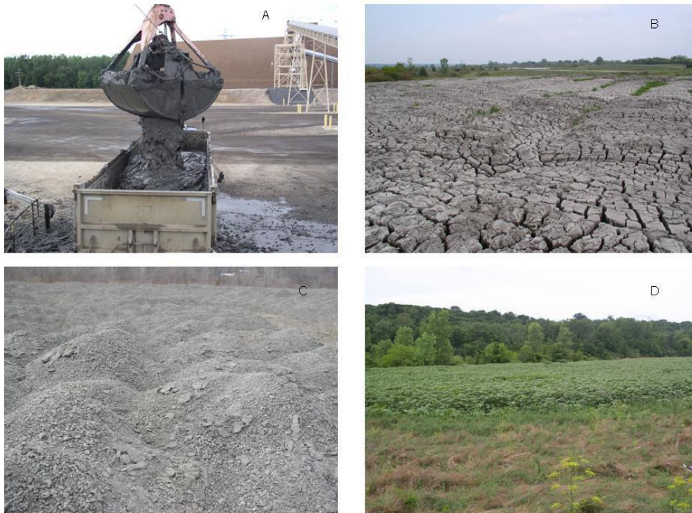
Figure C3. Sediment application to Banner Marsh State Fish and Wildlife Area: A, Truck receiving sediment from barge for transport to Banner Marsh pre-law strip mine area; B, Sediment drying one month after placement; C, frost shattered sediment polygons the following spring; D, Planting of sunflowers thriving on sediments after tillage, foreground is untreated.
