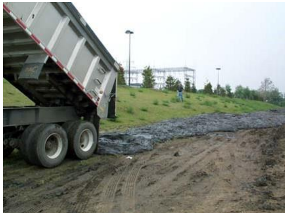
Figure 39. The Spindler material was dumped from moving trucks in April 2000 on level compacted ground at a former power plant.
