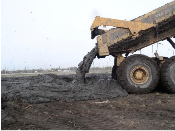
Figure 18. Material deposited at USX from most barges was cohesive and formed piles.
