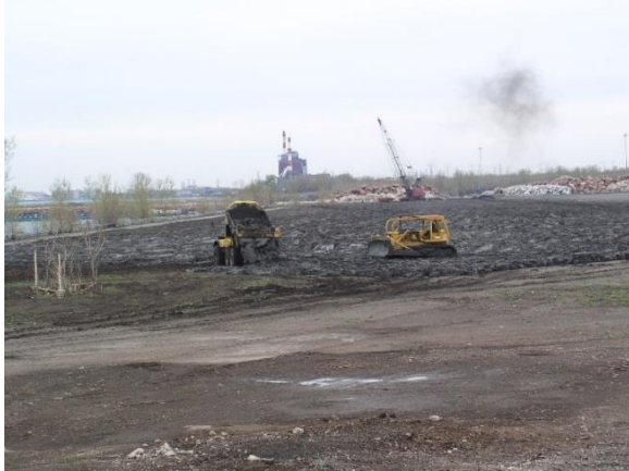
Figure 46. Placing sediment south of the slip at USX in March 2004.
