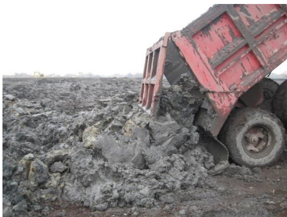
Figure 50. In 2012, material dredged where the East Port channel neared the shore was light colored and sticky. It was difficult to handle.
