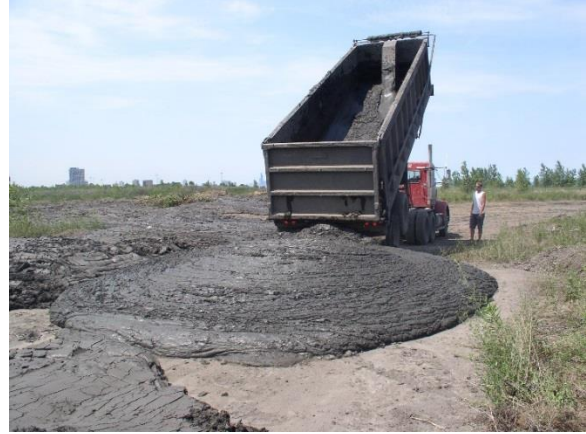
Figure 19. Material from the few “wet” barges was more fluid but not enough to cause concern.
