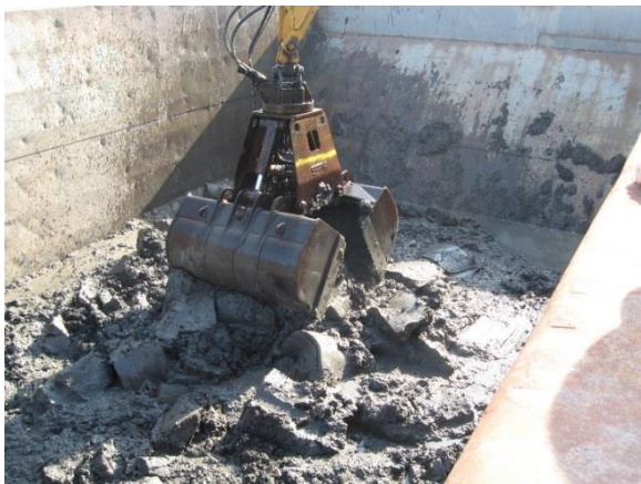
Figure 22. A hydraulic clamshell bucket depositing drained material in a barge.
