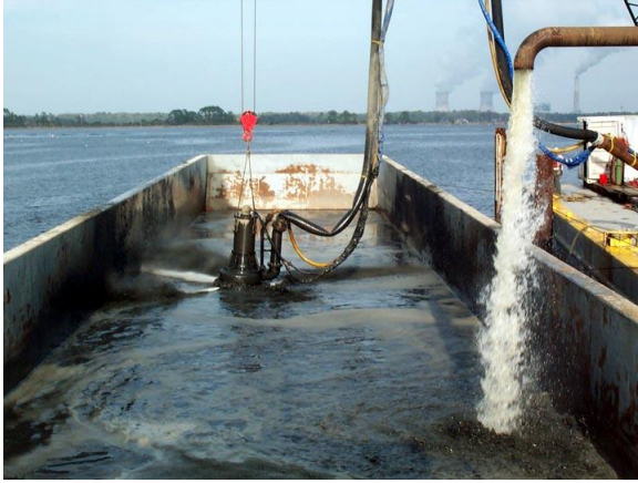
Figure 36. Water is added to a barge load of fine-grained dredged material at Jacksonville, Fla., for pumping by a slurry pump.
