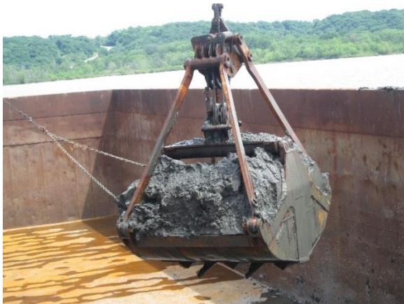
Figure 20. A conventional bucket with sediment heaped does not carry much free water.
