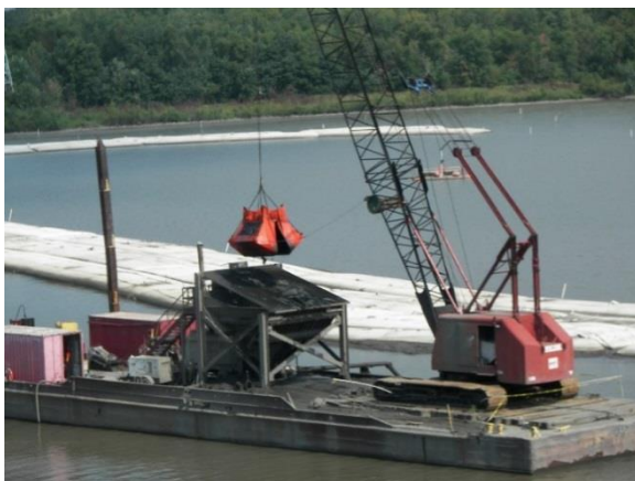
Figure 28. Soft sediment is placed in a mud hopper feeding a displacement pump during island construction on Lower Peoria Lake.
