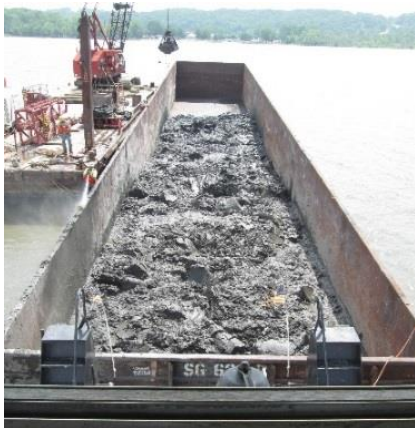
Figure 16. Crane operator has allowed very little free water to enter this barge.
