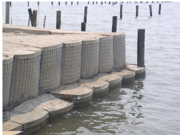
Figure 74. Hesco Units, shown here near New Orleans, come in several sizes and can be placed at various heights and in different patterns.
