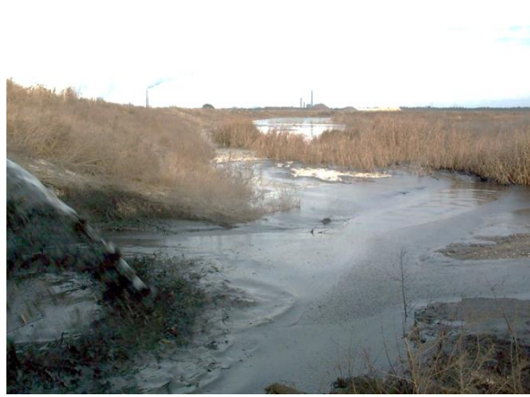
Figure 37. Material the consistency of thick molasses flowed from the pipe and spread across the CDF without blocking the discharge point.
