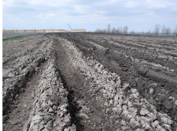
Figure 47. A bulldozer and mining trucks left furrows in the sediment, which aided drying.
