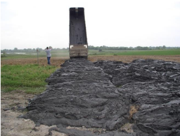
Figure 56. Sediment from Rice Lake poured in long lines from moving trucks onto strip mine overburden at Banner Marsh SFWA.
