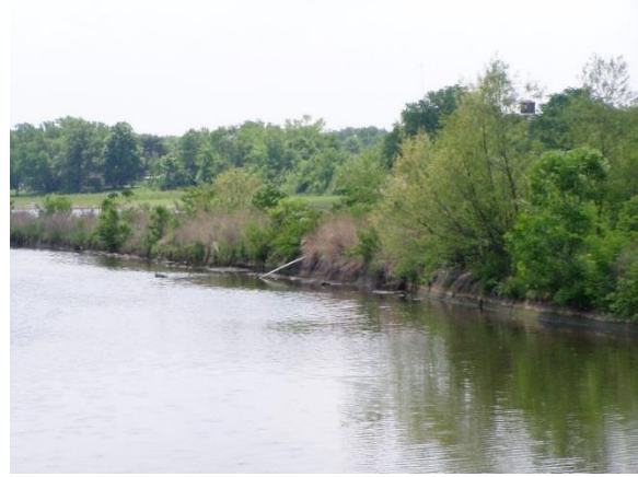
Figure 70. Trees and other vegetation were planted in geotextile tubes in a sheltered inlet on Old Hickory Lake in Tennessee.
