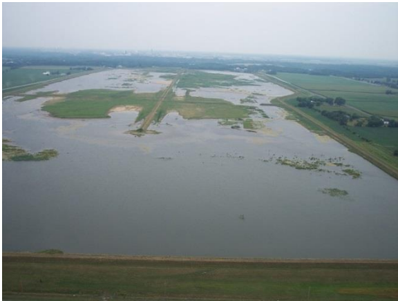
Figure 14. Dewatering basin for the Lake Decatur water supply reservoir dredging project.
