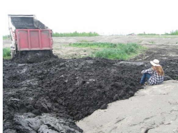
Figure 51. On 6-5-2013, sediment from Spindler Marina near the navigation channel handled easily and was essentially friable.
