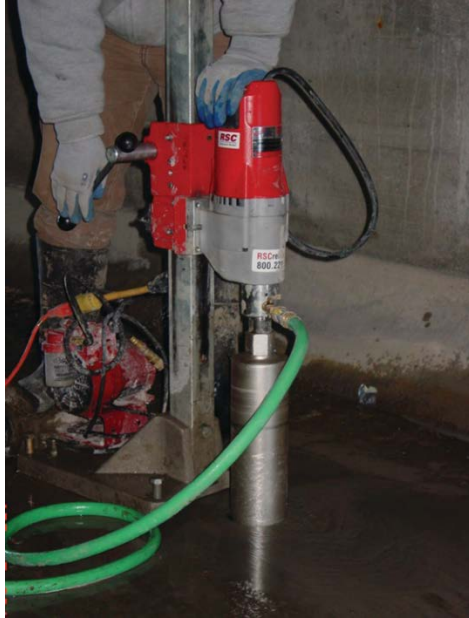
Figure 2.5. PCC drilling.
