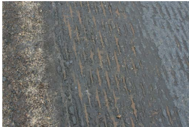
Figure 4.2. Brown, “unbroken,” emulsified-asphalt prime coat on US 52 Laraway Road to Gougar Road—contract 60N08.
