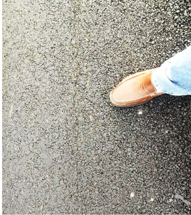
Figure 4.11. Evidence of hairline crack at underlying transition from level binder to no level binder. Level binder (4.75 mm) to left of crack and milled surface to right of crack. Increased segregation also at pavement edge (right side of photo).
