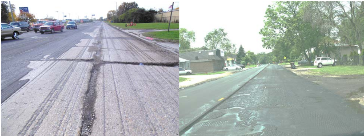
(a) Crawford/Pulaski Road after milling (2014)
