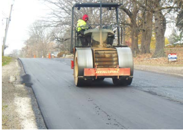
Figure 4.6. US 52 (60Y02) level binder construction with exposed, milled 12 in at edge.
