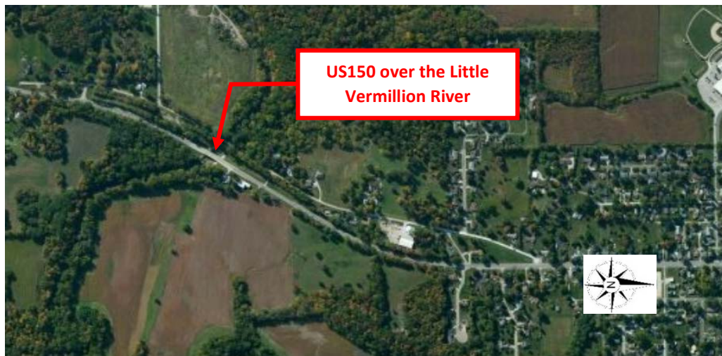
Figure L.1 Location of US 150 over the Little Vermillion River.
