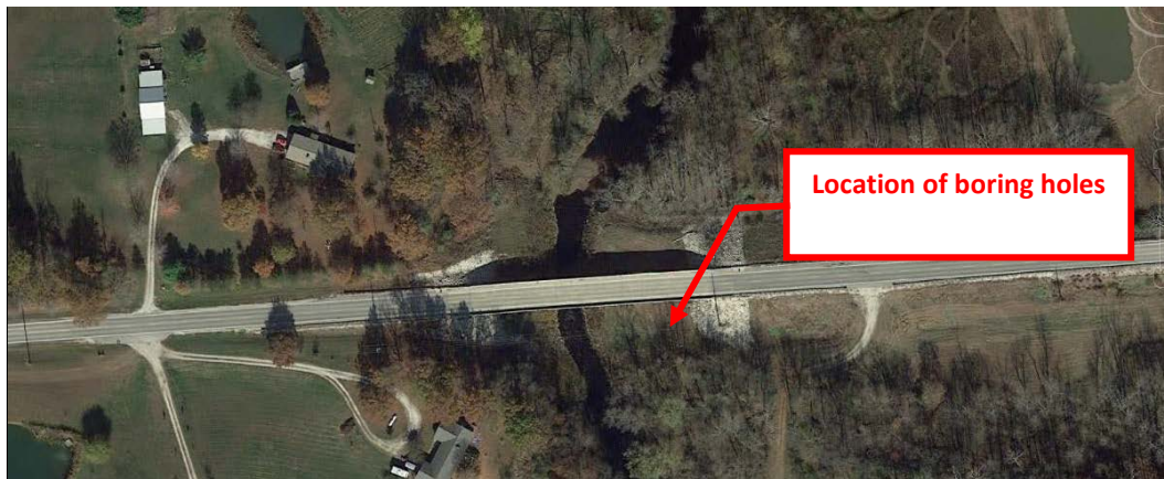
Figure N.2 Location of boring holes for obtaining MSPT blow counts and shale core samples.
