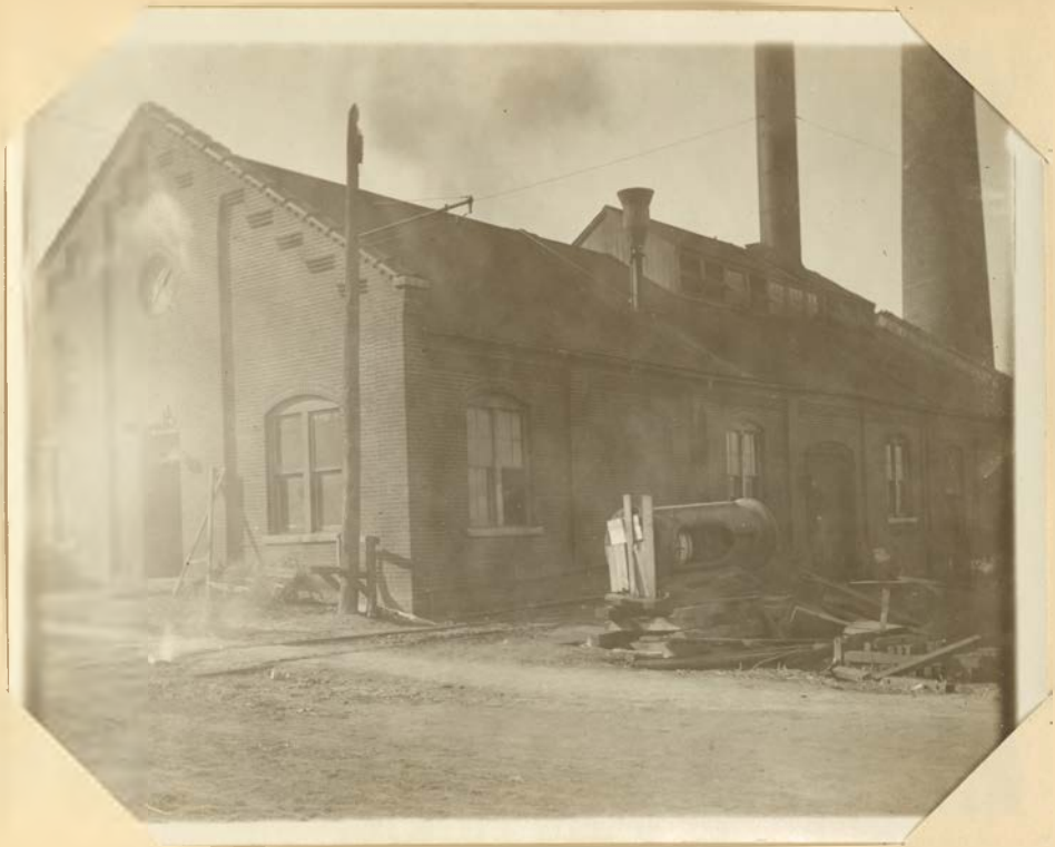
A view of the Present Power Plant.
