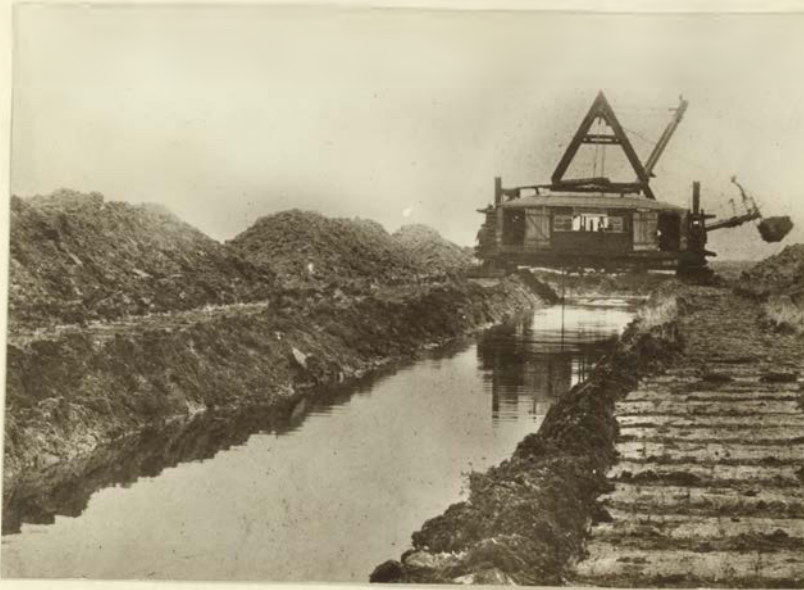
Walking Dredge Excavating Drainage Canal
