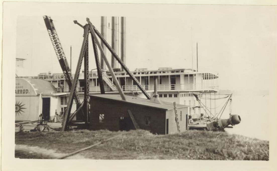
Stern Of Suction Dredge Showing Connection To Floating Line
