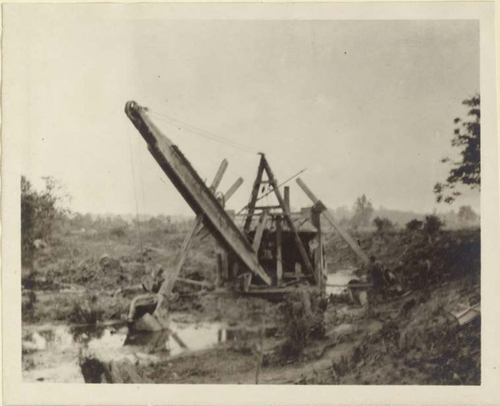
Floating Dipper Dredge Digging Drainage Canal
