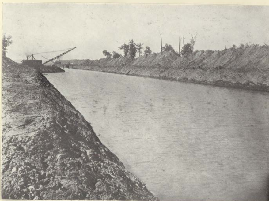
Drag Line Excavators Digging Large Canal
