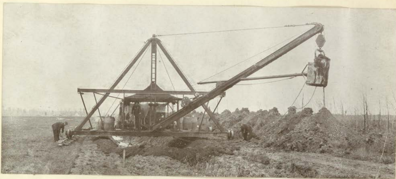
Dry Land Dredge In Operation
