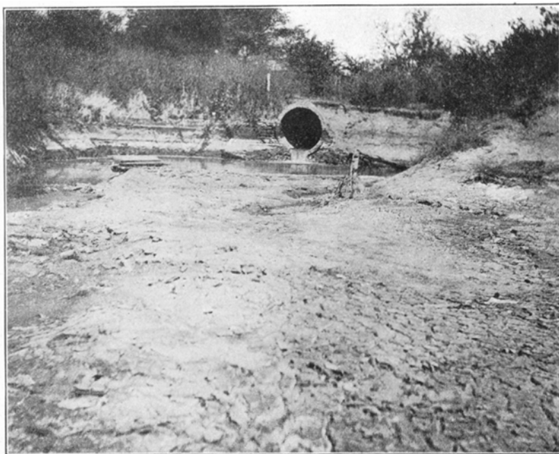
Broadway Sewer Outlet, Decatur. Note Heavy Sludge Deposits in the Fore-ground.
