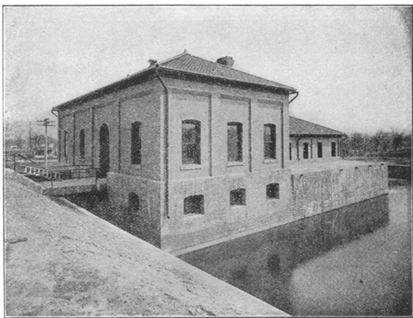
Fig. 2.—Exterior View of the Modern Mechanical Filter Plant at Rock Island. This Plant Is Built Within One of Four Abandoned Slow Sand Filter Units and Shows the Striking Contrast in Size.
