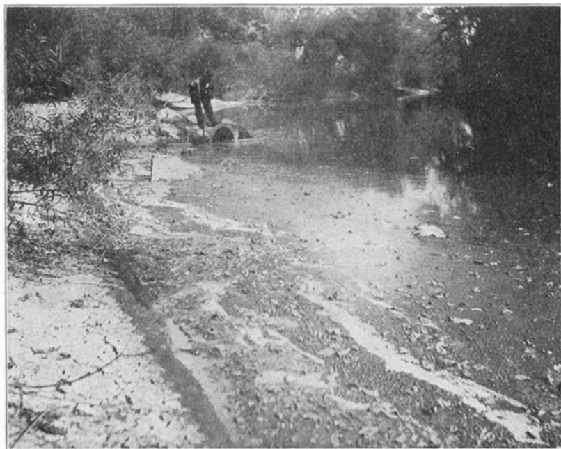
Oakland Avenue Sewer Outfall, Decatur. Note Heavy Deposit in the Foreground.
