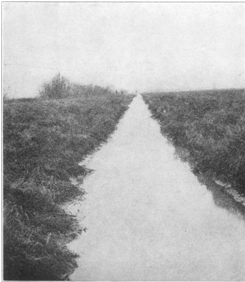
Fig. 3.—Ditch Carrying Effluent from Winnetka Septic Tank Along Roadside.
