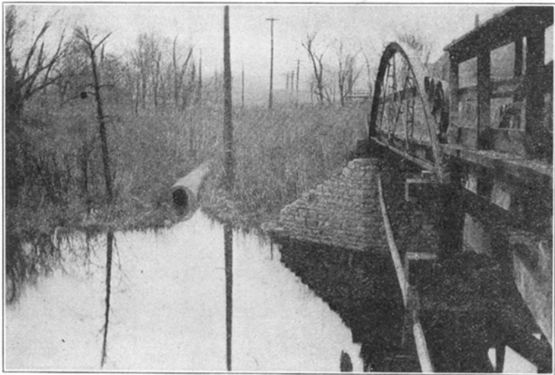
Fig. 1.—Outlet to New Sewer System, Morton Grove.
