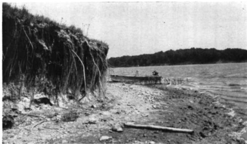
FIG. 5.—Wave erosion on north shore of Big Creek arm.
