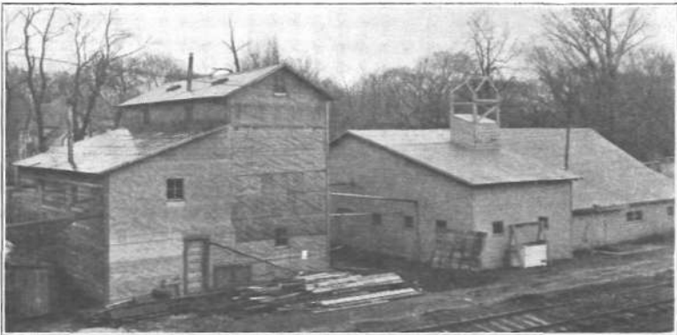
FIG. 3. GENERAL VIEW OF EXPERIMENTAL SEWAGE TREATMENT PLANT NOW IN OPERATION
