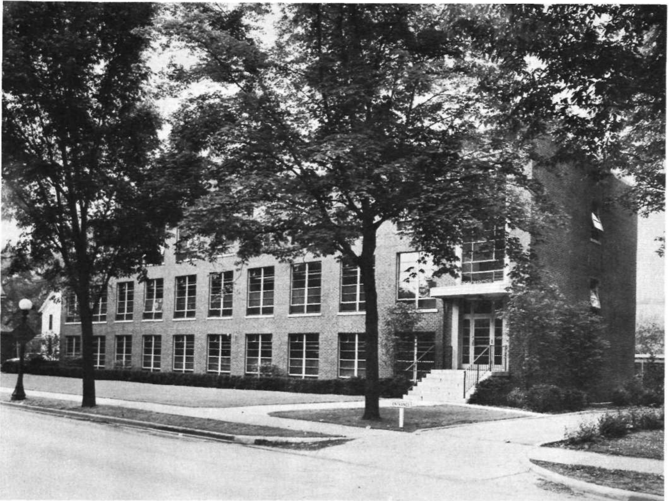
FIG. 1. THE WATER RESOURCES BUILDING AT URBANA.
