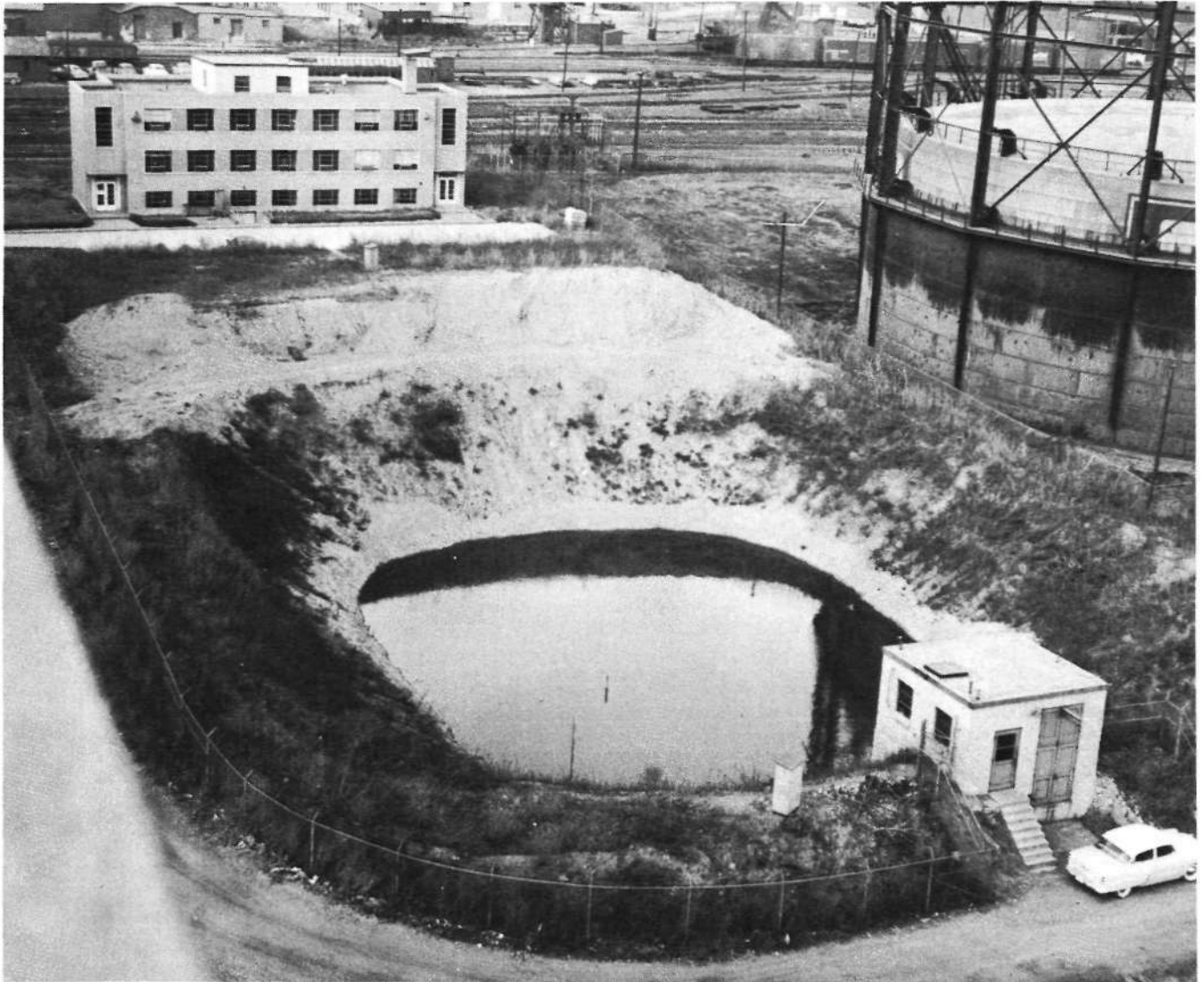
FIG. 8. VIEW OF WATER SURVEY FACILITIES AT PEORIA, SHOWING RECHARGE PIT AND BUILDING.
