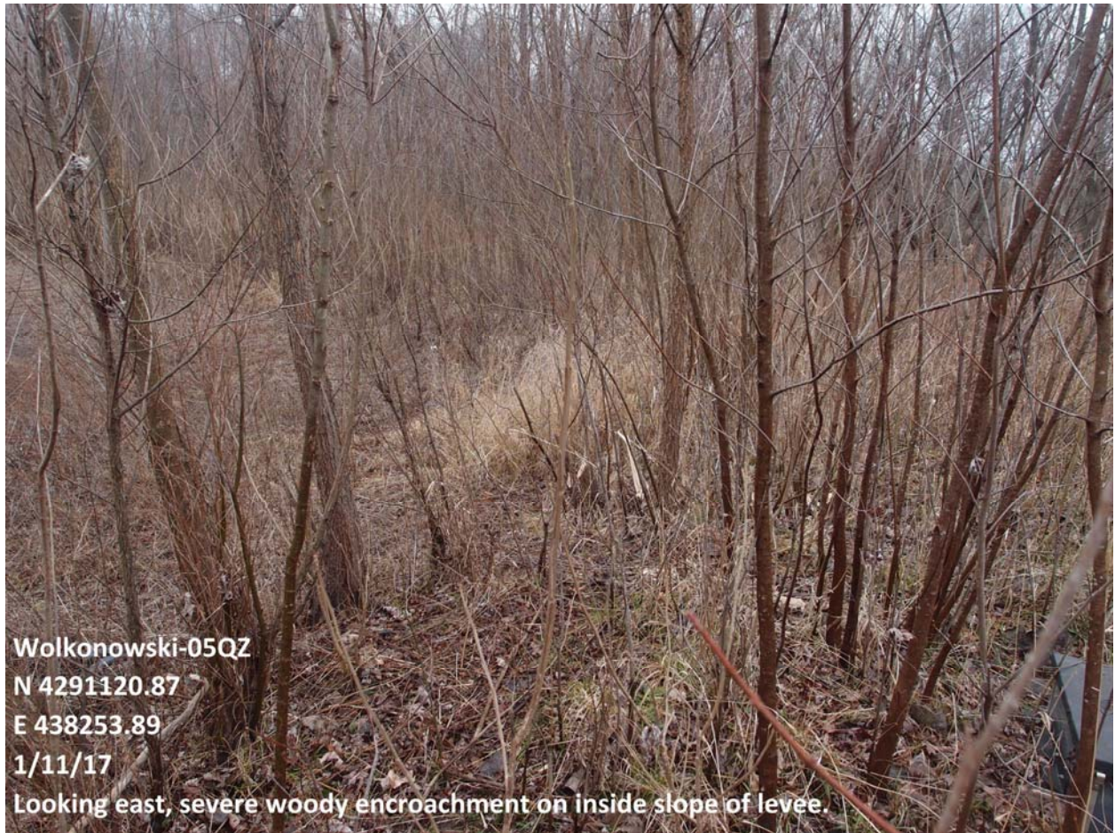
Photo 3: Woody encroachment on inner slope of levee.
