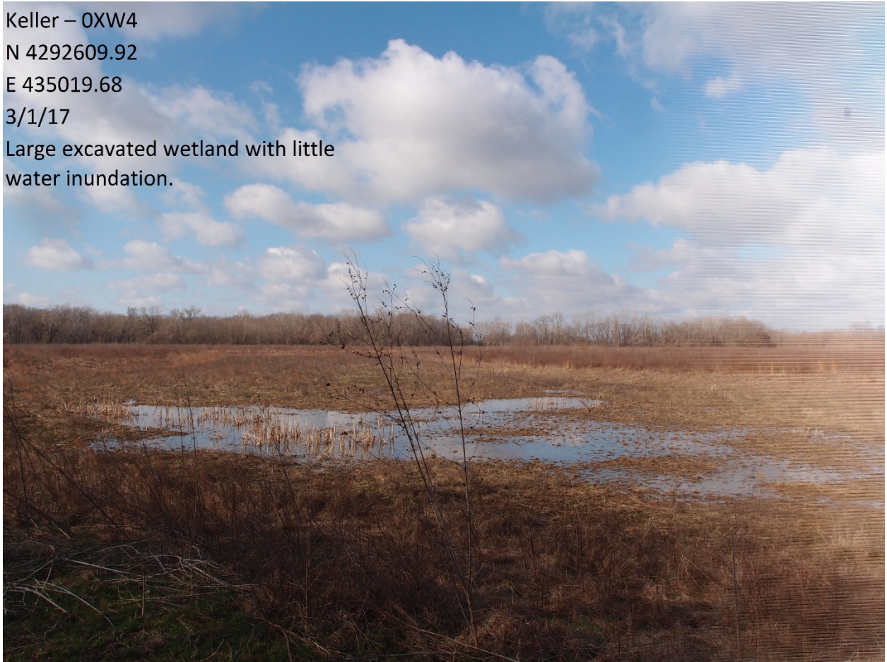
Picture 1: Wetland excavation with small amount of water inundation.
