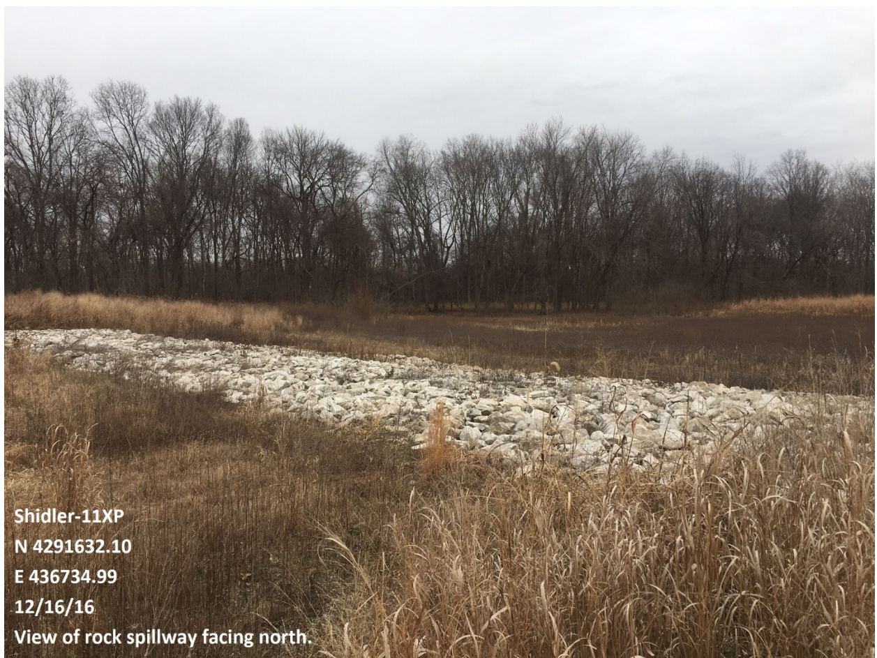
Photo 2: View of rip-rap spillway in working condition and free of debris.
