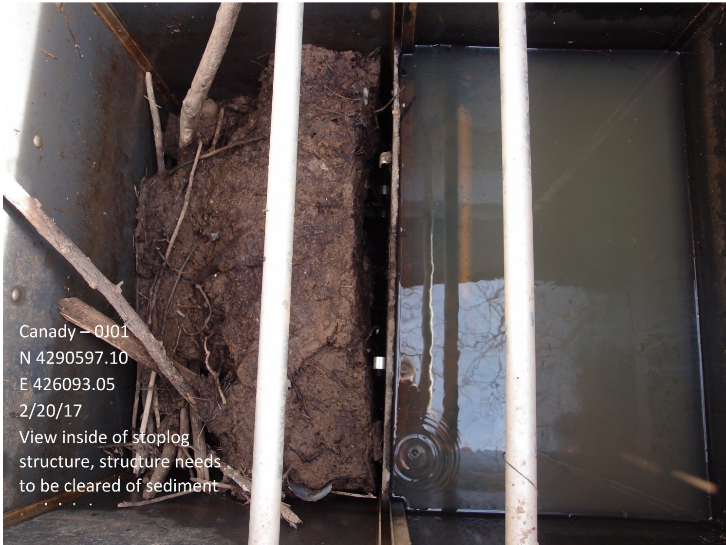
Picture 2: Sediment and debris preventing operation of stoplog structure.
