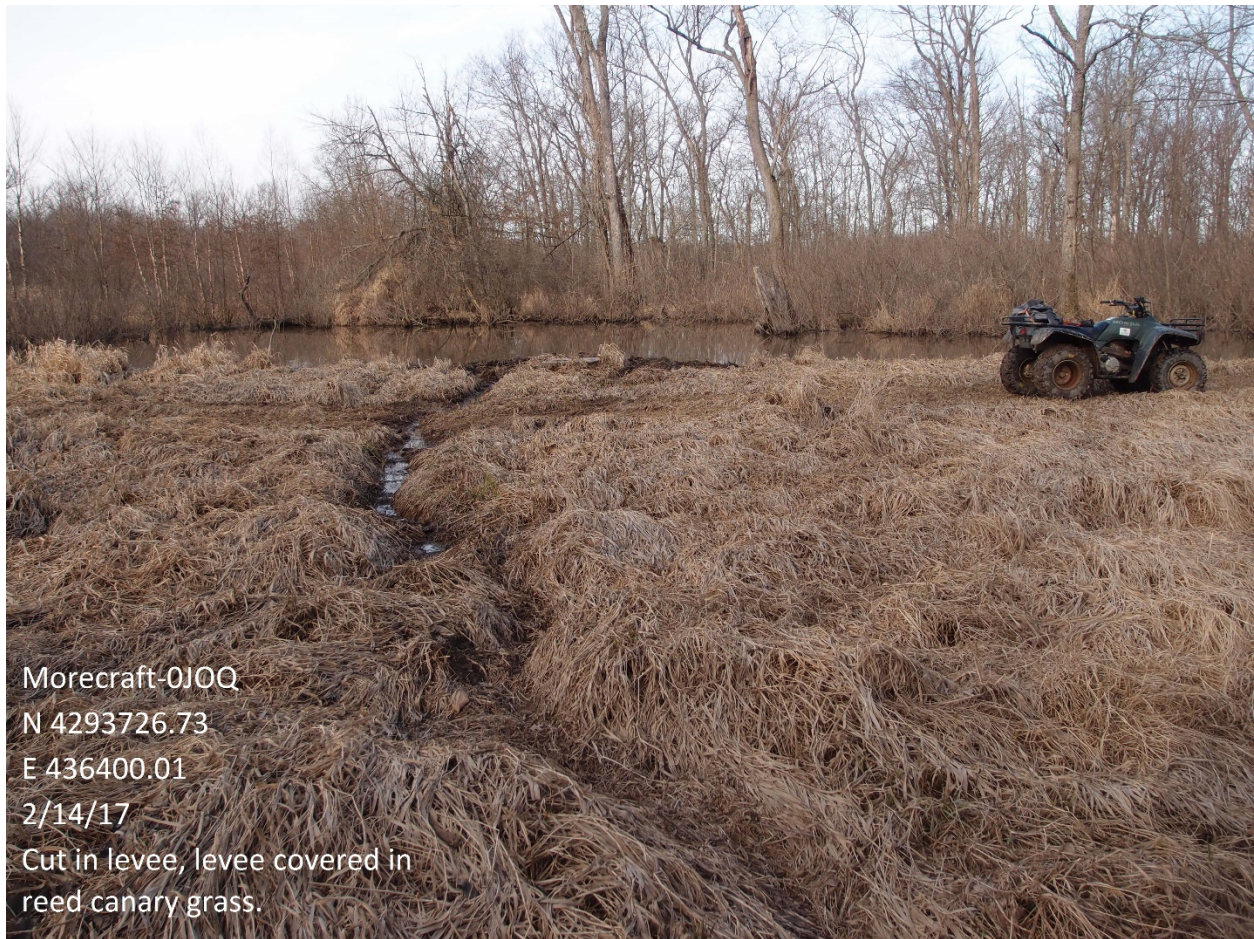
Photo 3: Cut in levee from high water levels in the impoundment.
