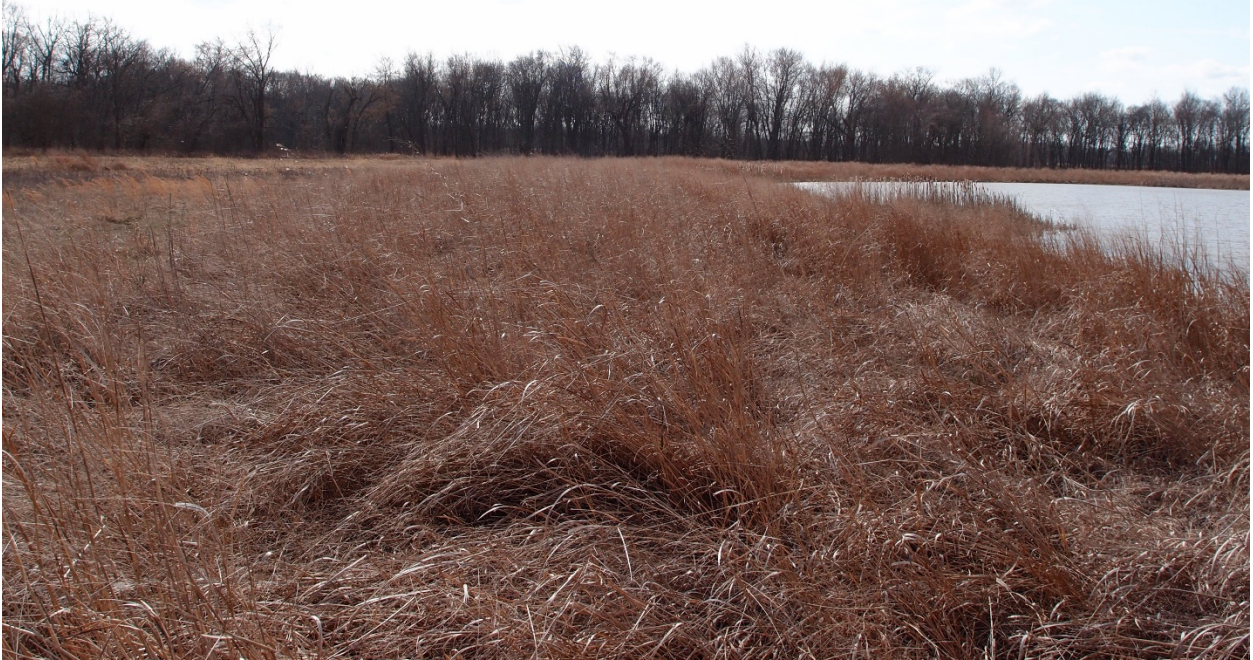
Photo 3: View of levee covered in tall switchgrass.
