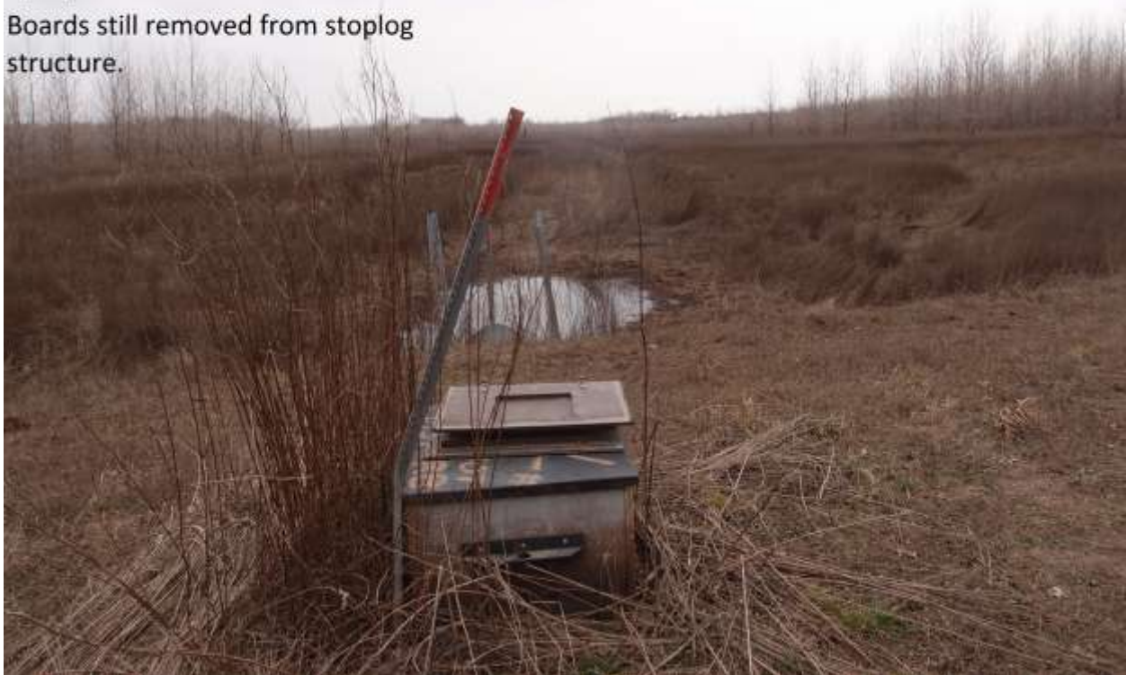
Photo 3: Westerly view of a dry impoundment on the ILDNR (OJOC) easement with the riser boards setting on top of the stoplog structure. Photo was taken in February of 2017.
