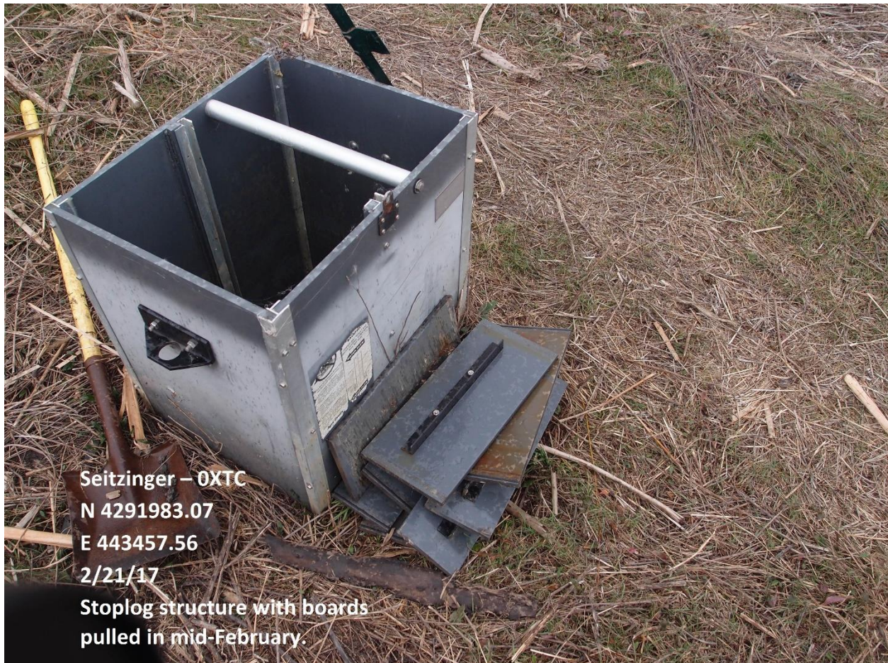
Photo 10. Stoplog structure on the NE portion of the the Seitzinger (OXTC) Easement in Lawrence County, Illinois. Photo was taken during February 2017, and all boards were removed from the structure allowing the wetland to dewater prior to spring waterfowl migration along the Embarrass River.
