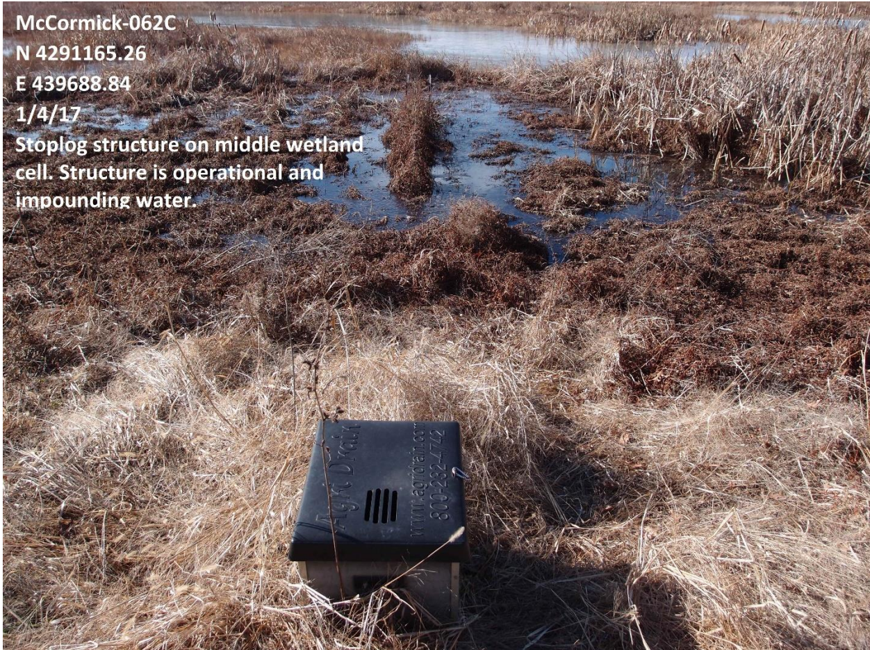
Photo 1. Stoplog structure with “beav-away” pipe installed.
