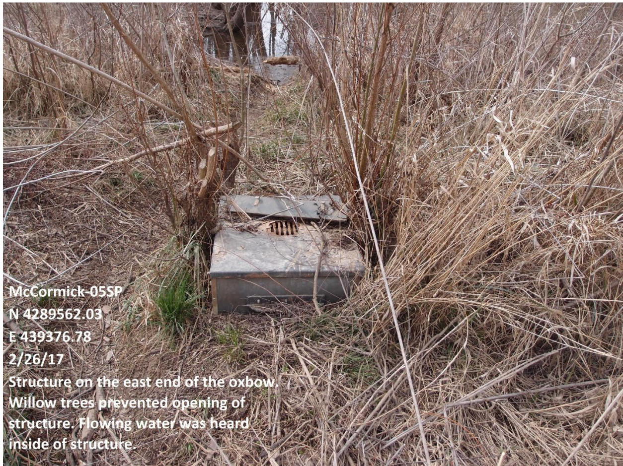
Photo 3: Water control structure on the oxbow lake. Willow growth prevented opening the structure.
