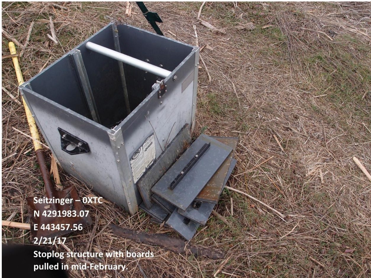
Photo 3. Stoplogs were removed from the water control structure on the Seitzinger OXTC Easement prior to spring migration of waterfowl in southeastern Illinois.
