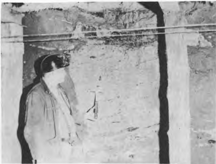
Fig. 6. - Calcareous conglomerate near center of south "cut-out" on west wall of 4th NW front entry. Crinoid stems and fossil fragments are abundant in this conglomerate.
