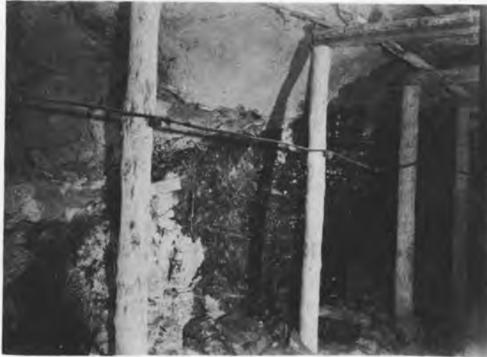
Fig. 8.- Contact between "cut-out" fill and coal showing upward bending of bands of coal toward the contact, on south side of north "cut-out" on east side of 4th NW back entry.
