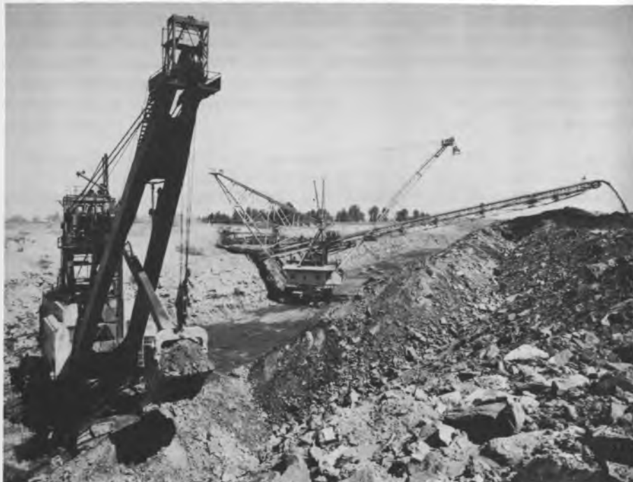
A. - Wheel excavator removing unconsolidated overburden from No. 6 Coal west of DuQuoin, Perry County. B. - Shovel stripping consolidated overburden, limestone, and shale, from No. 6 Coal following the wheel excavator.
