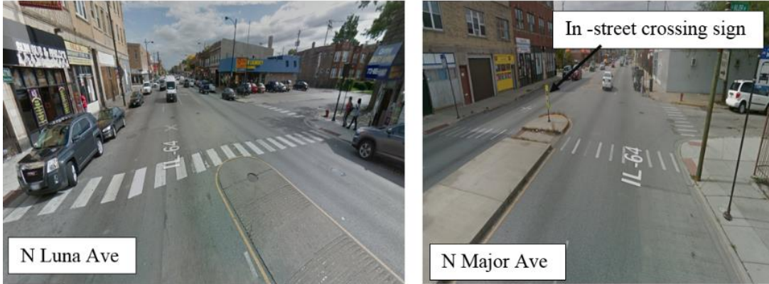
Figure E-73. Example marked crosswalk with refuge island at the intersection of W. North Ave. and N. Major Ave.
