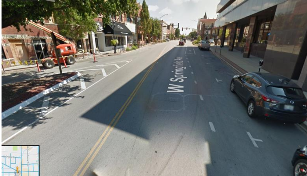
Figure E-50. Intersection of W. Springfield Ave. and W. Main St.
