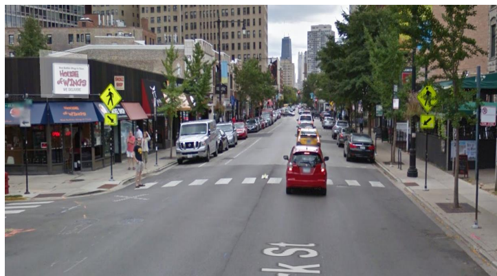
Figure 60. Pedestrian-crossing sign (dual back-to-back display) on N. Clark St., Chicago.
