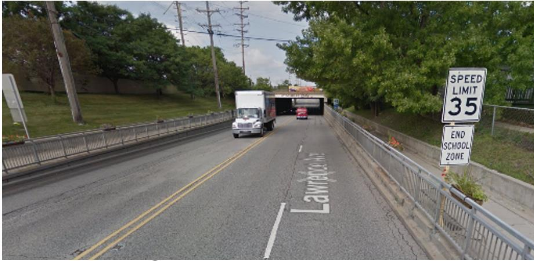
Figure E-86. Pedestrian channelization along Lawrence Ave. under the Metra Rail Bridge.
