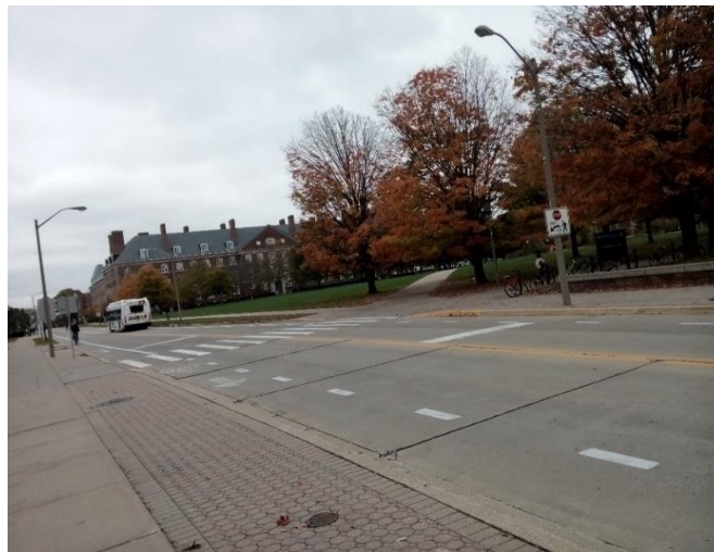
Figure 36. Example of the best practice of placing an advanced stop bar and sign.
