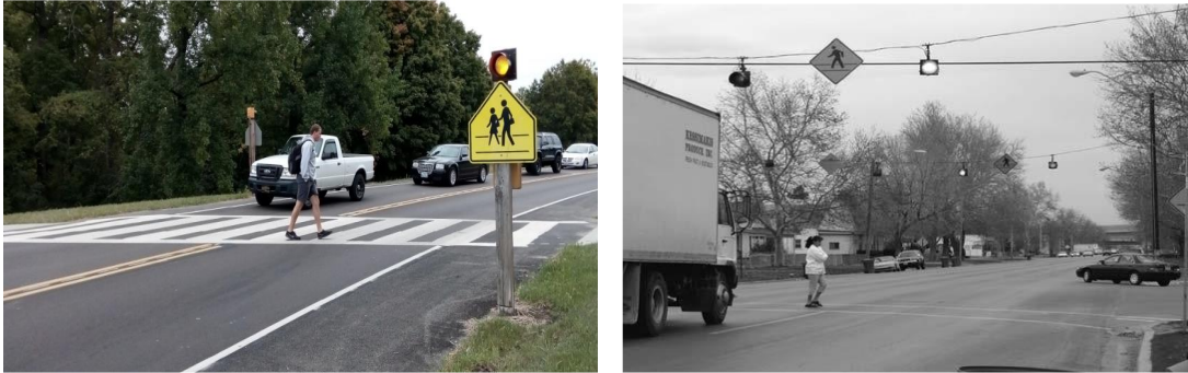
Figure 53. Pole-mounted and overhead flashing beacons (Fitzpatrick et al. 2006). Rectangular Rapid Flashing Beacon (RRFB)
