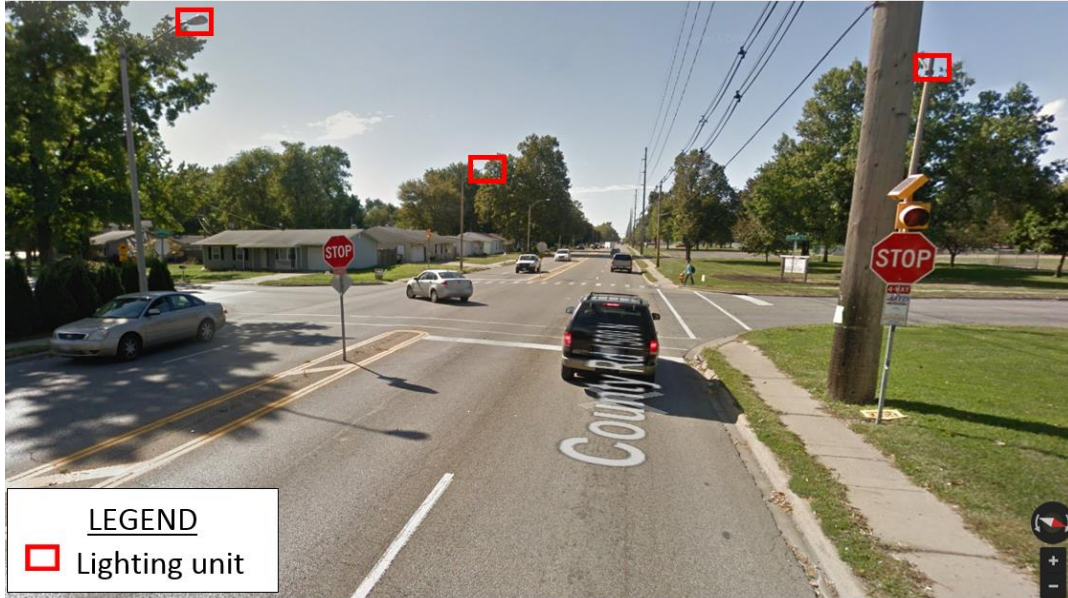
Figure E-42. Existing pedestrian treatment at intersection of Kirby Ave. and Crescent Dr.
