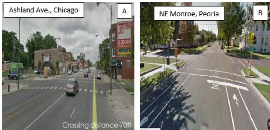
Figure 30. (a) Wide crossing distance with no median; (b) parking lane increasing the crossing distance.
