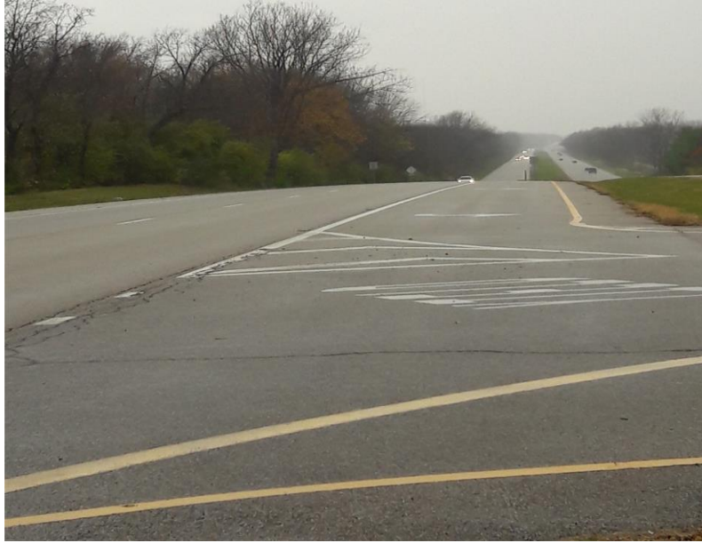
Figure E-109. Example of vehicle occlusion near the intersection of Illinois Rte. 29 and Taft Dr.
