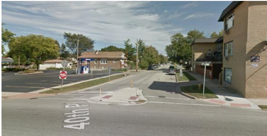
Figure E-82. Median refugee island at the intersection of IL 43 and 40 th Pl.
