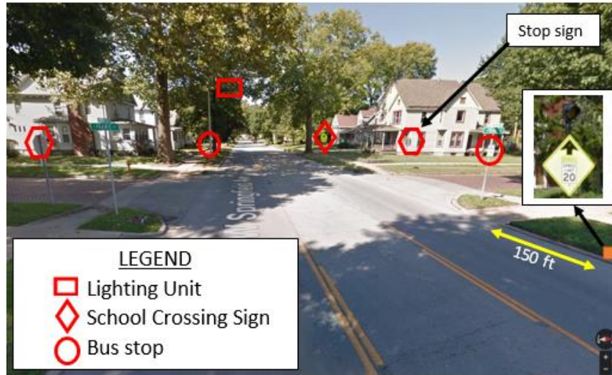
Figure E-45. Unmarked crosswalk with school crossing signs at the intersection of Springfield Ave. and S. Prairie St.
