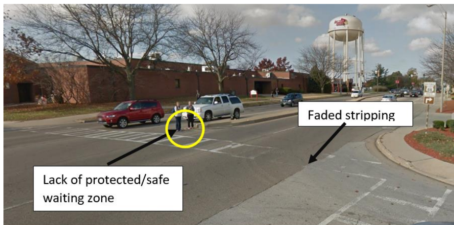
Figure E-33. Faded marking and lack of refuge island at US Business 51 and W. Locust St.
