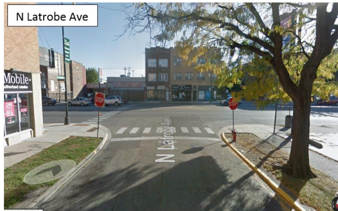
Figure E-76. Example of stop controlled marked crosswalk at the intersection of W. North Ave. and N. Latrobe Ave.
