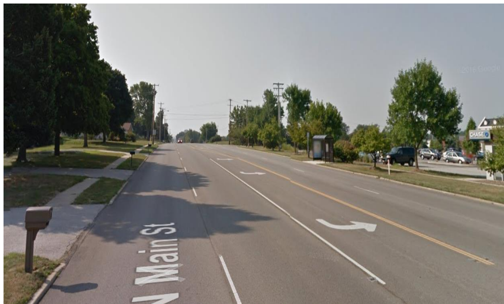
Figure E-26. Typical view of US Business 51, Main St.
