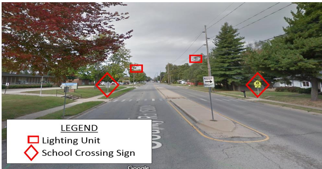
Figure E-41. Existing pedestrian treatment at intersection of Kirby Ave. and Cambridge Dr.
