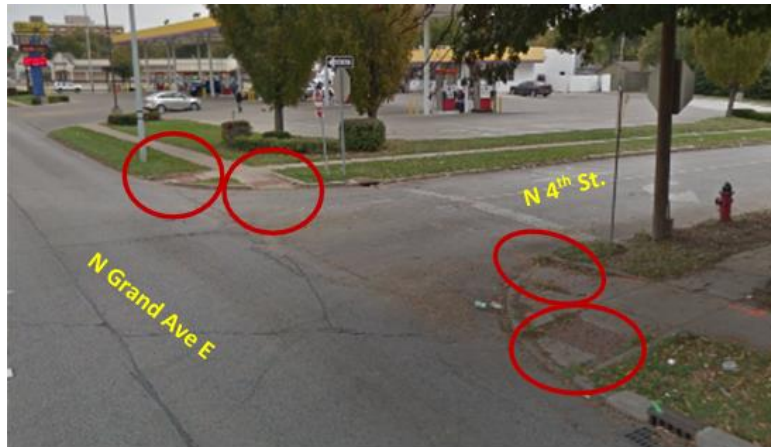
Figure E-94. Sidewalk with curb ramps but no marked crosswalks at the intersection of N. Grand Ave. and N. 4th St.
