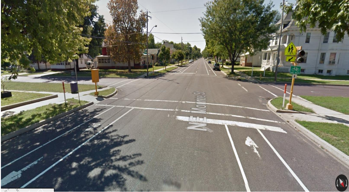
Figure E-2. Marked crosswalk with warning sign and pedestrian actuated flashing beacon.
