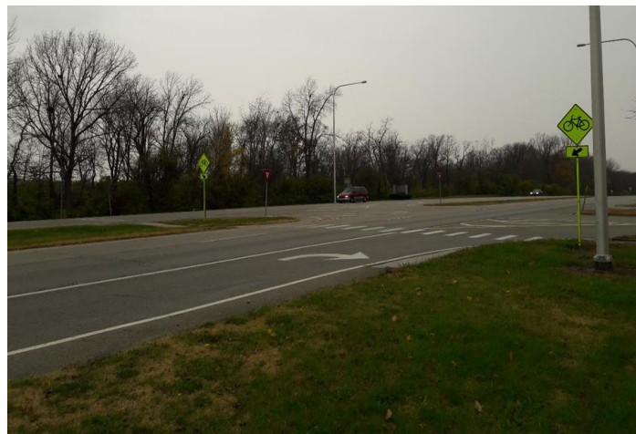
Figure 45. Example of retroreflective signposts, IL Rte. 29, Rochester, Illinois.
