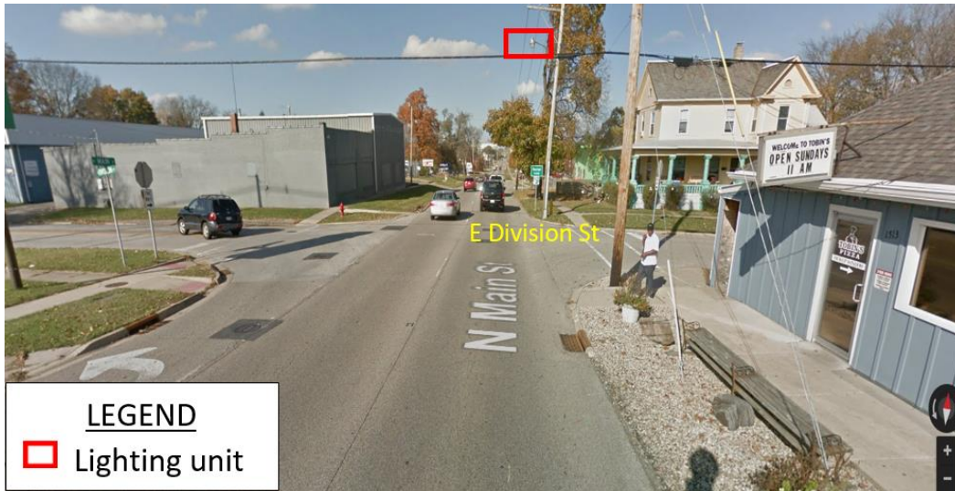
Figure E-32. Unmarked crosswalk with stop control on minor-street.
