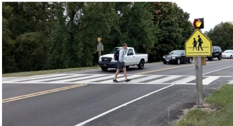
Figure 39. Example of a marked crosswalk with a flashing beacon, Edwardsville, Illinois.
