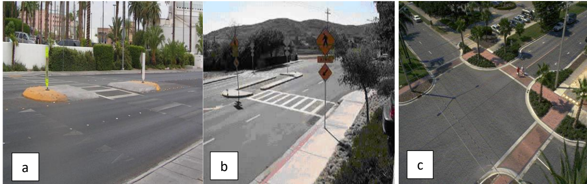
Figure 51. (a) Raised median (Pulugurtha et al. 2012); (b) split pedestrian crossover (VDOT, 2004); and (c) curb extension (Turner and Carlson, 2000).
