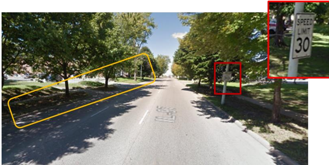
Figure E-100. Trees cover speed limit sign and crosswalk at W. Jefferson St., residential area.
