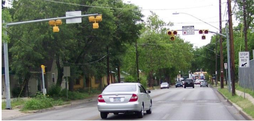
Figure 55. Example of a PHB treatment in Arizona (Fitzpatrick et al. 2014(a)).
