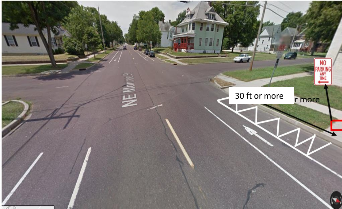
Figure E-6. Parking prohibition close to crosswalk.
