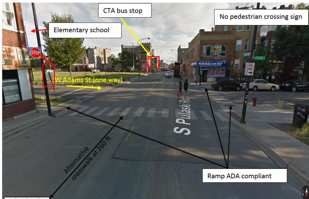
Figure E-64. Existing stop control on minor street-without median at the intersection of S. Pulaski Rd. and W. Adams St.
