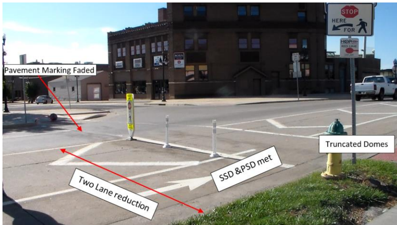
Figure E-11. Newly deployed treatment at the intersection of SW Jefferson St. with Walnut St.
