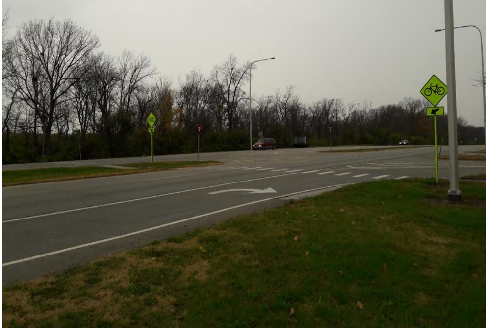
Figure A-13. Retroreflective signpost along IL 29, Rochester, IL.
