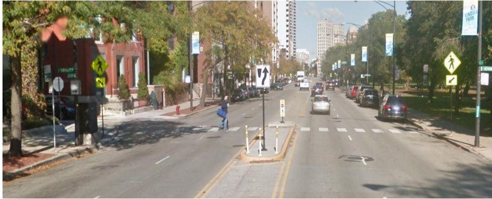
Figure 38. Example of marked crosswalk with pedestrian-refuge island, warning signs, and in-street crossing sign.
