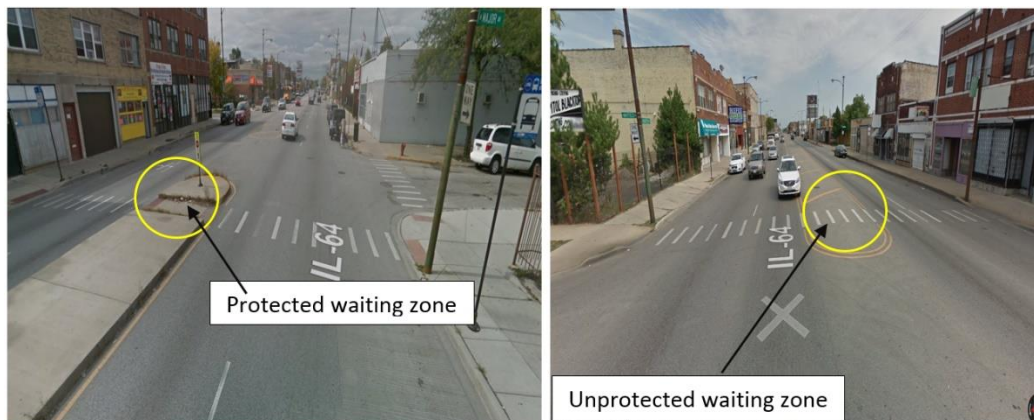
Figure E-78. Protected and unprotected waiting area along W. North Ave.
