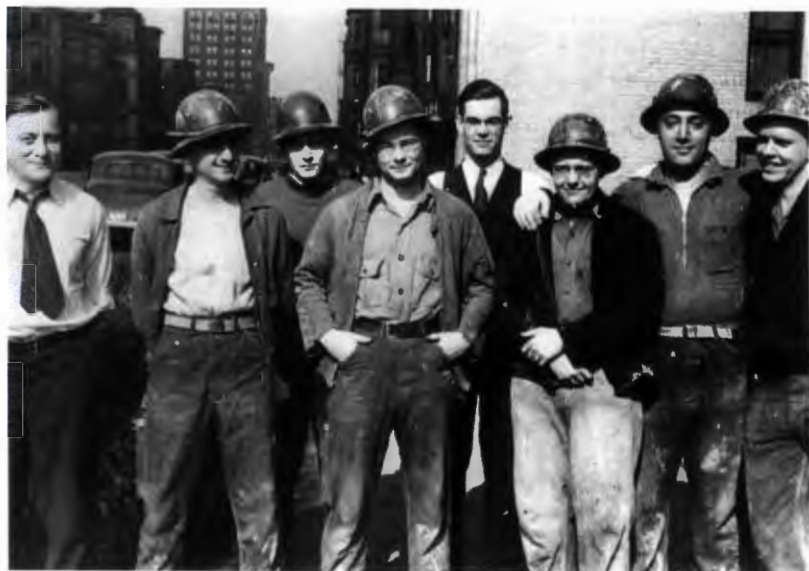
Archival photo taken during the construction of the Chicago subway. Chester P. Siess, faculty member and department head from 1973-1978 is second from left. Ralph Peck, who served on the department faculty from 1942-1974, is fifth from left.
