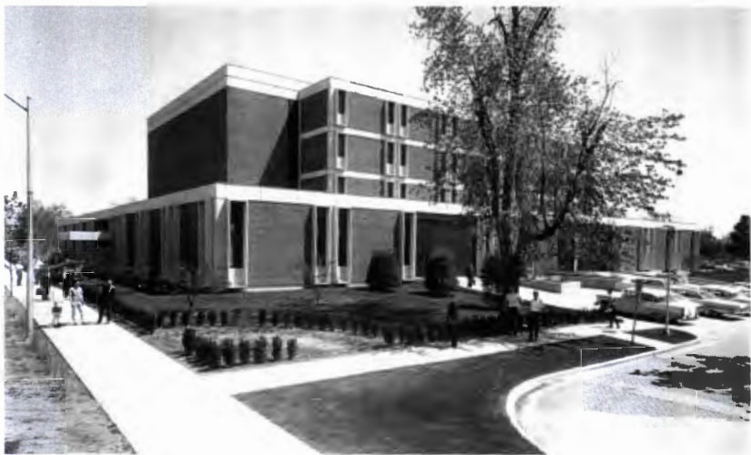
The early days of the Civil Engineering Building, later Nathan M. Newmark Civil Engineering Laboratory, shown here from the south, circa 1967.
