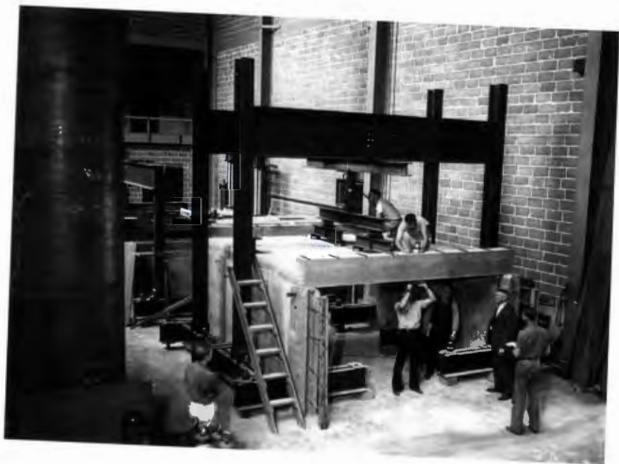
One of the structural research programs of this era was what came to be known within the department as "The Slab Project." The objective of the 10-year project was to improve our understanding of the behavior of reinforced concrete slabs and improve our ability to design and build them. Much of the theory developed is still in use today. Photo courtesy of the University of Illinois archives. (Image 0005372, Bridge Slab Investigation, circa 1939)
