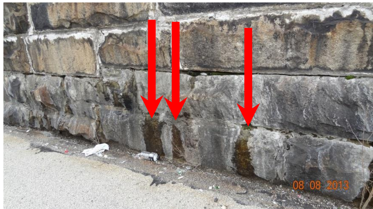
Figure 3.59: Water seeping from (a) masonry abutment wall under Upland Avenue Bridge and (b) north-south trending masonry wall north of Upland Avenue Bridge on 8 August 2013.
