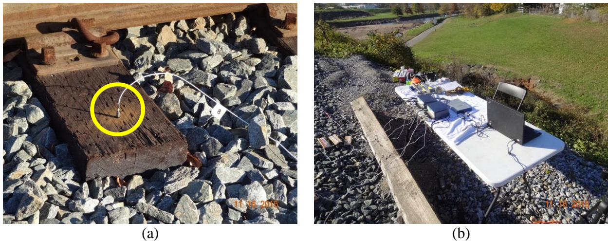
Figure 4.4: Photographs of (a) an accelerometer attached to a timber tie, and (b) the roadside accelerometer setup including signal conditioners, DAQ, and laptop.
