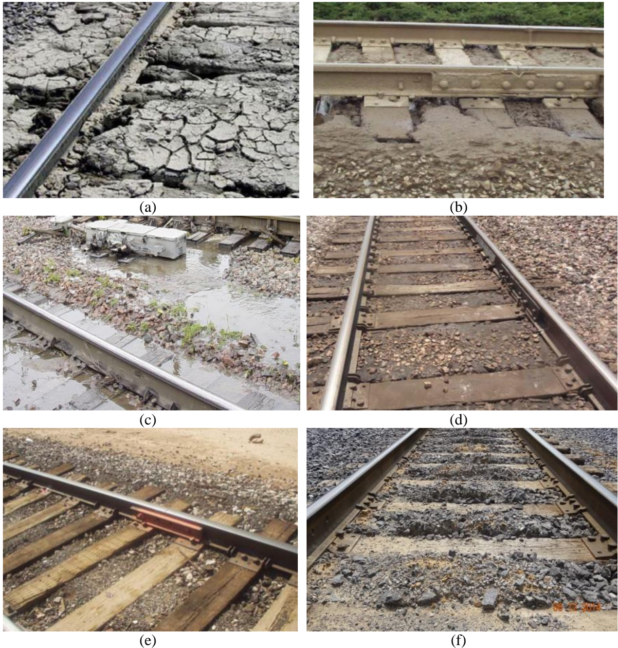
Figure 2.9: Photographs of track with various fouling levels (a,e photos courtesy of David Jamieson).
