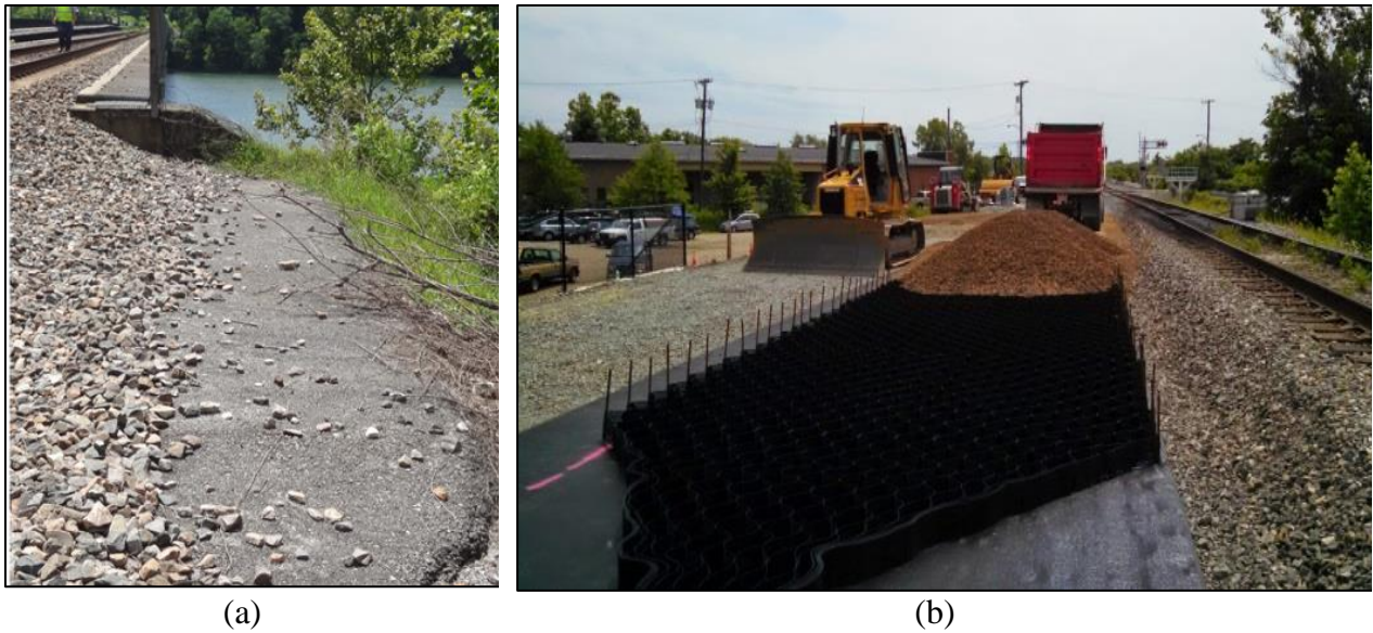
Figure 6.13: Photographs of (a) HMA and (b) geoweb underlayment.
