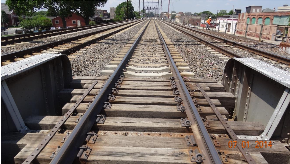
Figure 3.1: Photograph on Upland Avenue Bridge on Track #2.
