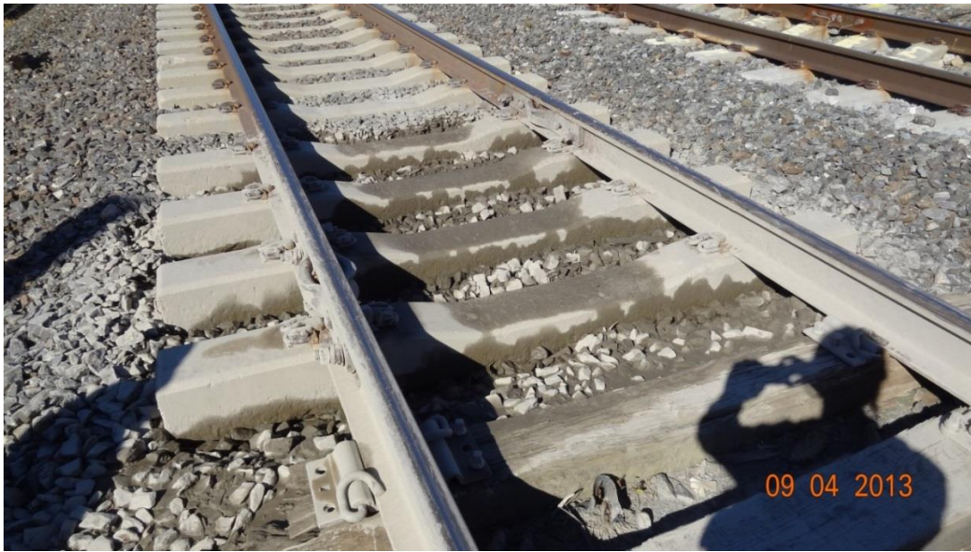
Figure 3.58: Fouling material covering ballast and concrete ties on Track #1 at Madison (12 ft) on 4 September 2013.
