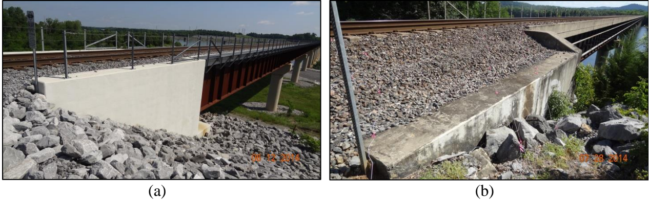
Figure 6.12: Photographs of concrete wing walls.
