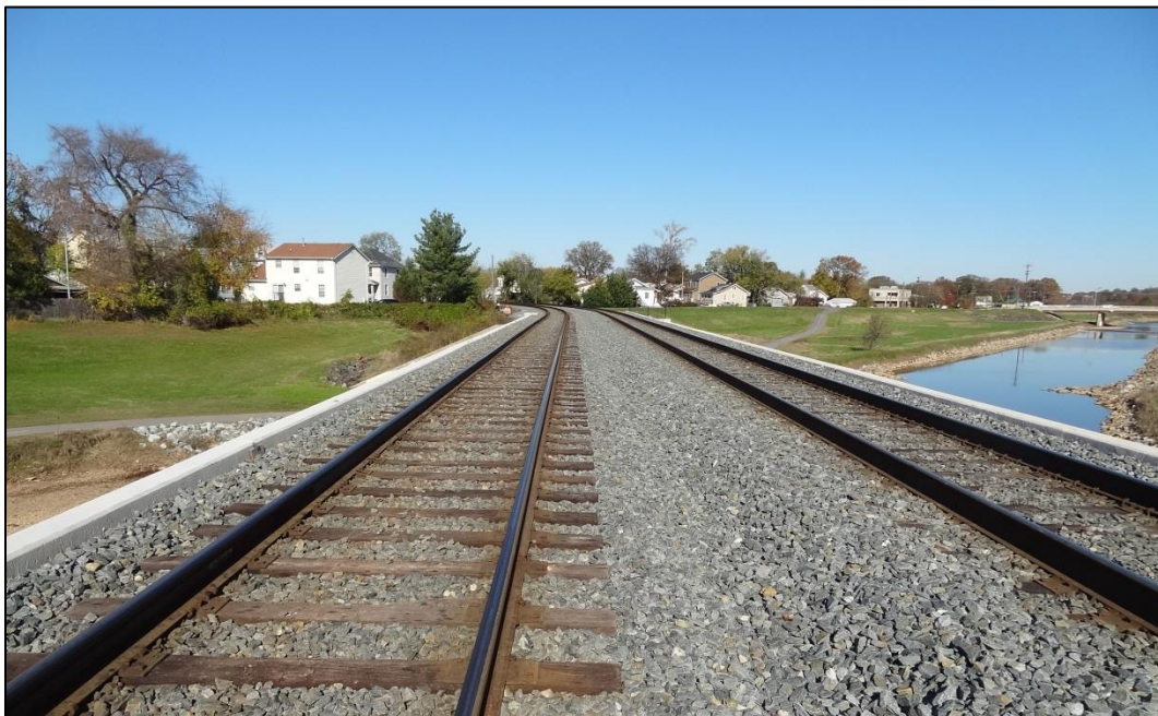
Figure 6.10: Photograph of ballasted-deck bridge.
