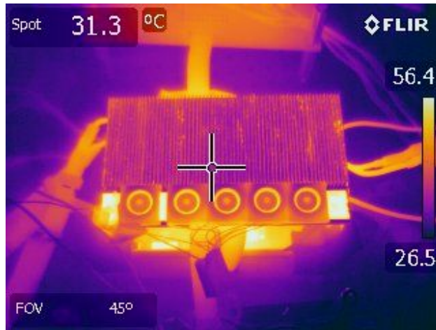
Figure 6.21: Thermal image of the inverter operating at full power (2 kW). The maximum temperature is 57 °C.
