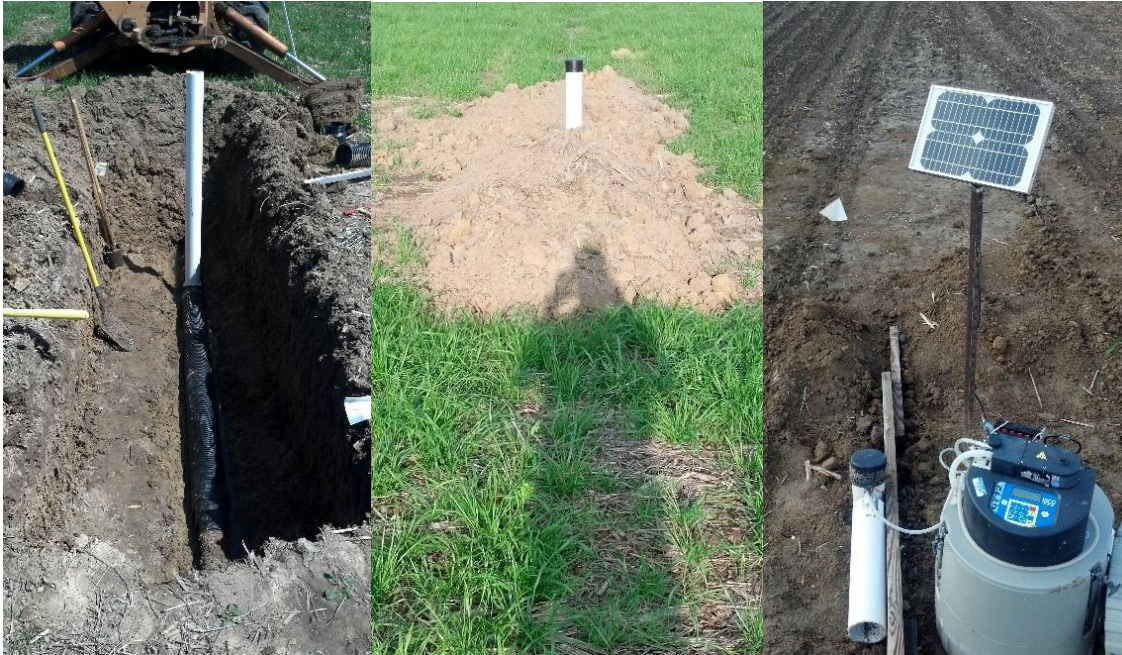
Figure 6. The replacement of tile with flow monitoring station and complete setup.
