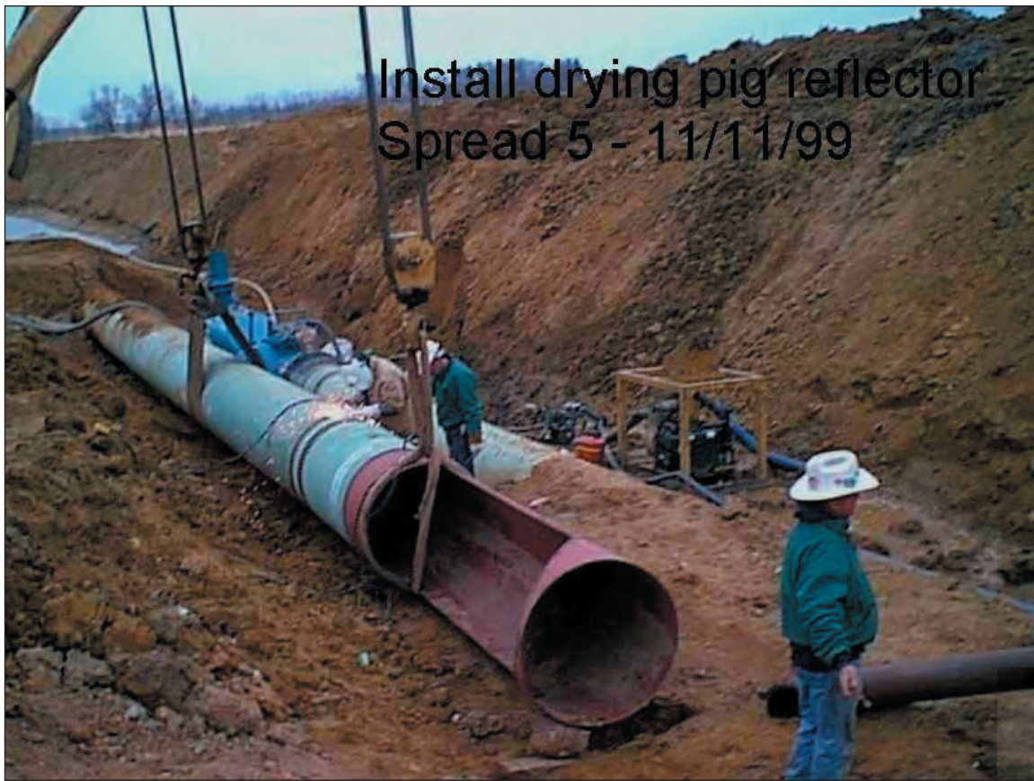
Figure C1.38. Drying pig deflector being installed after test/dewater header has been removed
