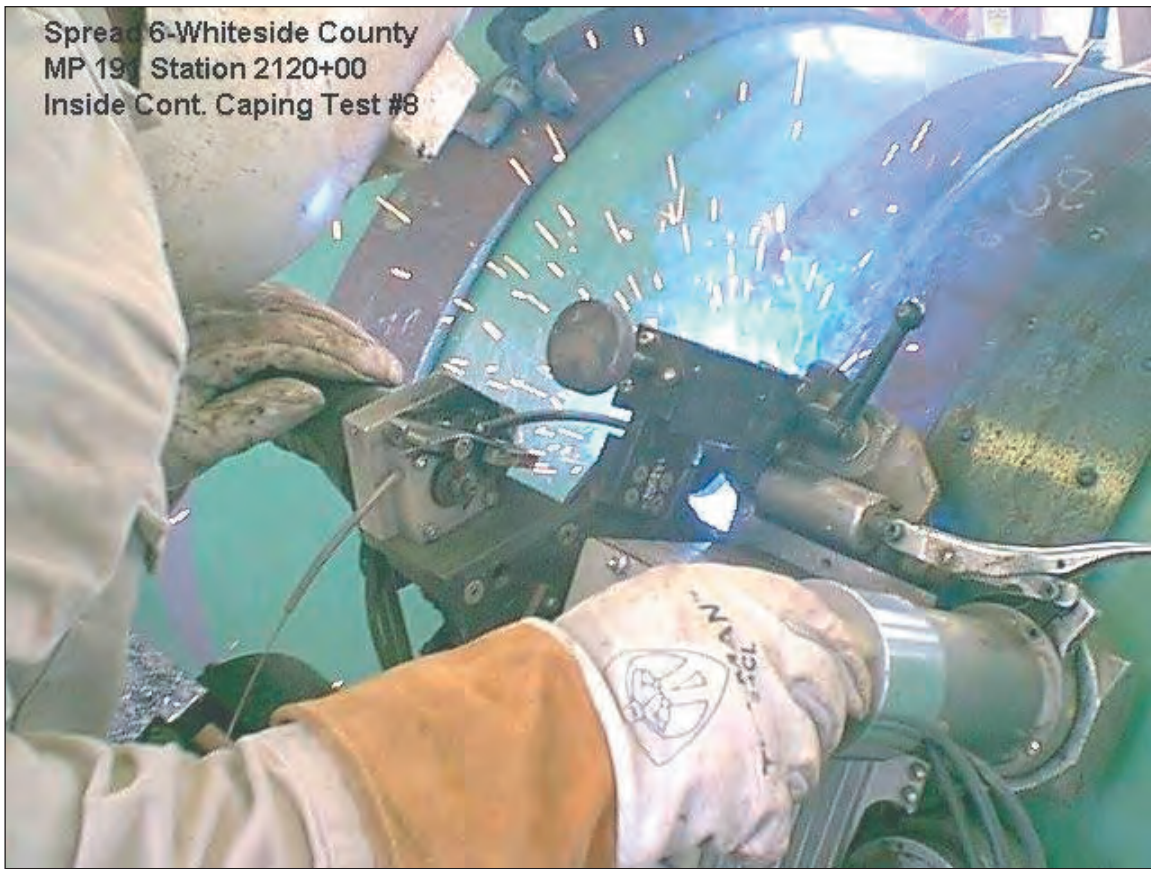
Figure C1.23. Mechanized welding, large-diameter high-pressure pipeline
