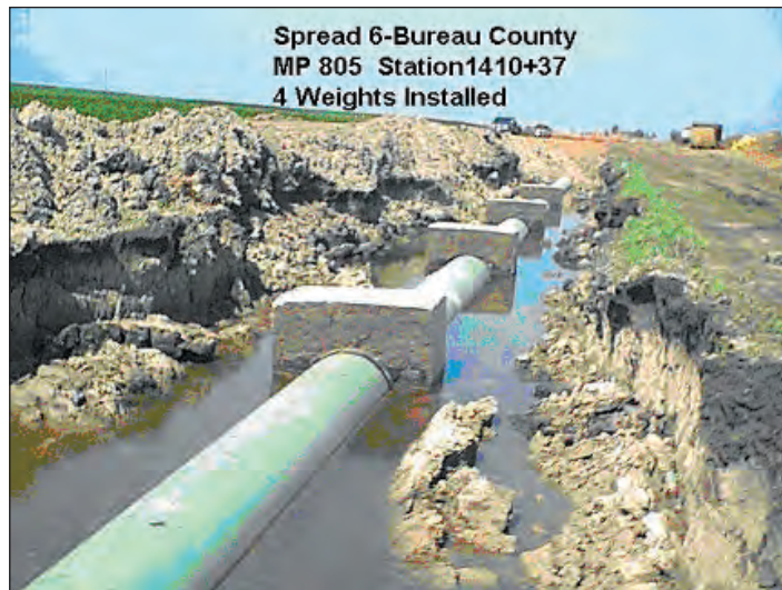
Figure 6.7. Set-on weights in a low areas where sand subsoil layer is on top of a deep layer of clay subsoil
