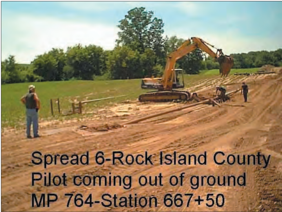
Figure C1.12. Horizontal directional drilling pilot coming out
