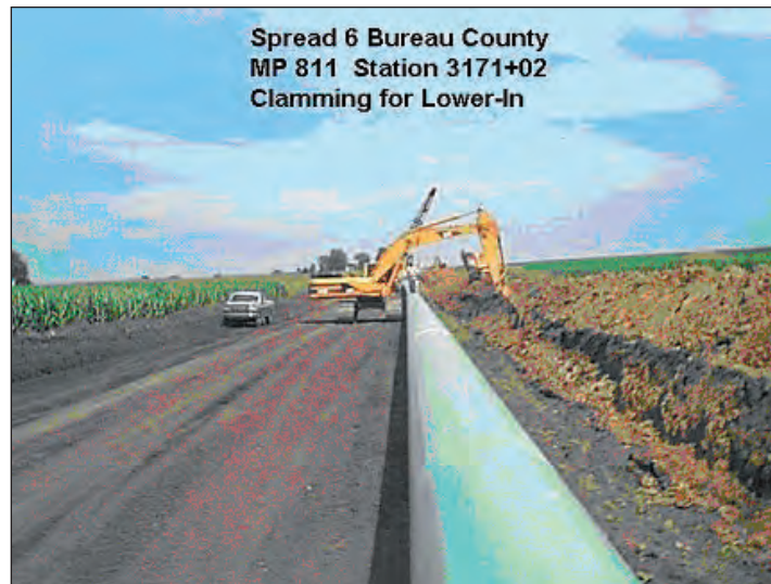
Figure 6.5. Backhoe reaches over pipe to clam out ditch
