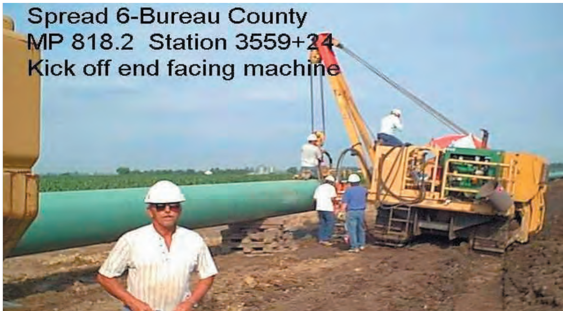
Figure C1.19. End facing to ensure the highest weld quality
