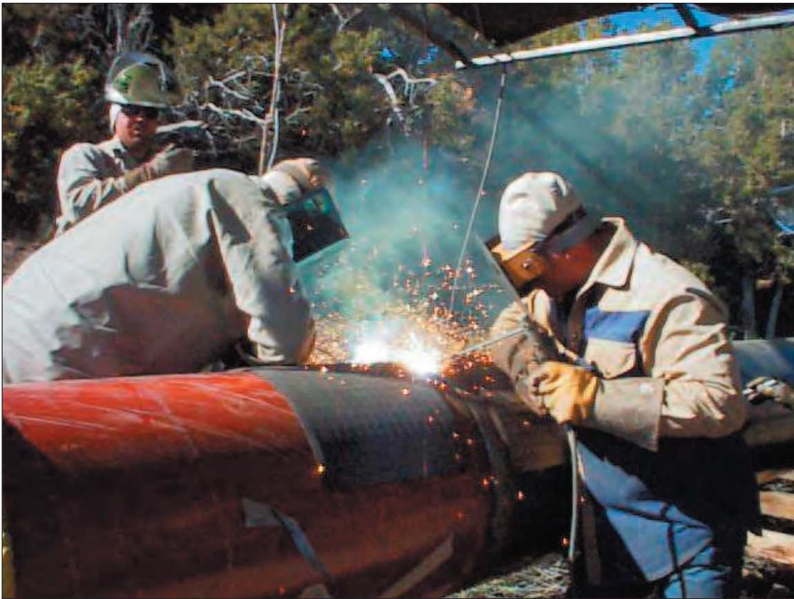
Figure C1.22. Manual welding from both sides (12 o'clock to 6 o'clock)
