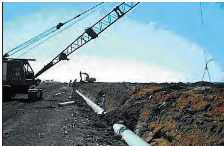
Figure 6.6. Crane plugs pipe during backfill operations
