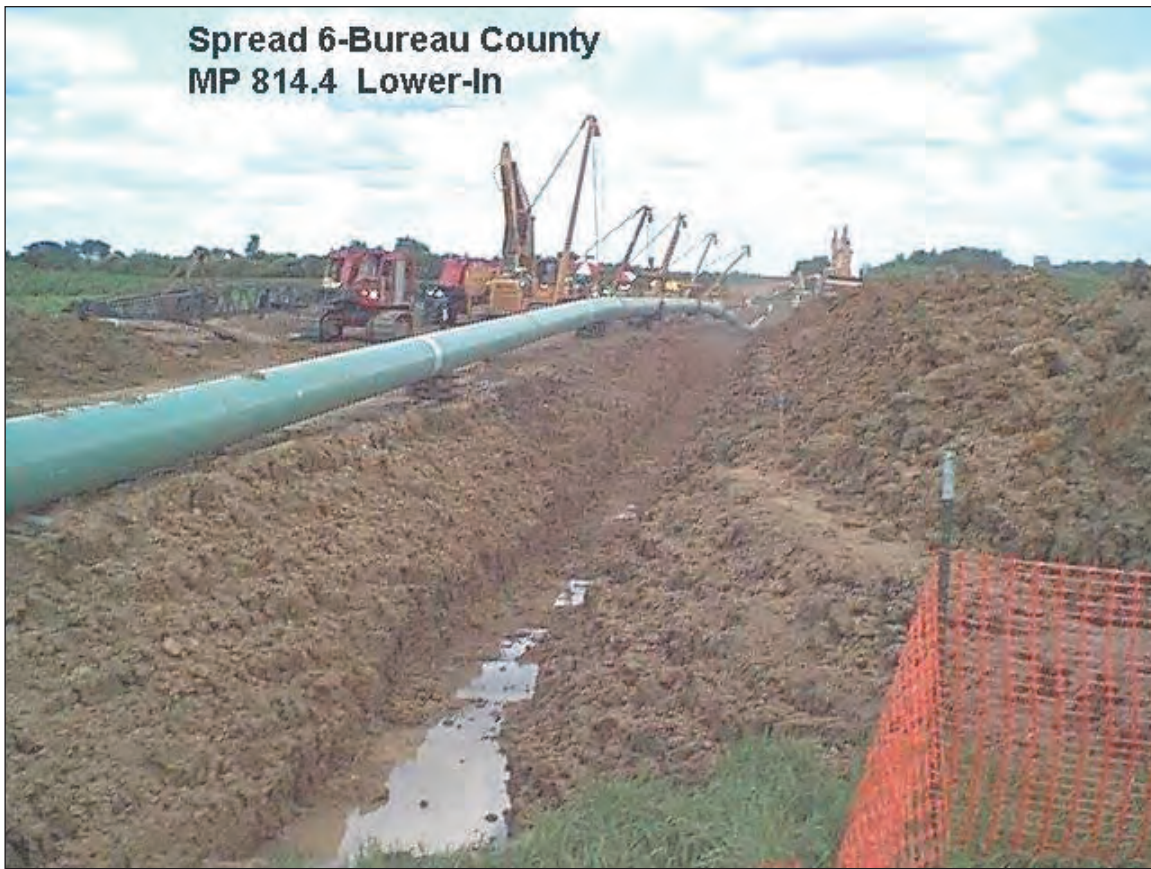
Figure C1.27. Lower-in tractors in various boom positions
