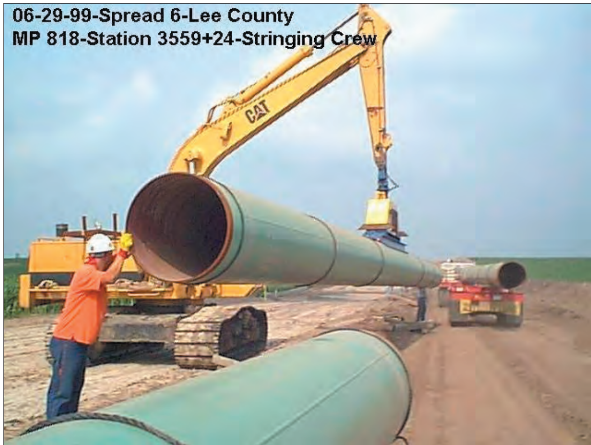
Figure C1.7. Setting pipe from the string truck on skids
