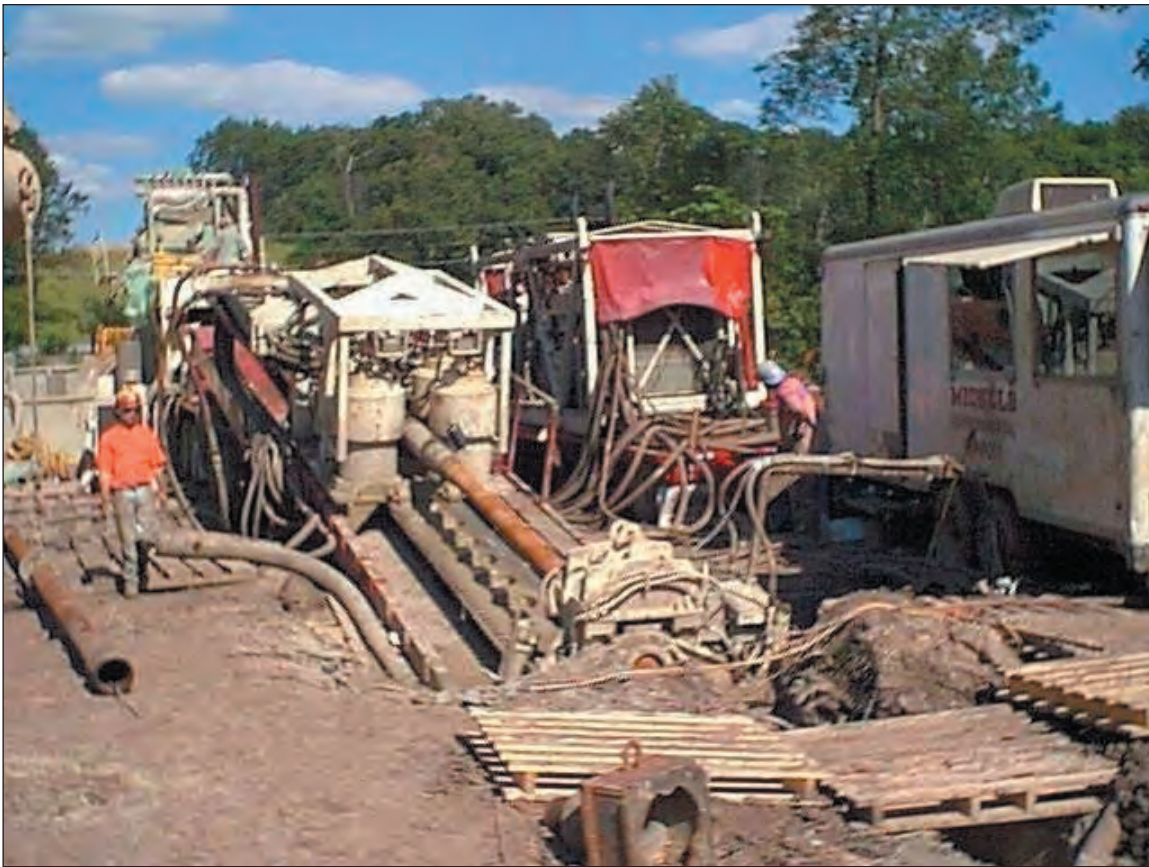
Figure C1.11. Horizontal directional drill site
