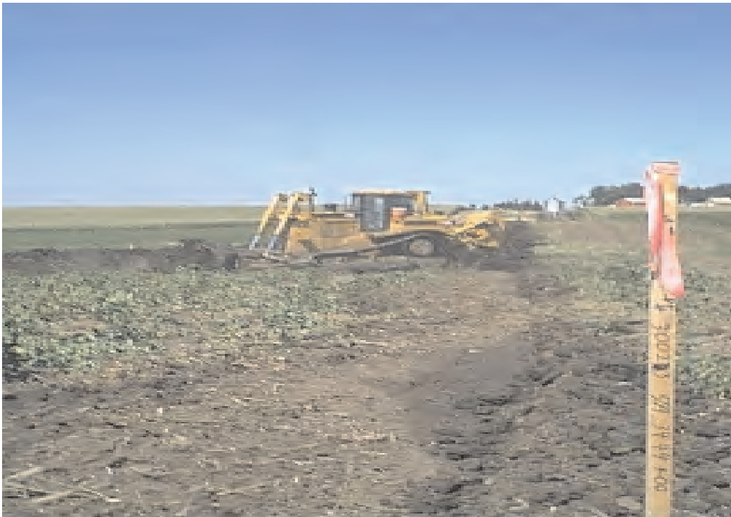
Figure C1.4. Topsoil stockpiling progress
