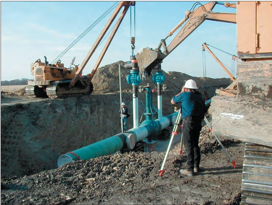
Figure C1.32. Prefabricated mainline valve being installed in rock ditch
