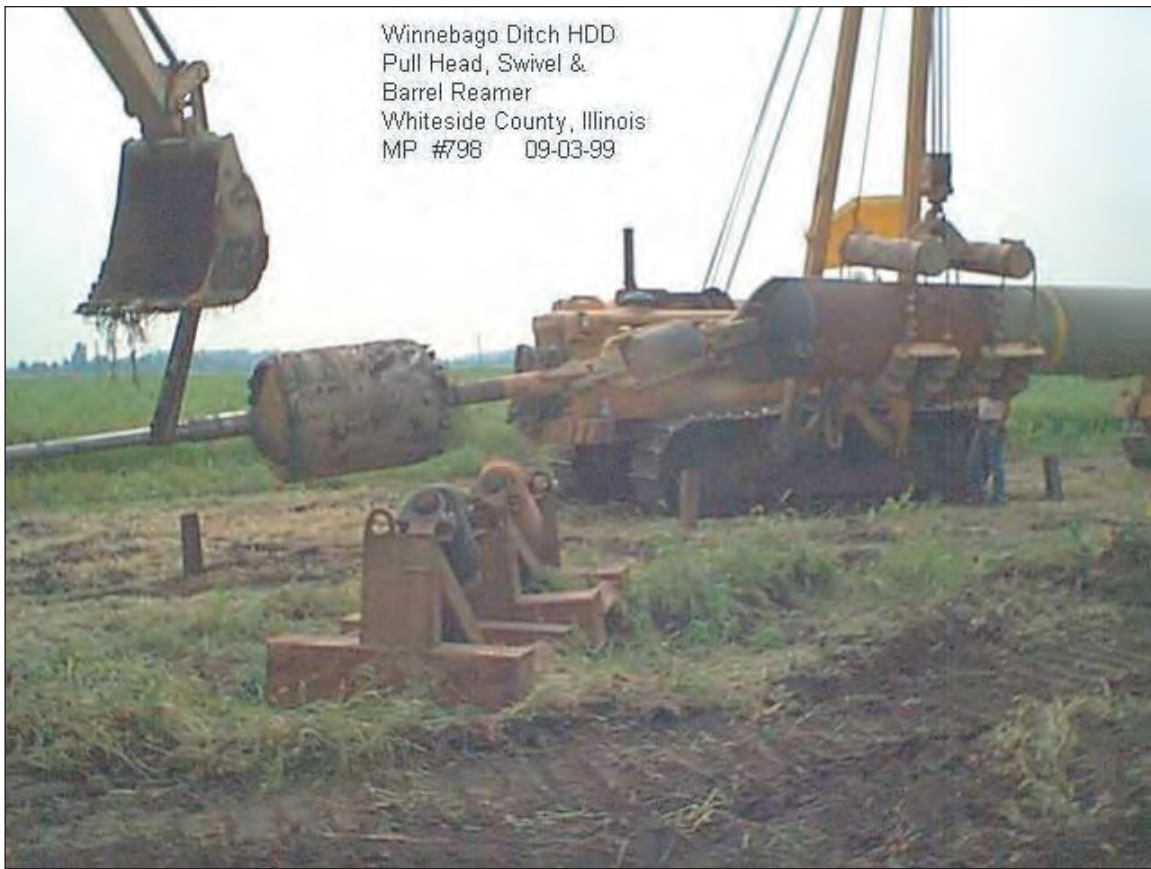
Figure C1.14. Horizontal directional drilling—ready to pull the prewelded pipe
