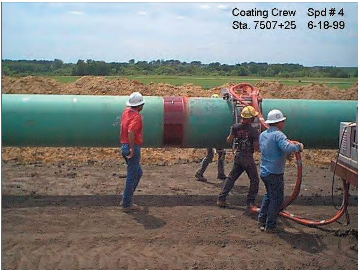
Figure C1.24. Coating using fusion bond epoxy
