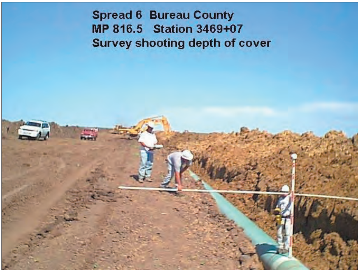
Figure C1.29. Surveying weld location and cover
