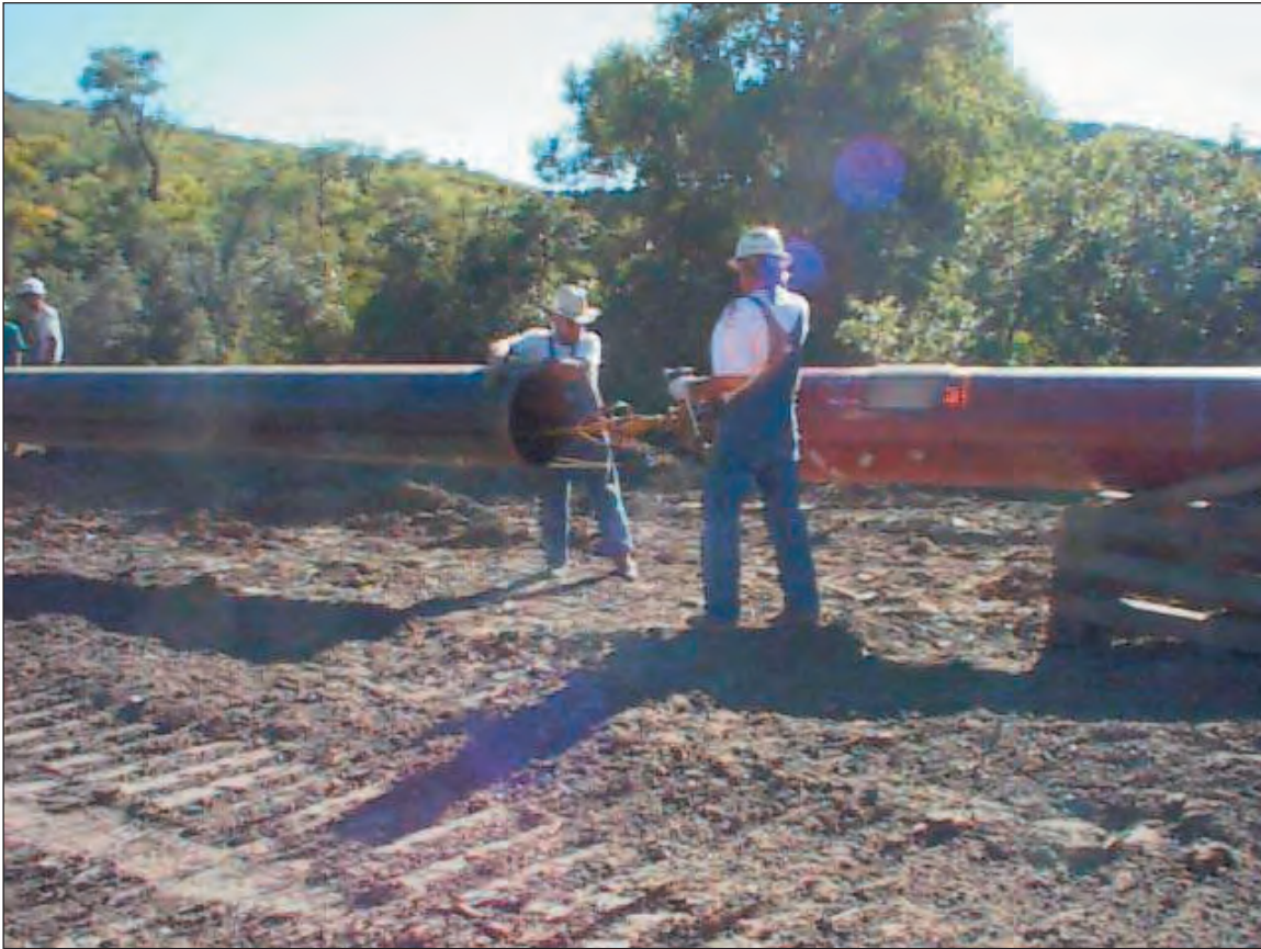
Figure C1.21. Pipe joint being stabbed over internal lineup
