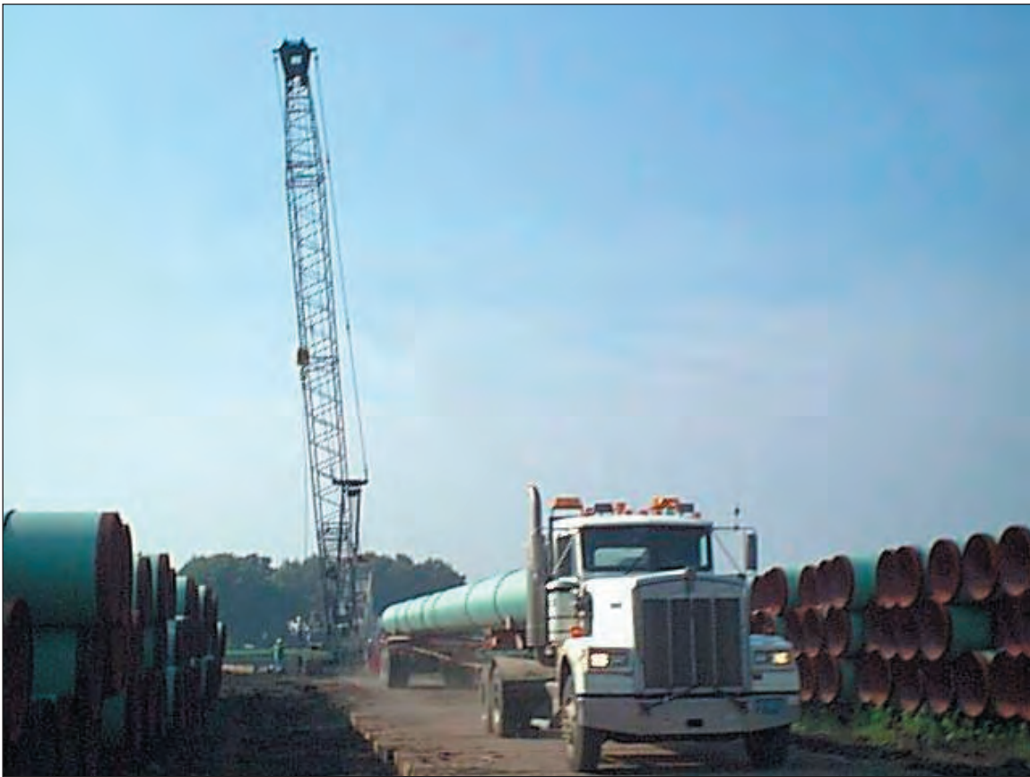
Figure C1.6. Stringing from the pipe yard
