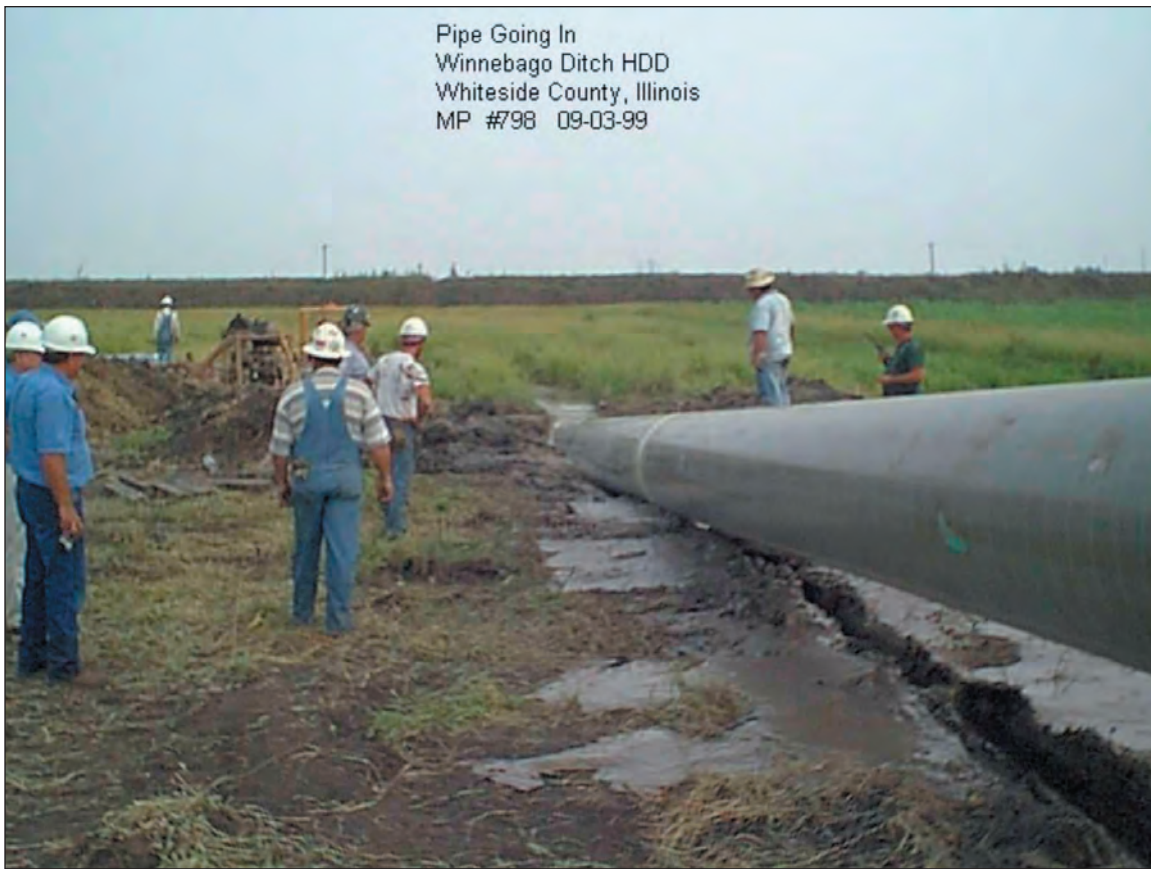
Figure C1.16. Pipe going in under levee canal
