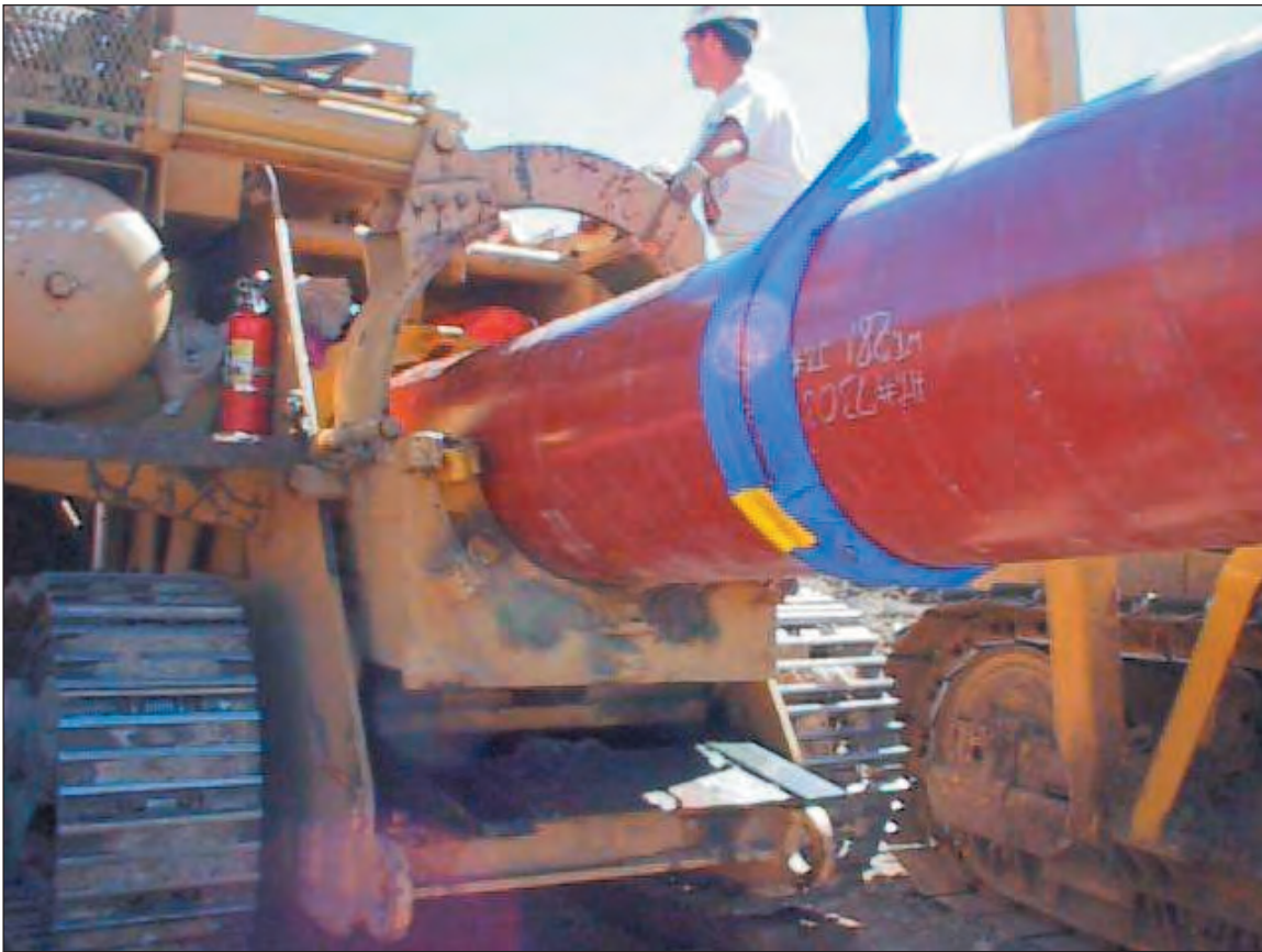
Figure C1.9. Pipe lifted into bending machine mandrel
