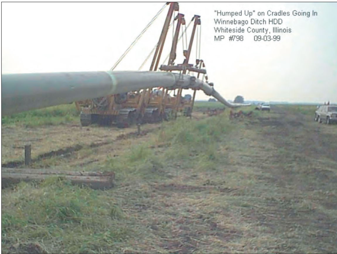
Figure C1.15. Pulling operations under way
