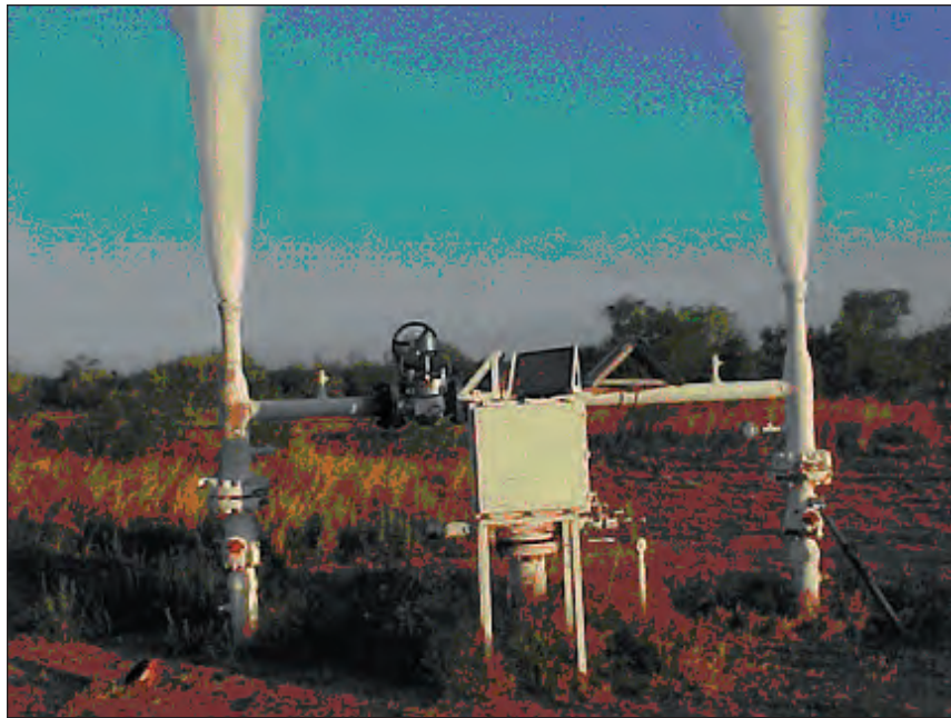
Figure 6.2. CO 2 venting during pipeline purging
