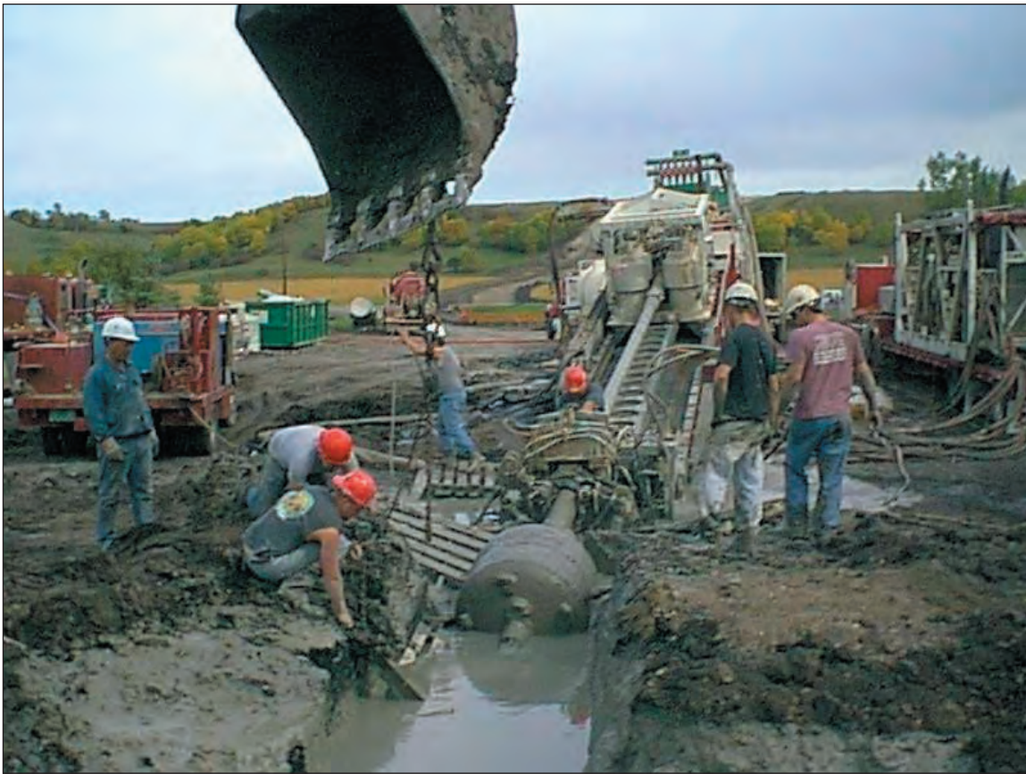
Figure C1.13. Horizontal directional drilling barrel reamer coming out
