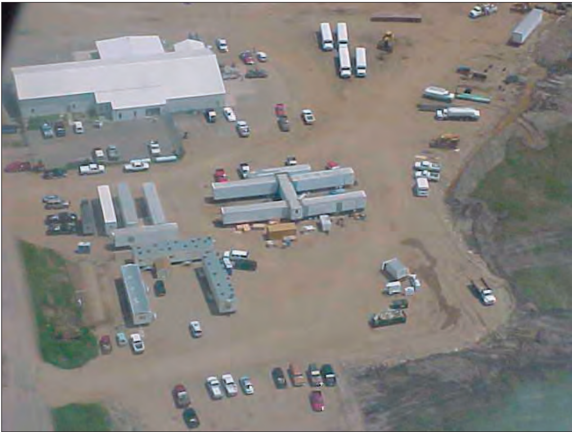
Figure C1.2. Spread construction yard
