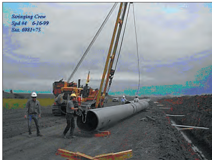
Figure 6.8. String crew working over existing drain tiles where temporary drain tiles (white segments) are in place
