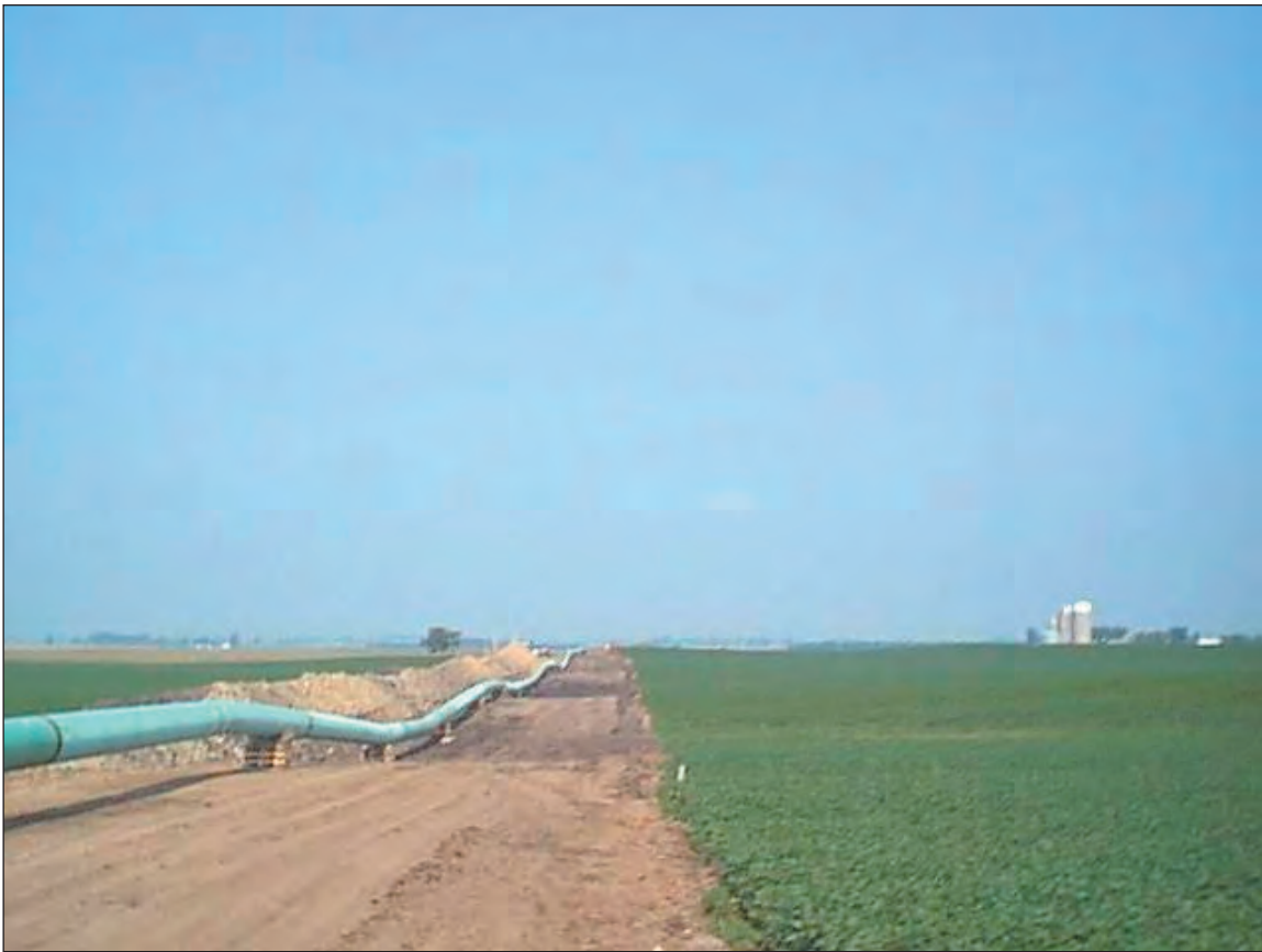
Figure C1.26. Pipe welded, coated, and ready to be lowered in
