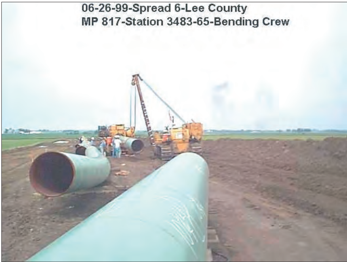
Figure C1.8. Pipe bent to accommodate direction change
