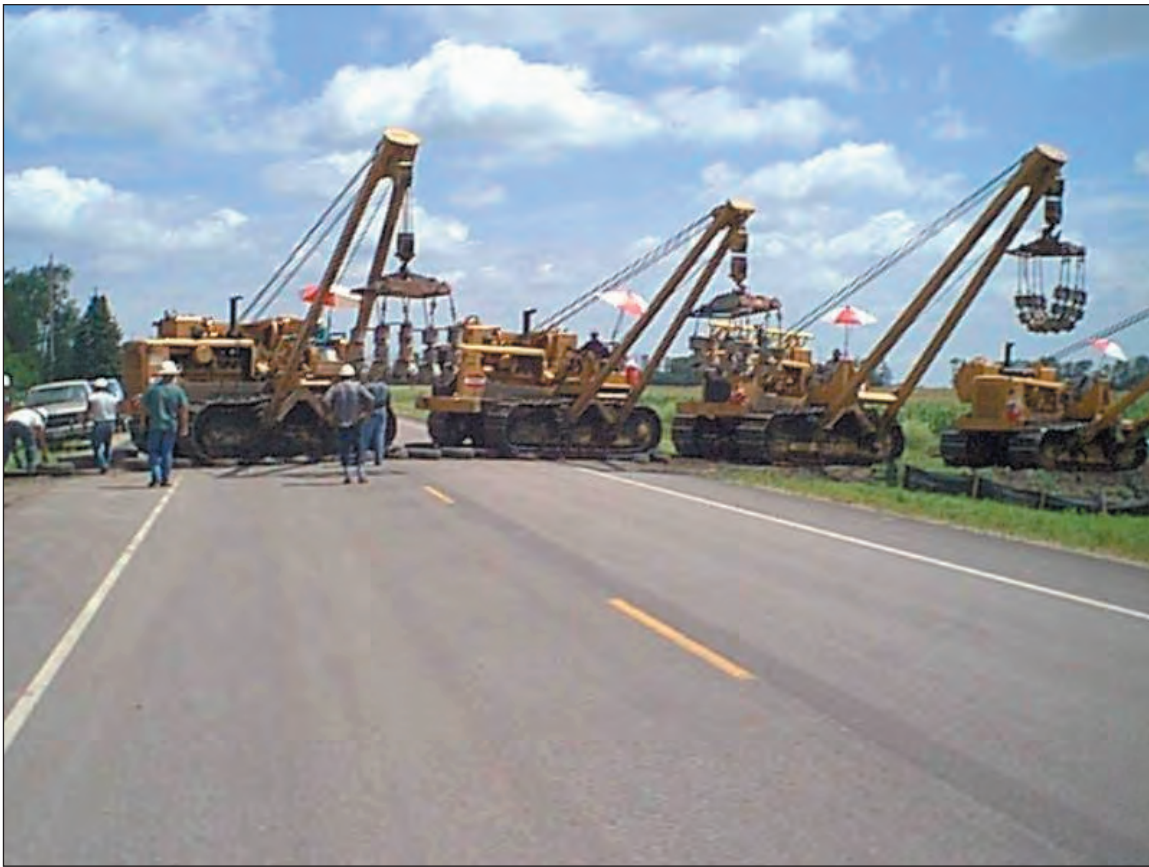
Figure C1.28. Lower-in crew making a road crossing
