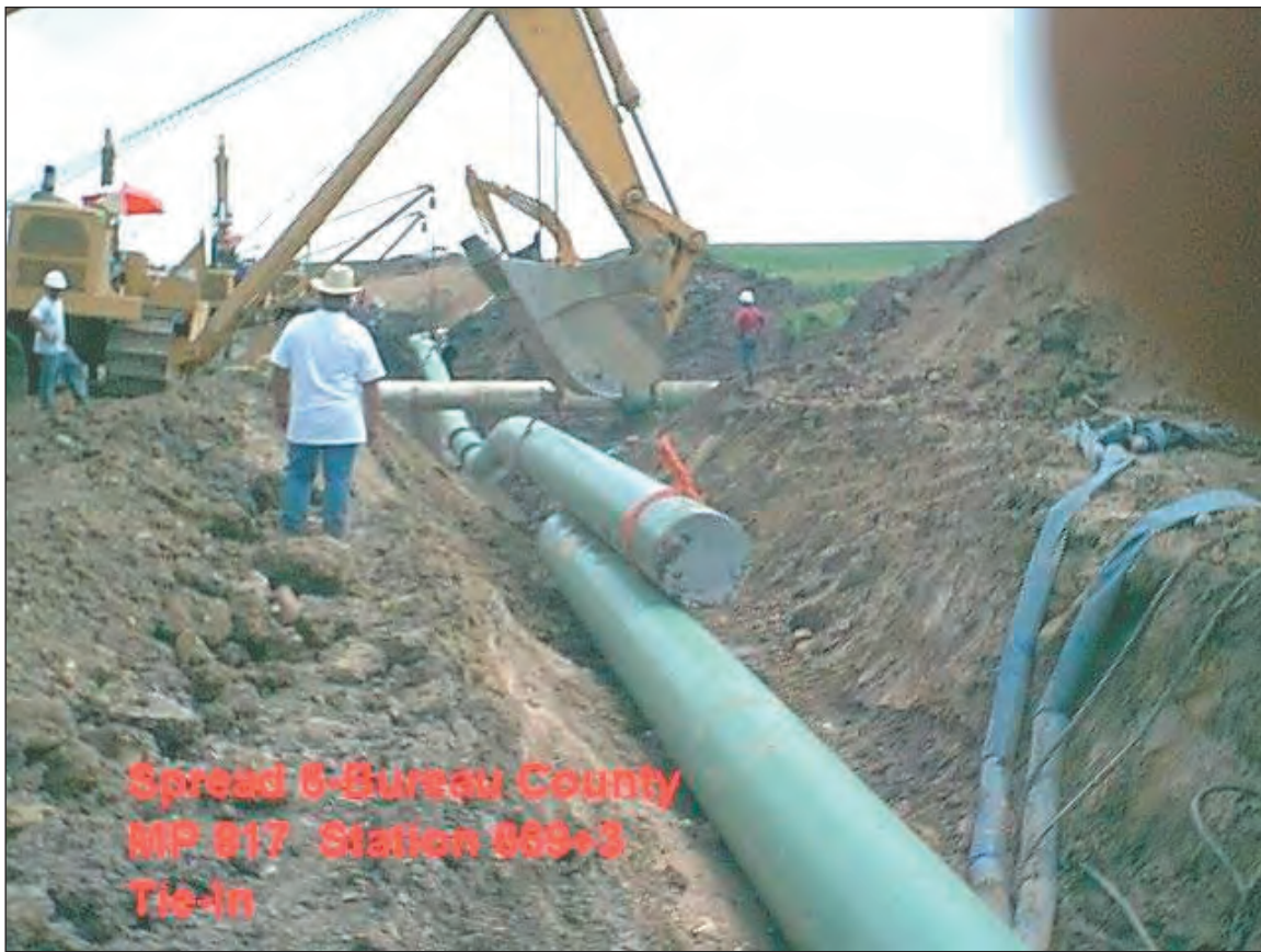
Figure C1.34. Tie-ins: Sag and overbend section set in place
