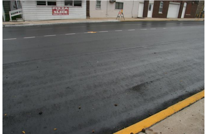
Figure 37. Prime coat on level binder looking west near Sta. 81+00.
