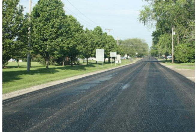
Figure 11. Segment 2 (Peale to US 30) cold-milled pavement looking west.
