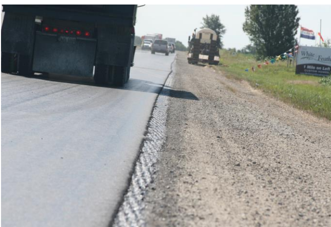
Figure 24. Level binder with 12 in. exposed milled pavement.
