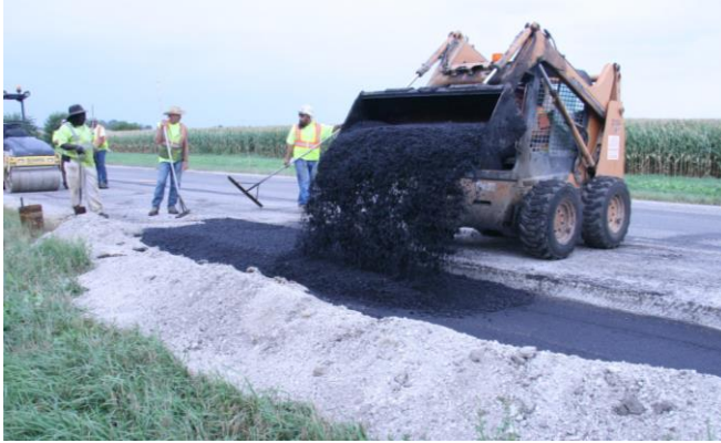
Figure 32. US 52 patching near Sta. 36+00 in eastbound (southbound) lane.
