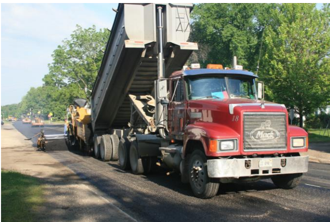
Figure 14. Segment 2 (Peale to US 30). Placing 4.75 mm level course.
