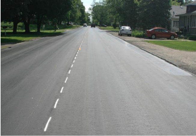
Figure 16. Segment 2 (Peale to US 30). Typical tack coat on level binder.
