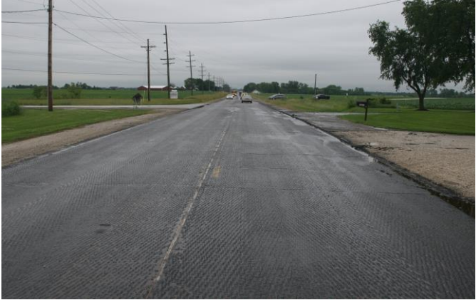
Figure 20. Primed cold-milled surface of US 52 near Sta. 47+00 looking south.
