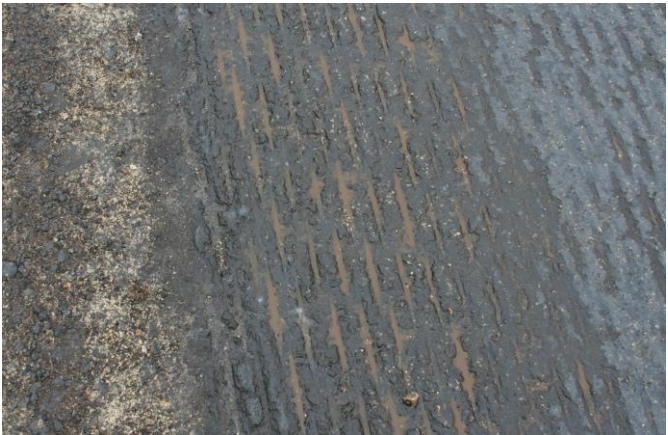
Figure 22. Brown “unbroken” emulsified asphalt prime coat
