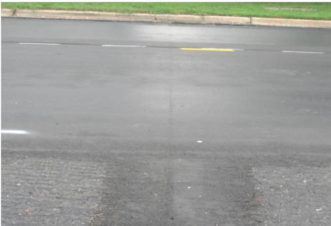
Figure 18. Segment 1 (Briggs to Peale). Reflection through level binder at Sta. 23+52.
