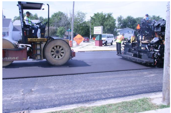
Figure 35. Rolling level binder directly behind paver in westbound lane near Sta. 84+00.
