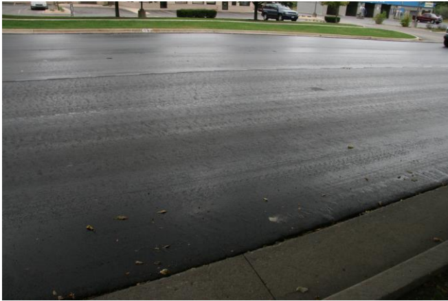
Figure 36. Prime coat on level binder looking west near Sta. 63+00.
