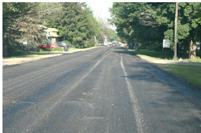
Figure 9. Segment 2 (Peale to US 30) cold-milled pavement looking west.
