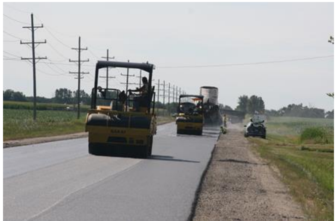
Figure 29. Paving train of surface looking south near Sta. 90+00.
