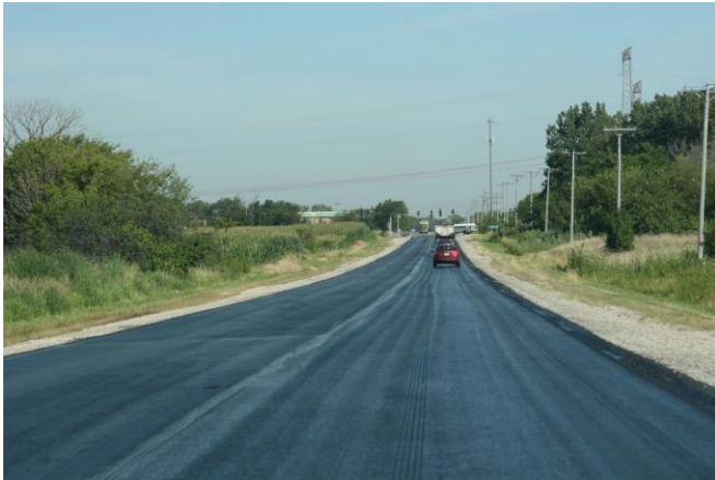
Figure 26. Prime coat on level binder looking north near Sta. 45+00.
