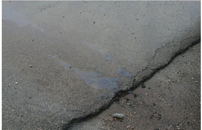
Figure 23. Asphalt prime migration to shoulder.
