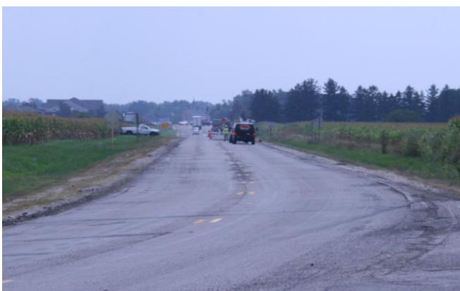
Figure 30. Cold-milled surface of US 52 near Gougar Road (to right) looking south.
