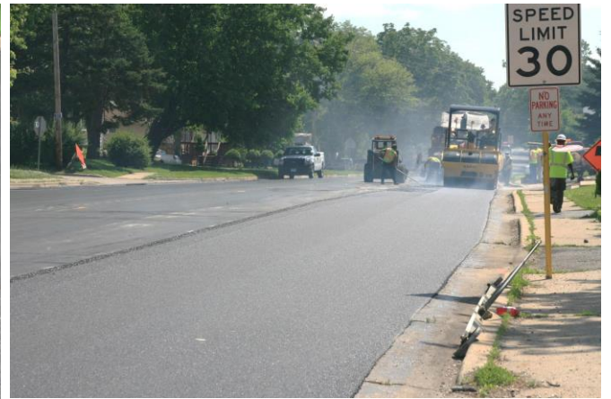
Figure 19. Segment 1 to 2 transition at Peale. Paving surface course.
