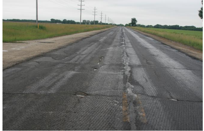
Figure 21. Prime cold-milled surface of US 52 near Sta. 114+00 looking north.
