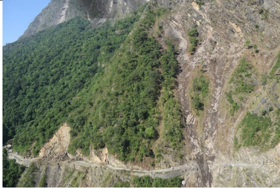
Figure 2.9 Landslides observed along the road alignment constructed along steep terrain.
