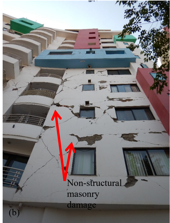
Figure 3.38 Swayambhu Apartment Complex – non-structural damage.
