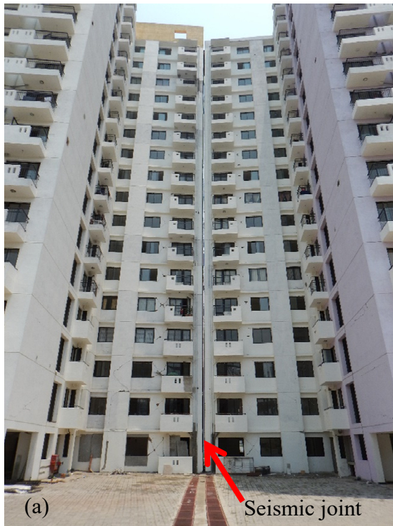
Figure 3.36 Sun City Apartment Complex – representative seismic joint: (a) overall view; (b) detail.
