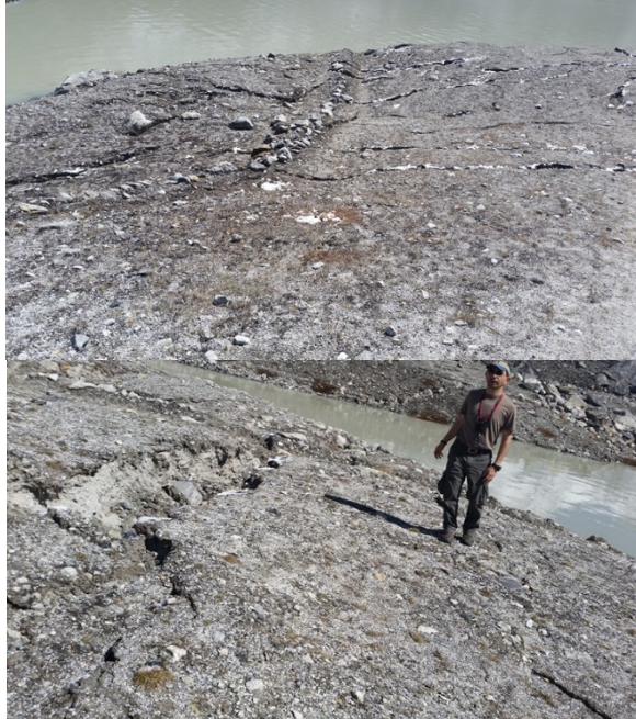
Figure 2.21 Lateral Spreading along the upstream side of the spillway (27°52'9.57"N, 86°27'44"E) (after Hashash et al. 2015).
