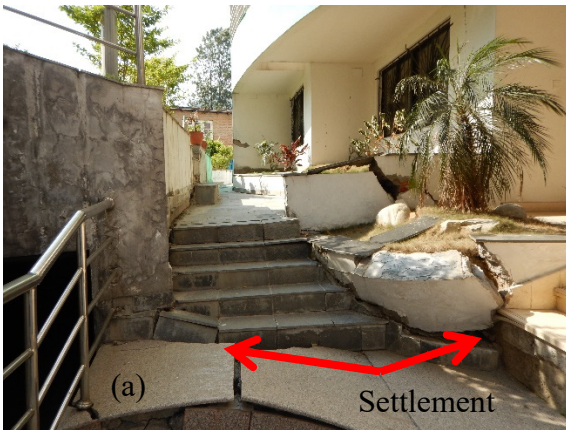
Figure 3.39 Swayambhu Apartment Complex – backfill settlement.
