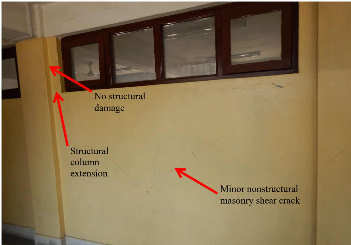
Figure 3.22 Kathmandu Engineering College Block E Building – interior view.
