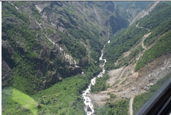
Figure 2.11 Landslide near the dam site of the hydropower project that damaged the road.
