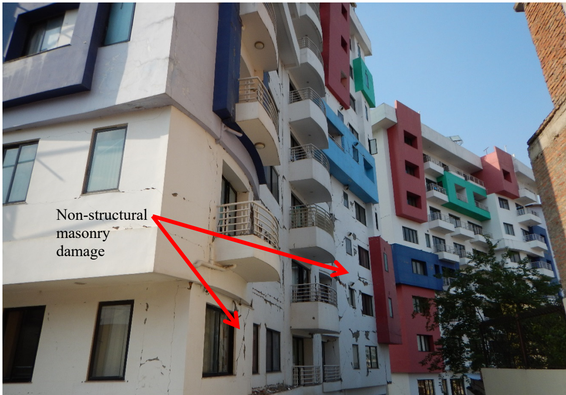
Figure 3.37 Swayambhu Apartment Complex.
