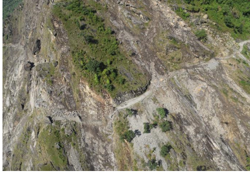
Figure 2.7 Charikot-Lamabagar road sector affected by landslides triggered due to the earthquake .
