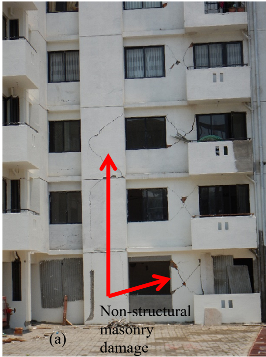
Figure 3.35 Sun City Apartment Complex – moderate non-structural damage in group of two buildings.
