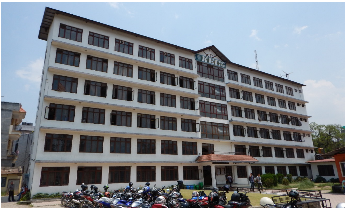
Figure 3.21 Kathmandu Engineering College Block E Building – exterior view.
