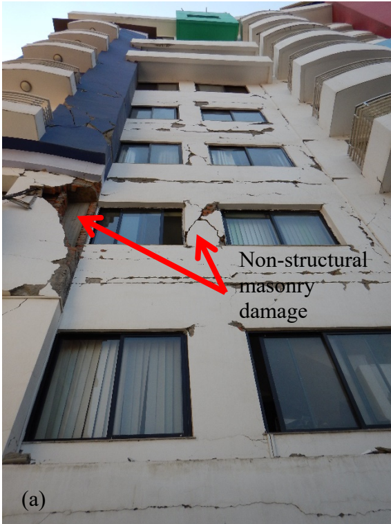
Figure 3.38 Swayambhu Apartment Complex – non-structural damage.
