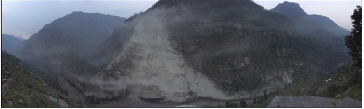
Figure 2.16 The landslide blocked the Kali Gandaki River forming approximately 2 km long and 150 m deep artificial lake (28°24'8.48"N, 83°35'47.5"E) (after Hashash et al. 2015).
