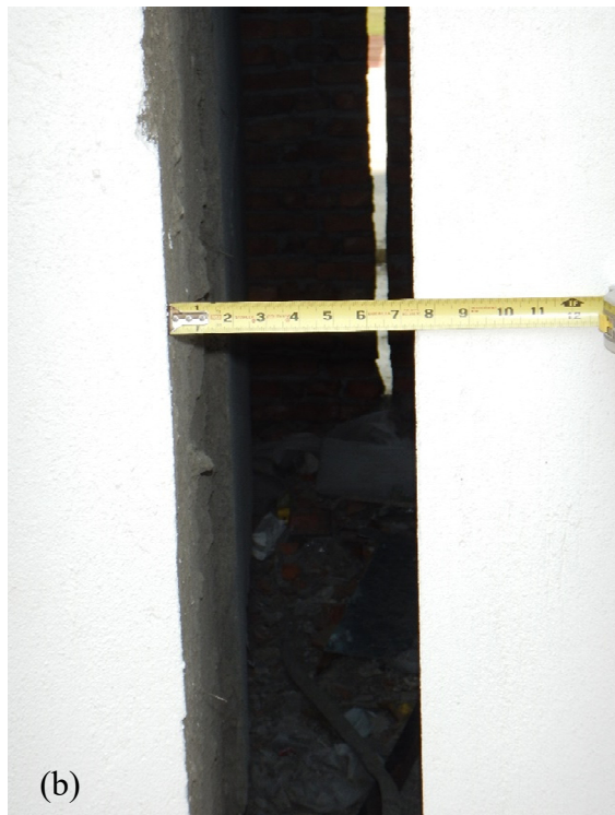
Figure 3.36 Sun City Apartment Complex – representative seismic joint: (a) overall view; (b) detail.
