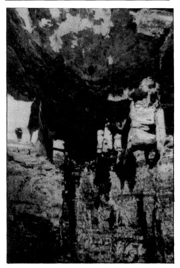
**Figure 21** Intense northeast-trending fractures along the strike-slip fault in Crown II Mine. Petroleum seeping from fractures stained the rock dust.
