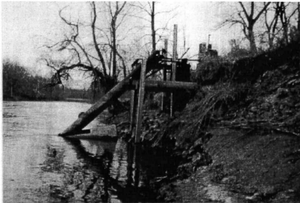
Figure 9b. An example of a rural pump station and bank erosion conditions along the Kankakee River in Indiana
