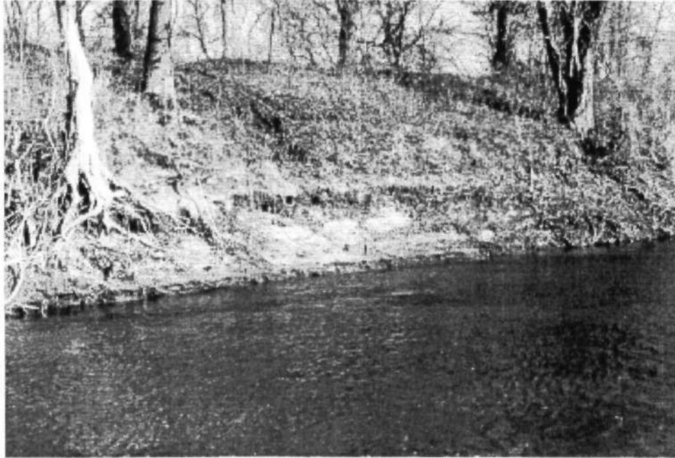
Figure 1 la. An example of exposed and undercut tree roots on a steeply sloped, sandy bank on the Kankakee River in Indiana
