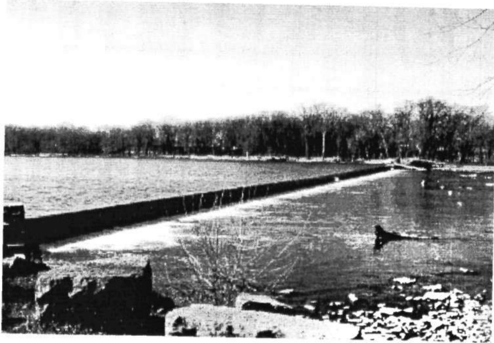
Figure 14a. A view of the Wilmington Dam on the Kankakee River in Illinois
