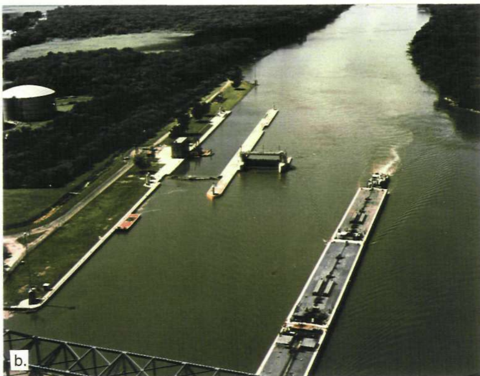
Figure 2. Aerial view of the Peoria Lock and Dam during flood stages when the wicket gates are lowered: (a) looking upstream, the lock and adjacent taintor gate are at the center of the photo and the Peoria Bridge is near the top of the photo and (b) looking downstream from Peoria Bridge
