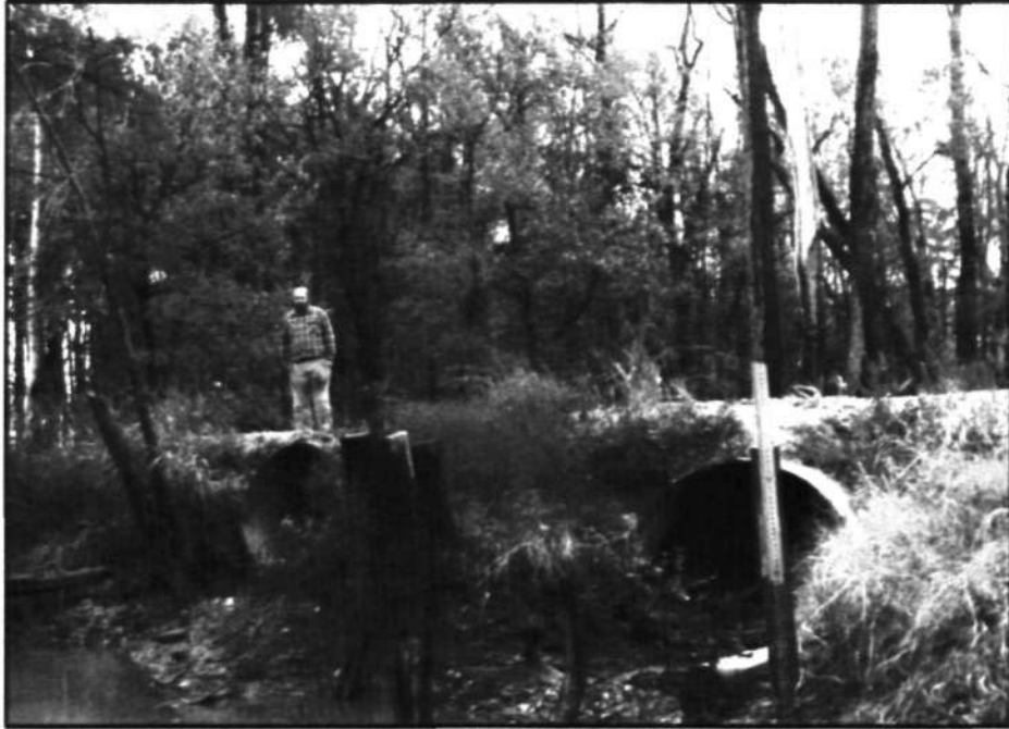
Figure 5. Lake Creek gravel road overpass fitted with two corrugated metal culverts
