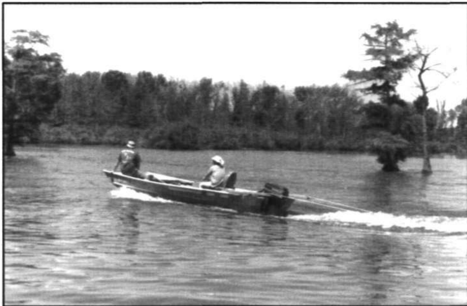
Figure 6. Sediment raking above the dam using log-chains pulled behind a power boat
