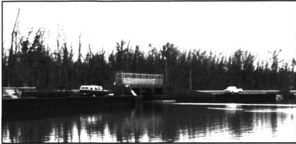
Figure 3. Panoramic view of upstream side of dam
