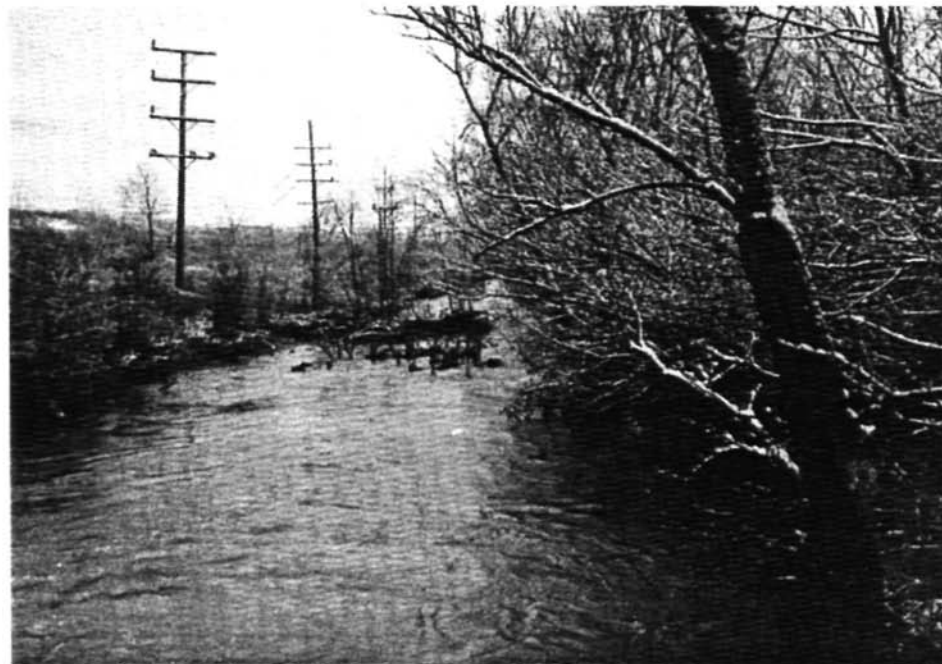
Figure 16d. The Illinois and Michigan Canal downstream of Lock 2 on January 5, 1993
