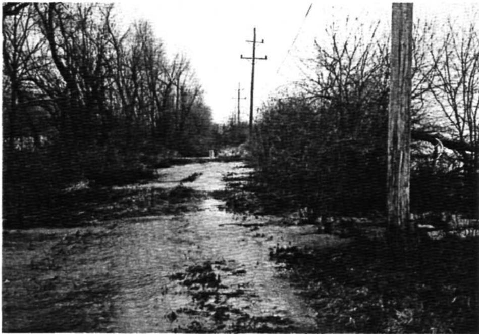
Figure 16f. The overland flow condition from the Illinois and Michigan Canal looking north from the Deep Run foot bridge on January 5, 1993
