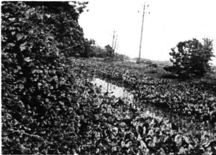
Looking Upstream from the Overflow Weir
