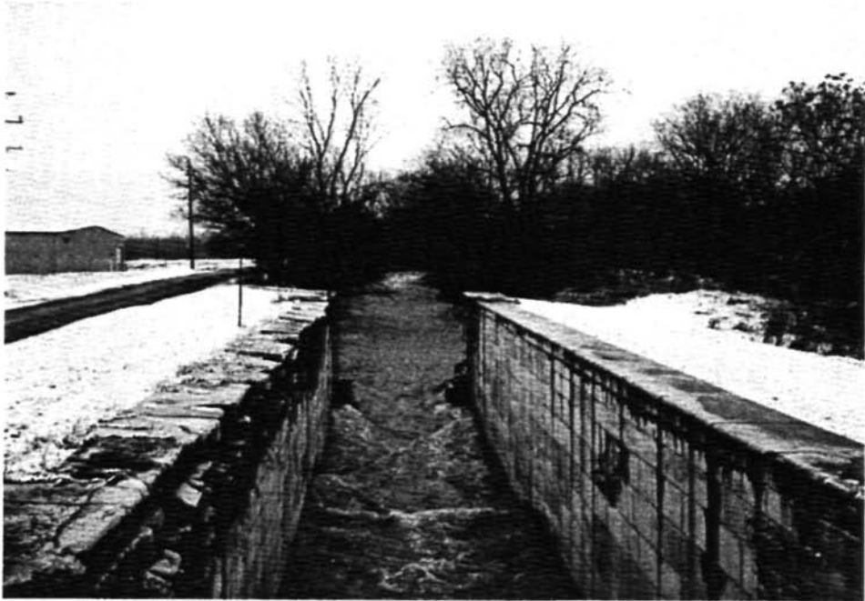
Figure 16a. The Illinois and Michigan Canal at Lock 1 on January 5, 1993
