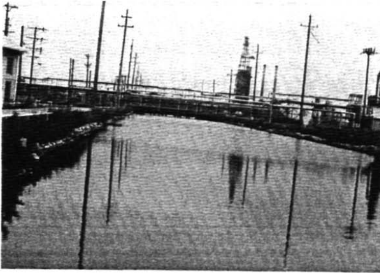
Looking Upstream from the Texaco Dam
