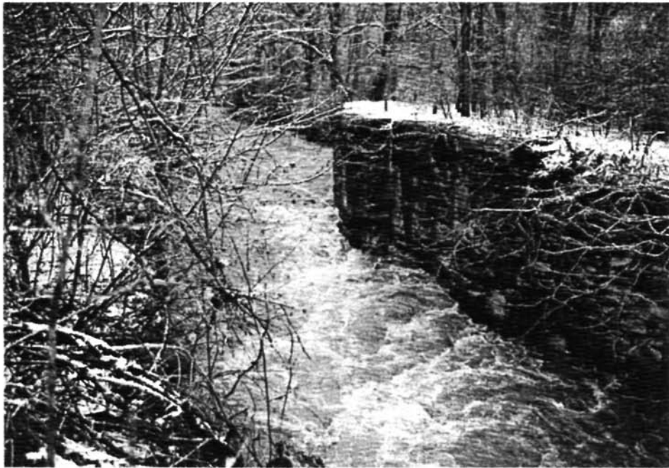
Figure 16b. The Illinois and Michigan Canal at Lock 2 on January 5, 1993
