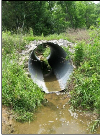
Figure 6.4 Impact Site #4: looking upstream at culvert.
