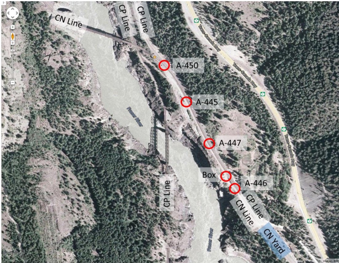
Figure 2-9 Google satellite image showing approximate location of four ties installed in track near Cisco Bridges, Lytton, BC.
