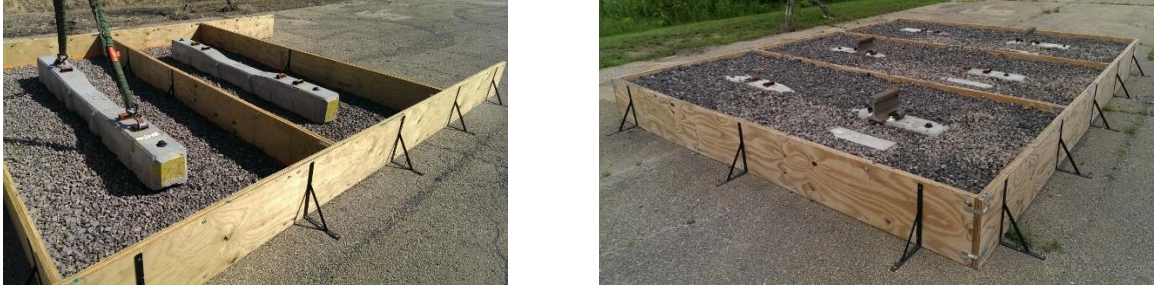
Figure 2-8 Construction of ballast box (left) and final configuration (right).
