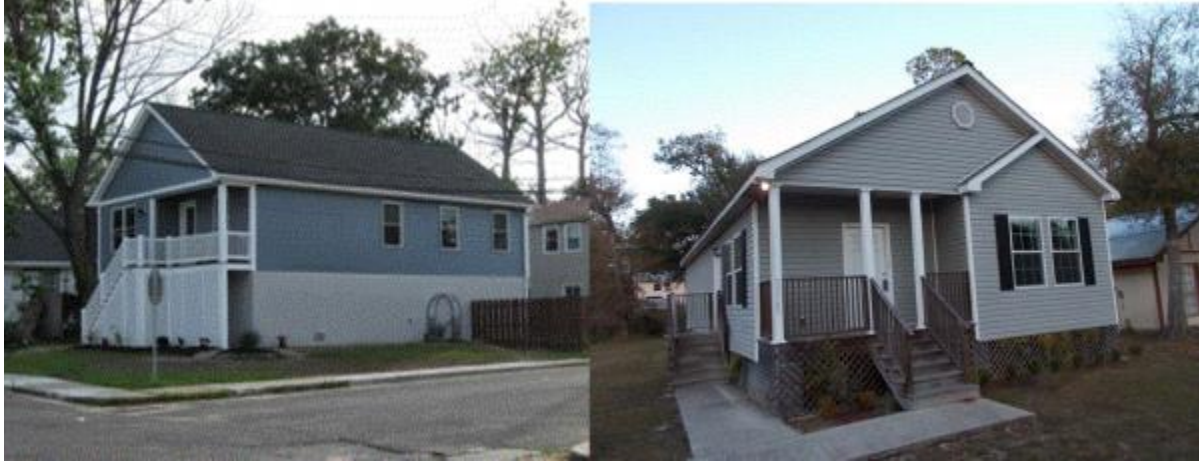
Figure 1 These homes have been elevated.
