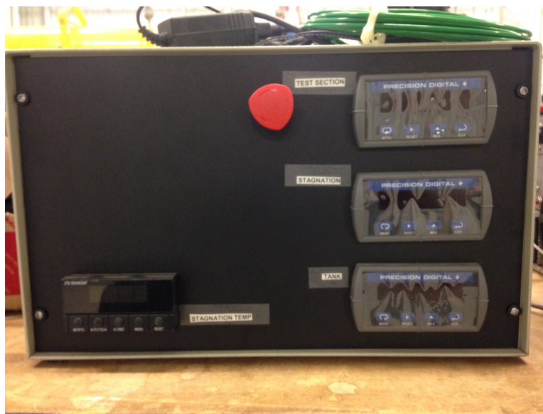
Figure 2.15: The wind tunnel control panel.
