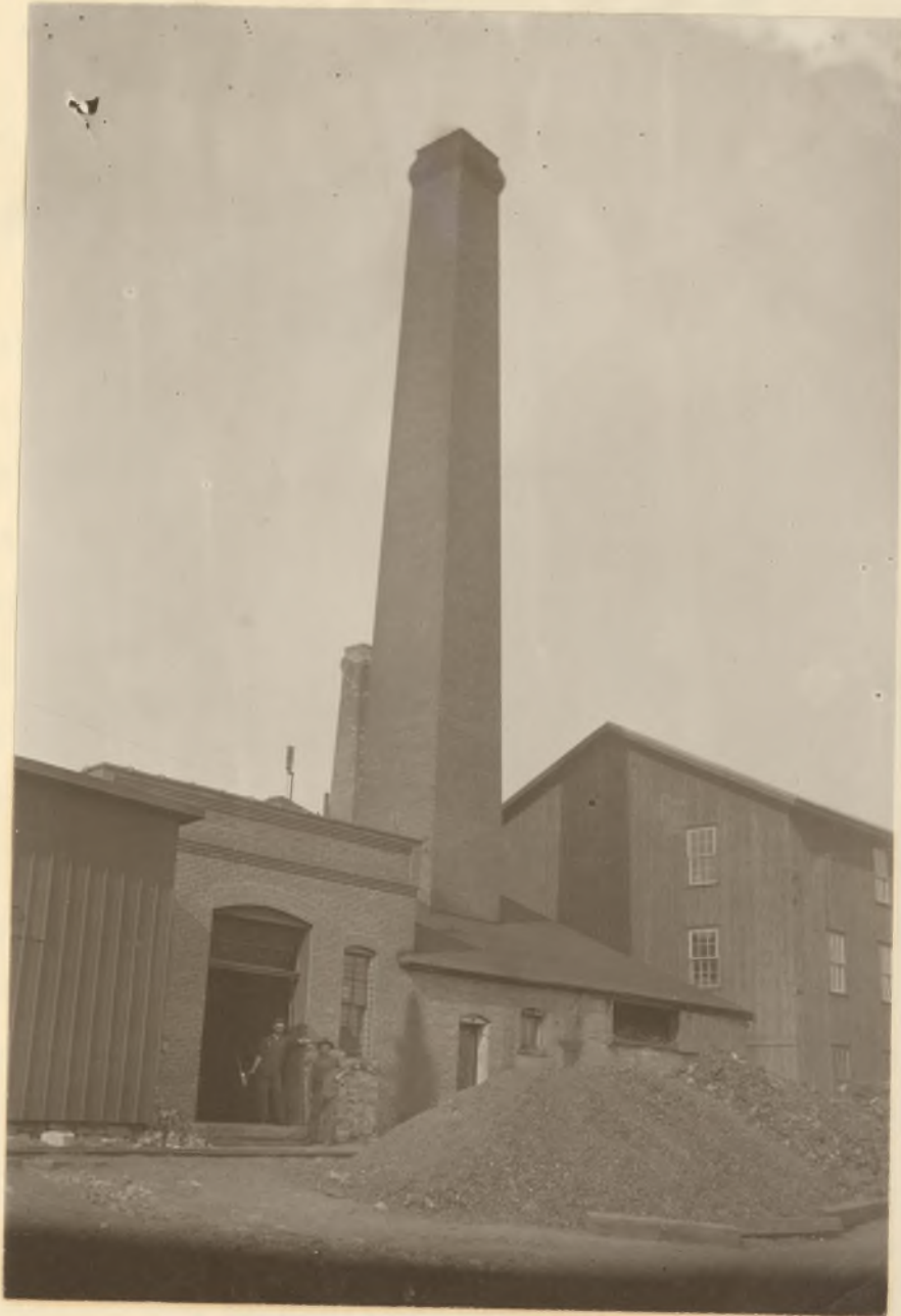
NAPERVILLE ILLINOIS ELECTRIC LIGHT PLANT.
