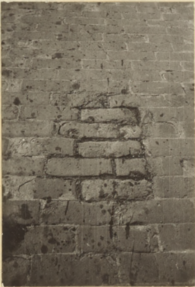
"POOR GROUTING"
