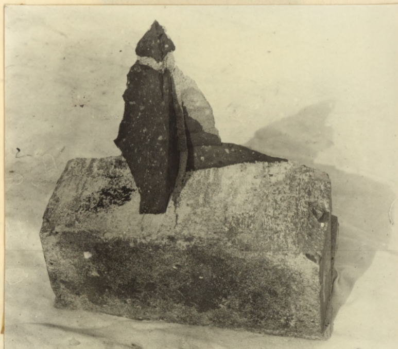
Shattered brick Showing strength of grout
