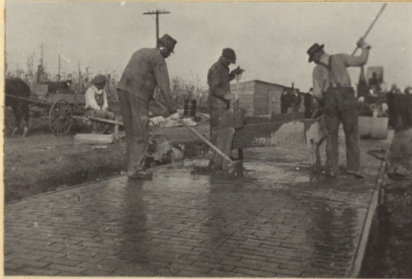
Wooden mixing box
