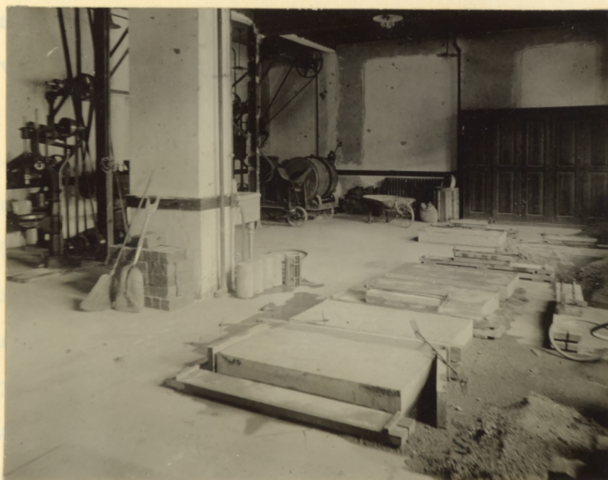
Forms removed preparatory to testing
