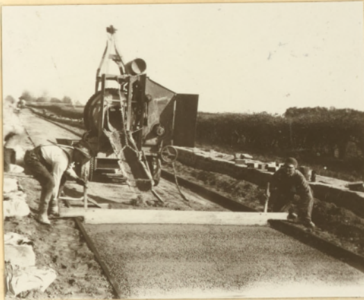
Striking off concrete
