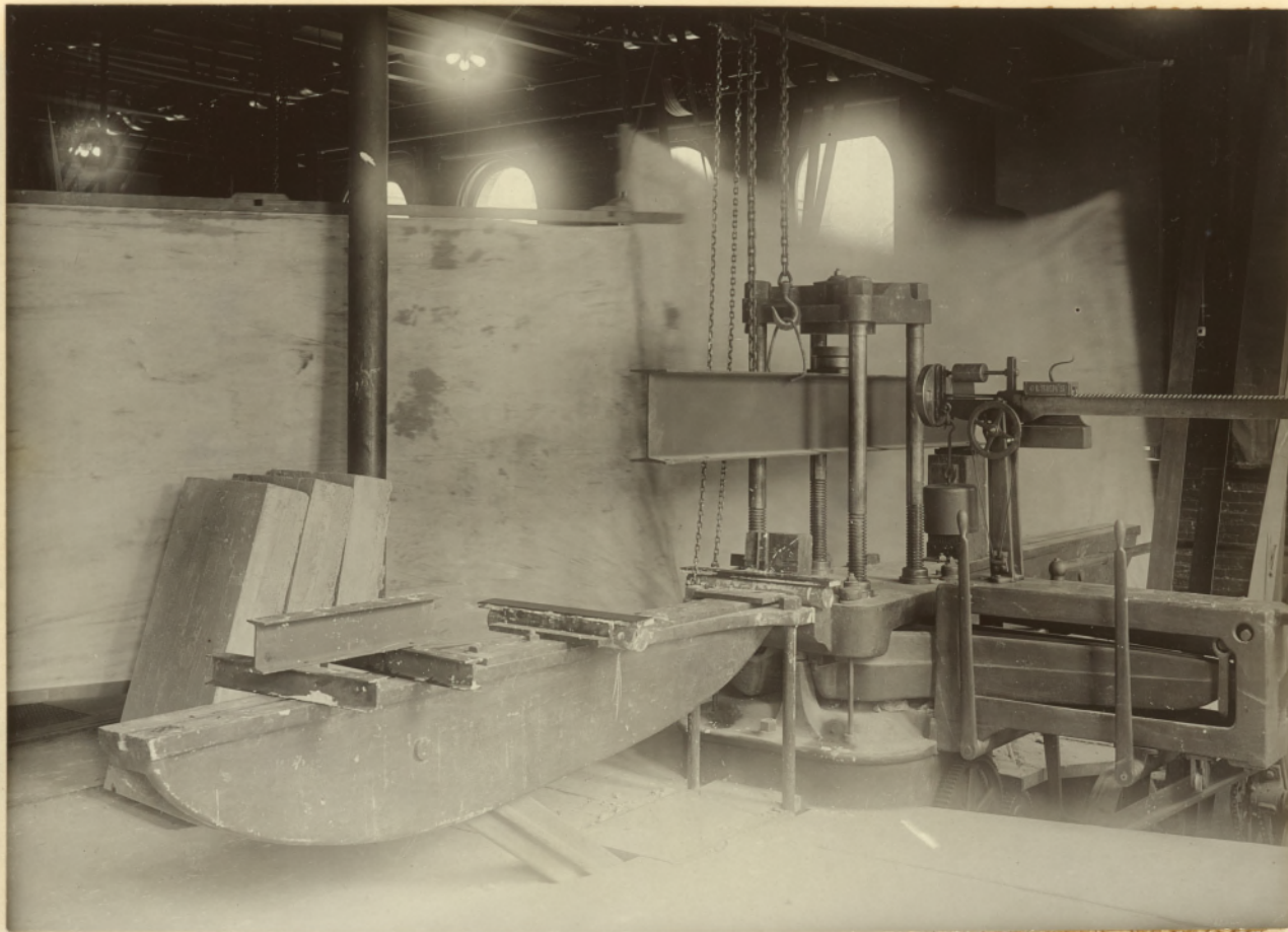
Equipment ready for Slab to be placed.
