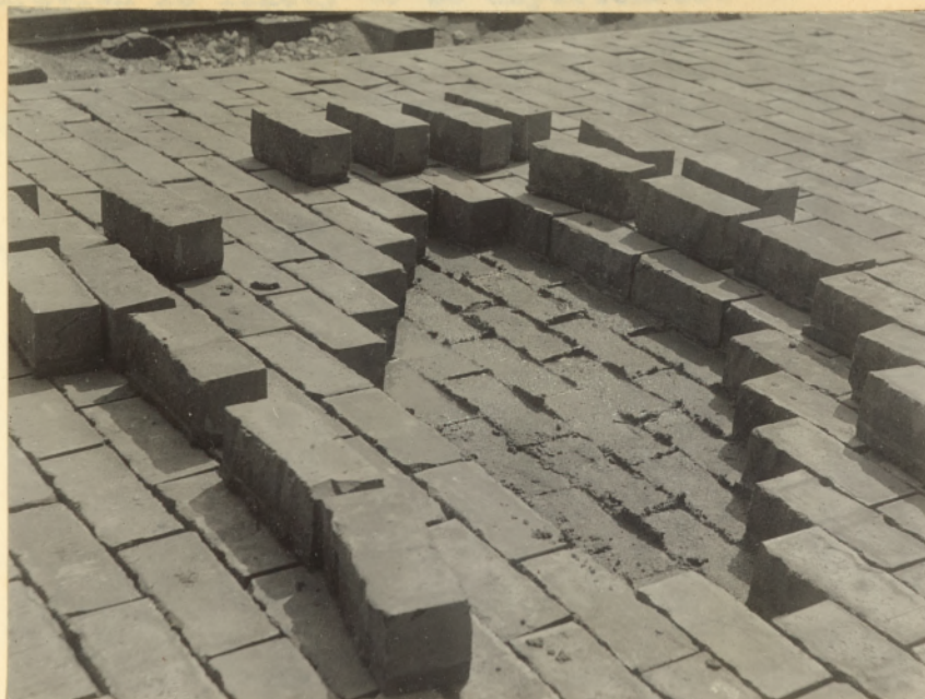
The brick are bedded in the green concrete
