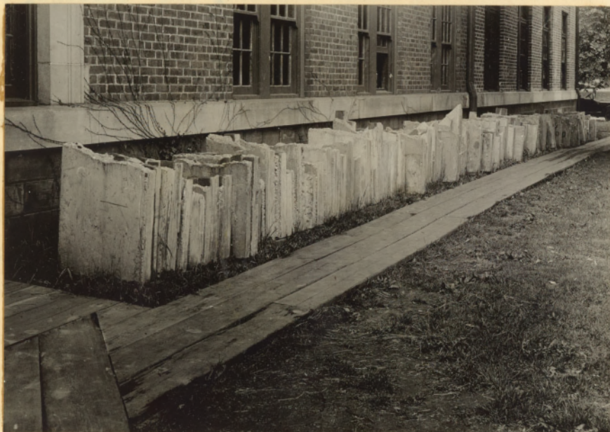
Storing slabs after breaking
