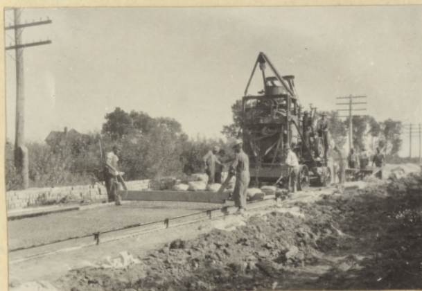
Placing and tamping concrete base
