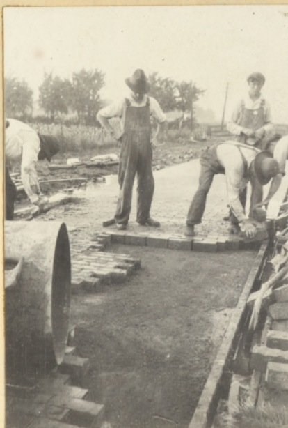
Reshaping concrete base
