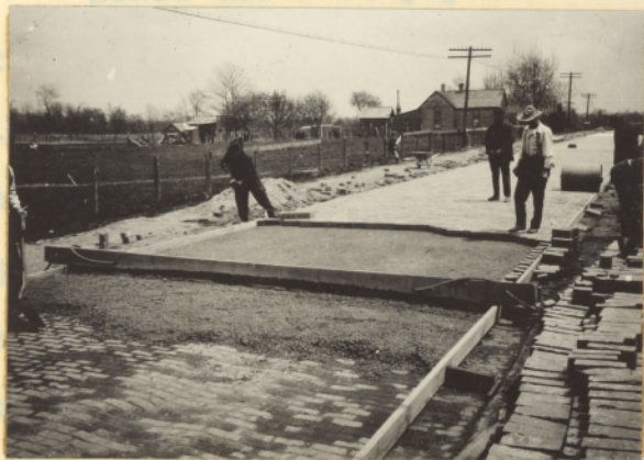
Re-surfacing old brick pavement
