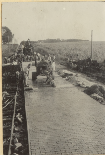
Use of mechanical mixer
