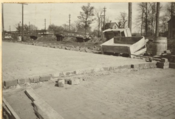
4-inch brick are laid on a smoothing layer of concrete
