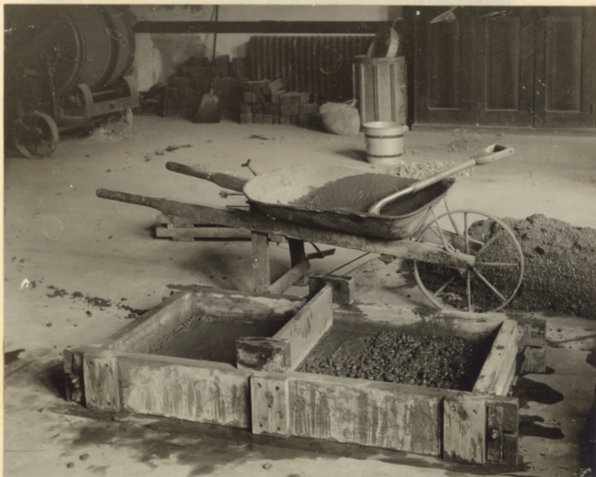
Striking off concrete
