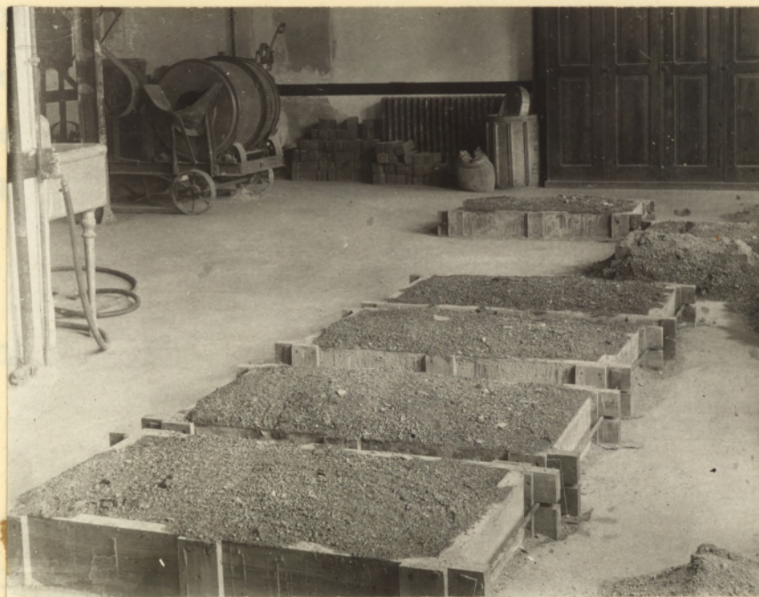
Curing the slabs
