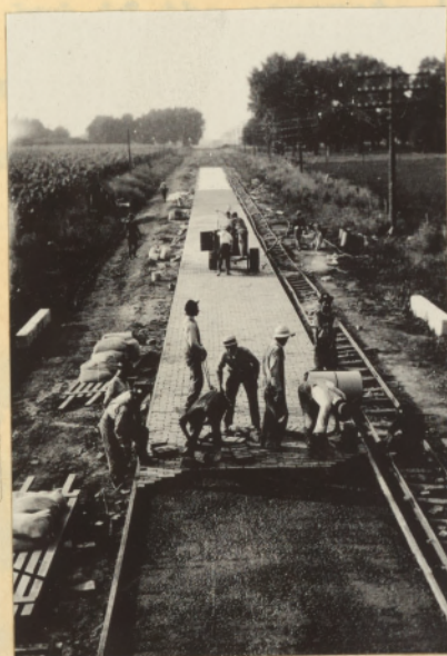
All operations are carried on within 100 feet of the mixer
