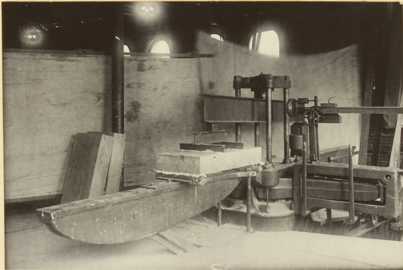
Slab ready for Load to be applied
