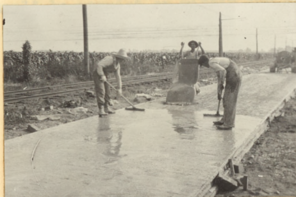
Second application of grout
