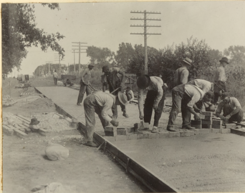
Laying brick on tamped surface
