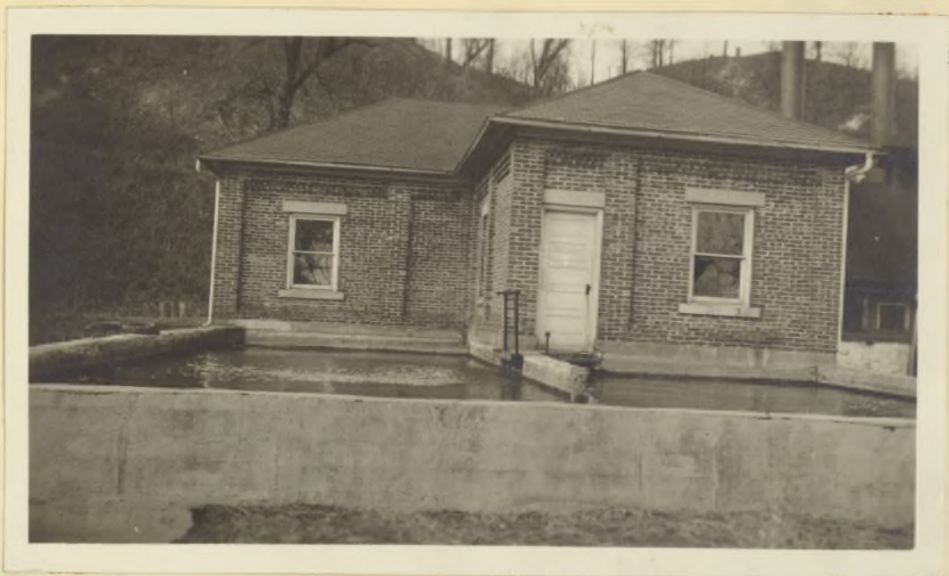
View showing sedimentation basin and filter house
