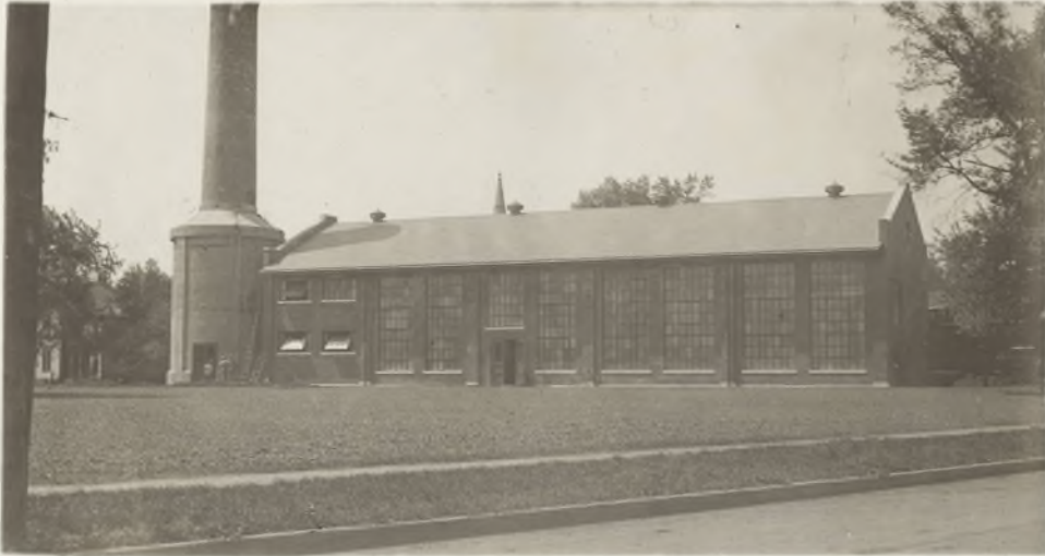
Fig. 30. Exterior View of The Illinois Plant.
