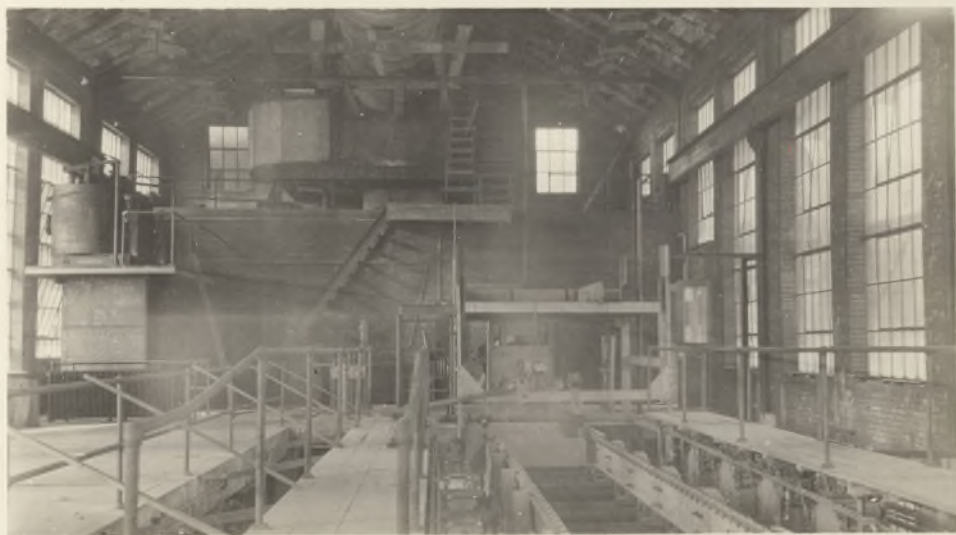
Fig. 23. Interior View of Plant, arranged to test a Consolidation Locomotive.
