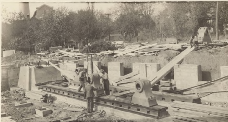
Fig. 15. Foundation for the Supporting Mechanism and Dynamometer Pier, Illinois Plant.
