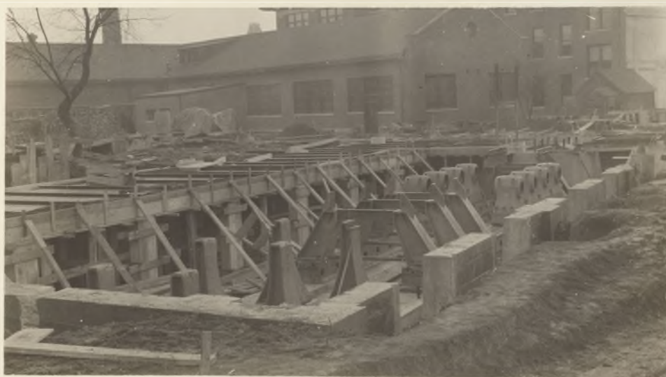
Fig. 16. Completed Foundations for Supporting Mechanism and Dynamometer, Illinois Plant.
