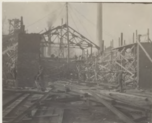
Fig. 20, Illinois Plant in Process of Construction.
