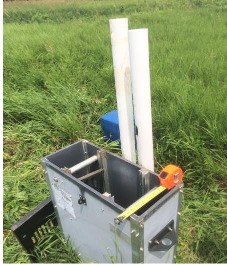
Figure 4.2: Drainage Control Structure
