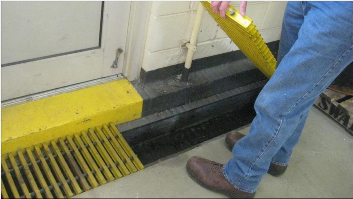
Figure 23. Drainage trench along interior perimeter of storage areas at SWALCO facility.
