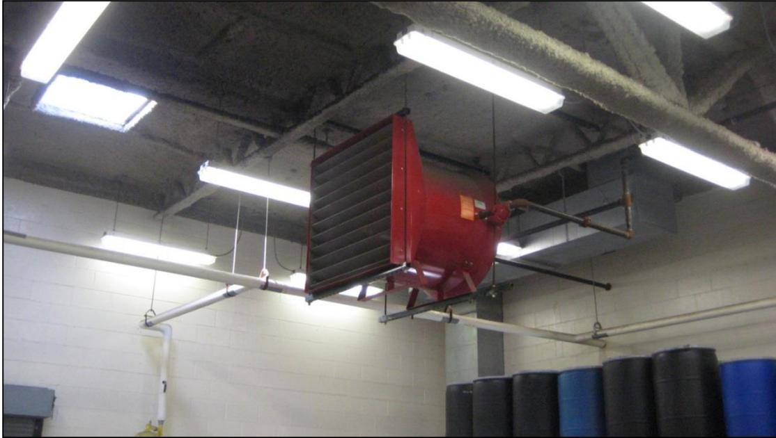
Figure 24. High-expansion foam fire suppression system over interior storage areas.
