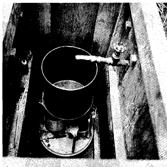
Fig. 21. A recording rain gauge measured the subsurface flow.
